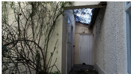
Figure 7: covered passageway at rear
