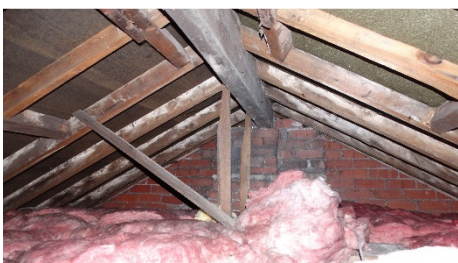
Figure 9: roof void over rear extension
