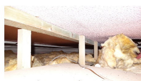
Figure 10: suspended ceiling on extension
