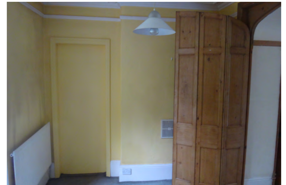
Existing infilled opening in rear Dining Room
