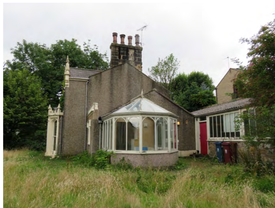
North end elevation, showing conservatory and garden room against West boundary wall.
