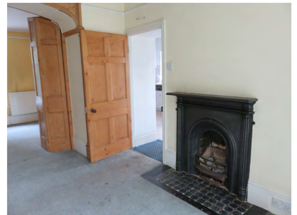
Existing front Dining Room.
