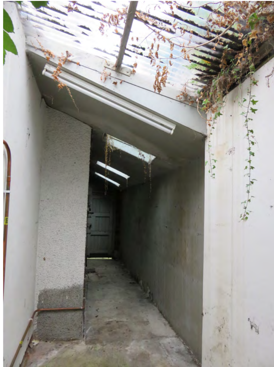
Covered storage area against South gable end of house.
