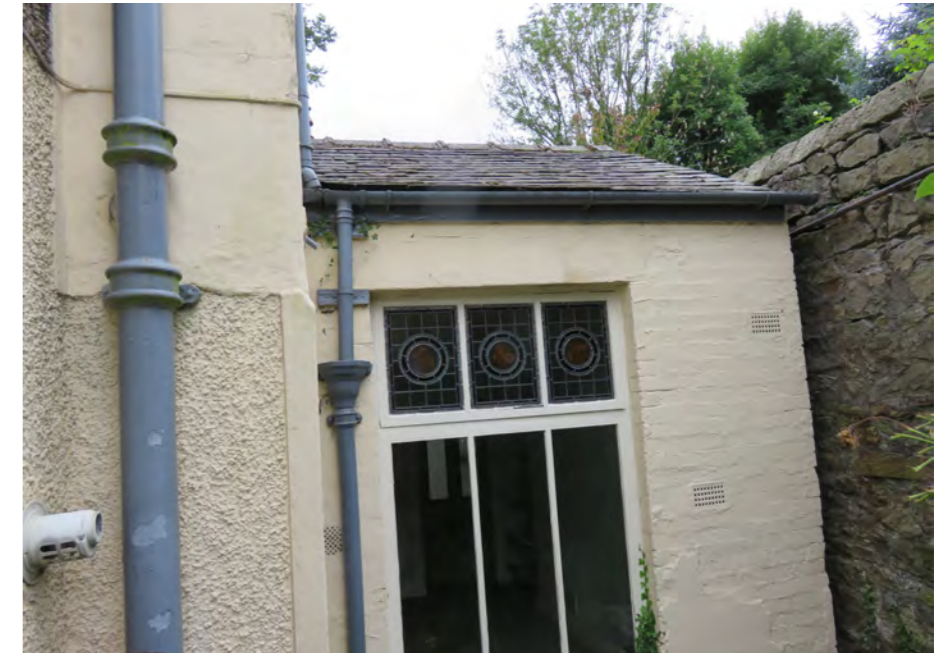
Rear courtyard area looking towards Sitting Room extension.
