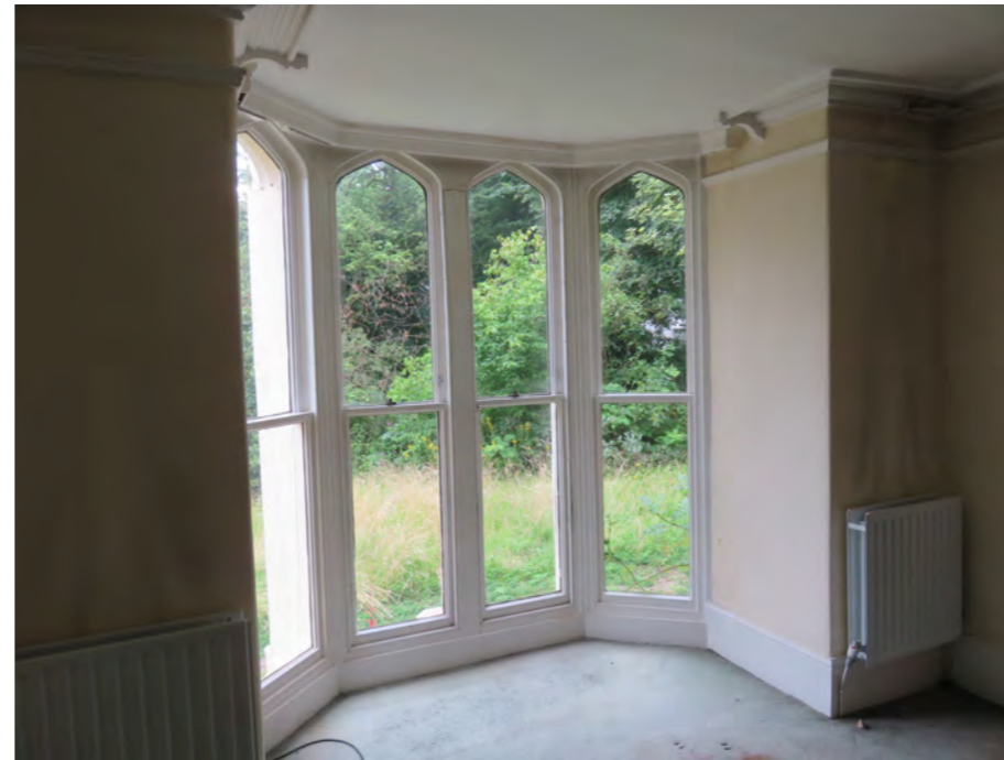
Existing full height front bay window.
