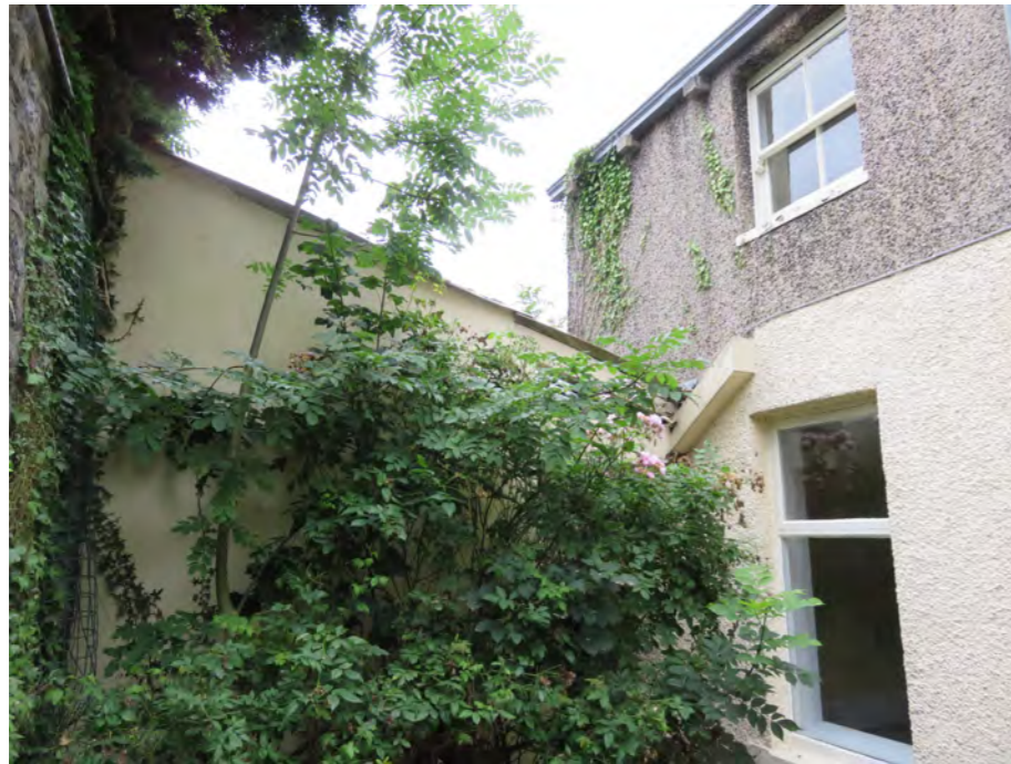
Rear enclosed courtyard area, towards current lean-to outbuildings.
