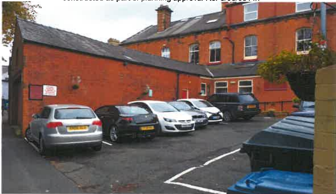
Photograph 4 West Elevation of the outbuilding, part north elevation of the main building and rear yard
