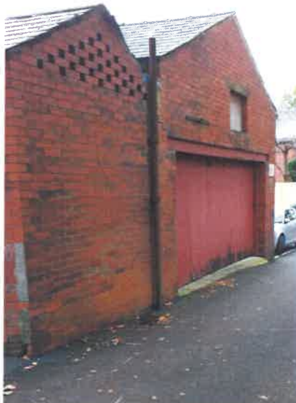
Photograph 6 North Elevation of the outbuilding. It is proposed to retain the main feature opening.
