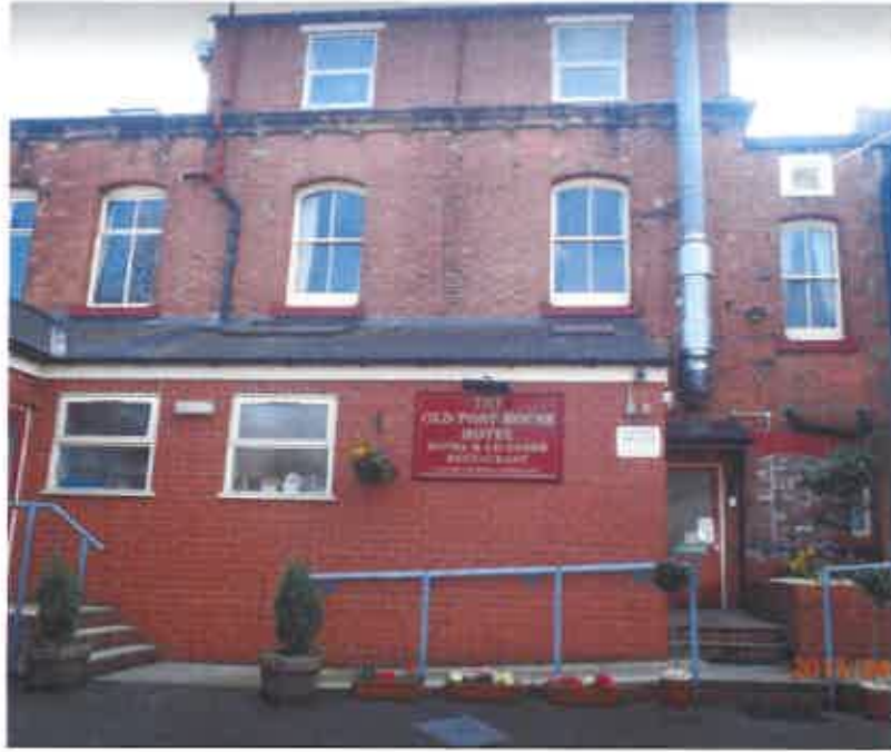
Photograph 3 Rear Elevation (North): The single storey lean-to was constructed as part of planning approval Ref 3/03/0511/P
