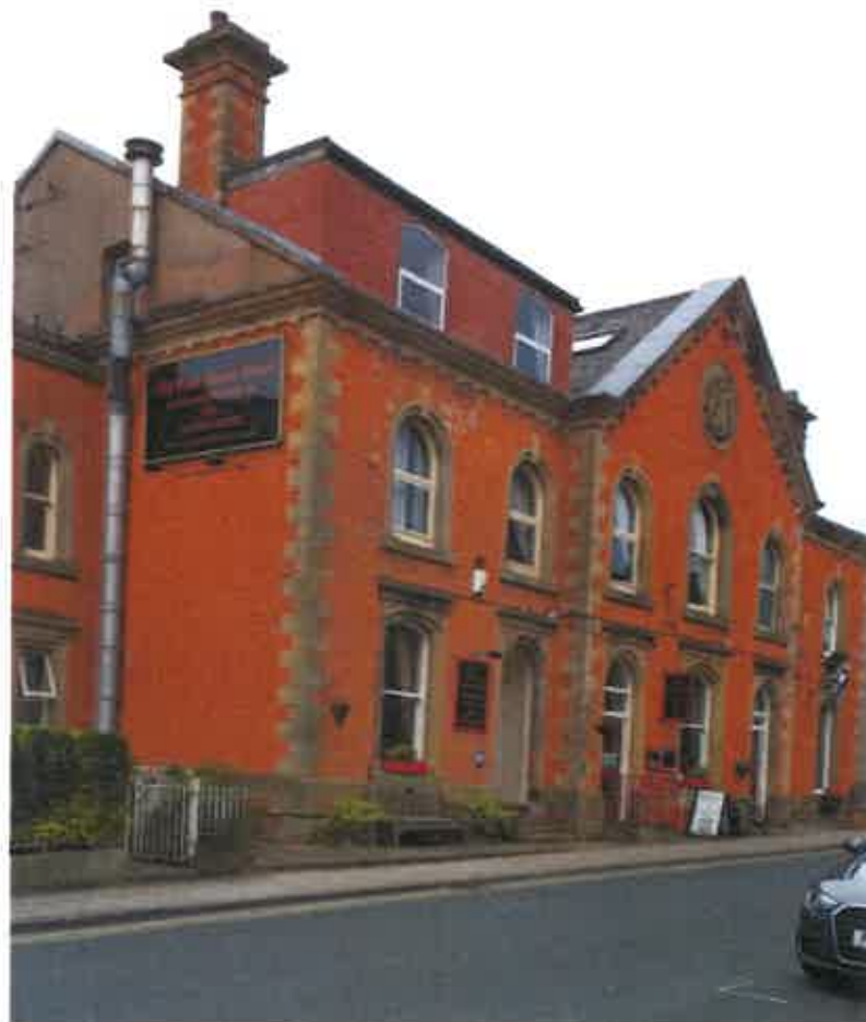
Photograph 2 Pinciple King Street Elevation (south): Roof dormer and s/s flue are the latter day additions.
