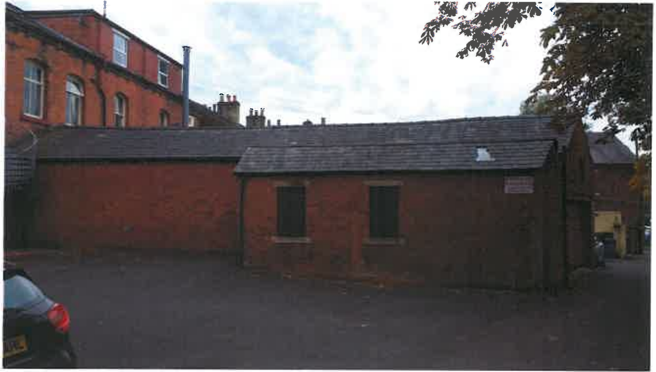
Photograph 5 East Elevation of the outbuilding and part north (rear) elevation of the main building
