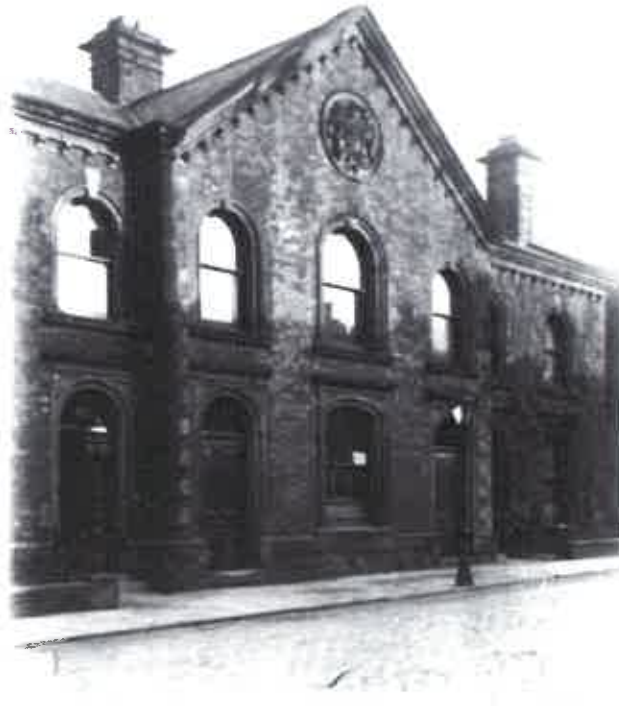
Photograph 1 Pinciple King Street Elevation (south): As Constructed
