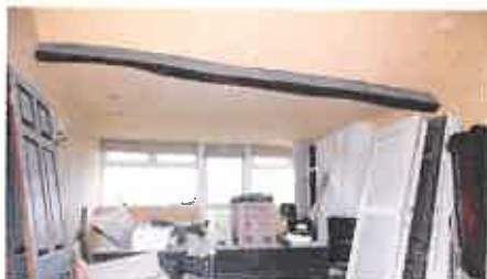
Figure 5: internal first floor room at rear
