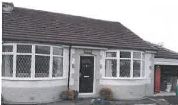
Front elevation to Whalley road
