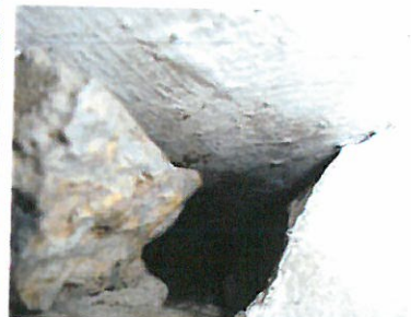
Void at abutment with wall and soffit
