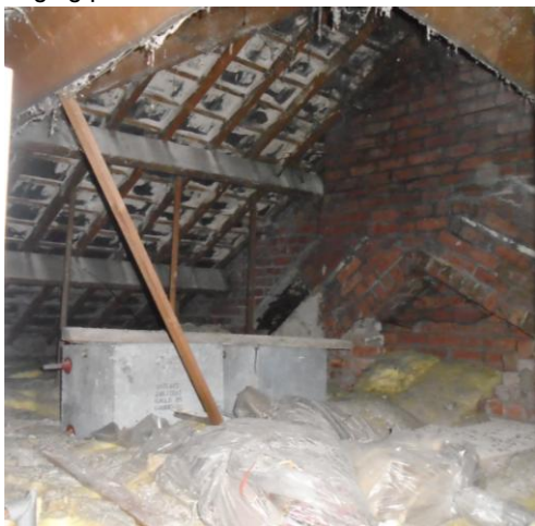
Main roof void
