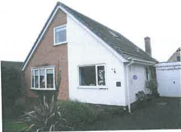
NE Front elevation from road.
