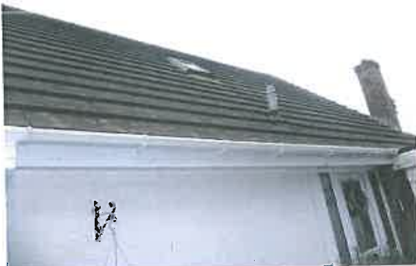
NW side elevation, concrete tiles are tight fitting with no gaps.
