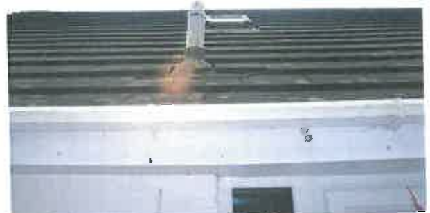
NW side elevation, concrete tiles are tight fitting with no gaps.
