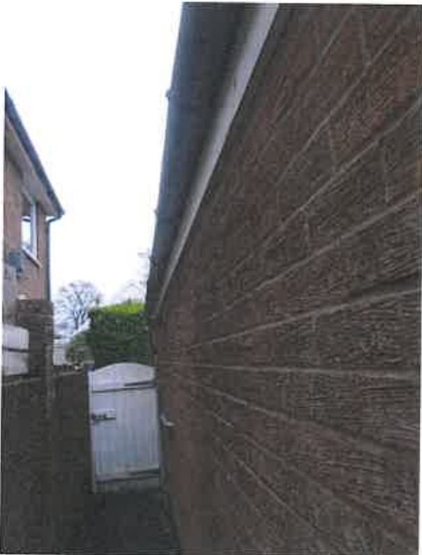
NW side elevation of garage with tight fitting fascia boards.
