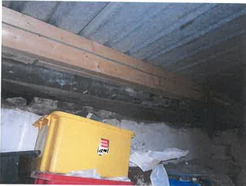
Photograph 9: Interior of west elevation. Roof felt and lead flashing is associated with the adjoining outbuildings.
