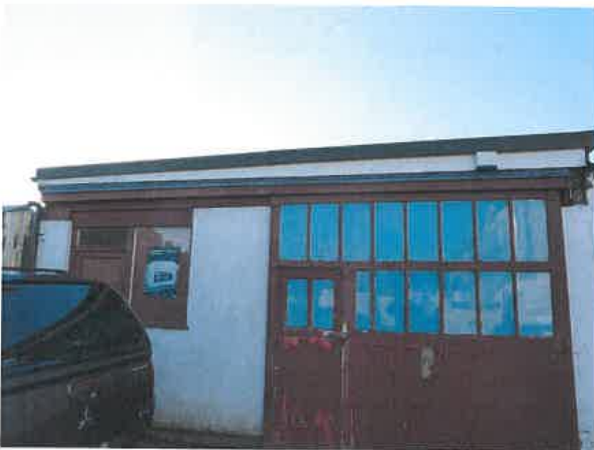
Photograph 1: Typical view of the front (north elevation) of the building.
