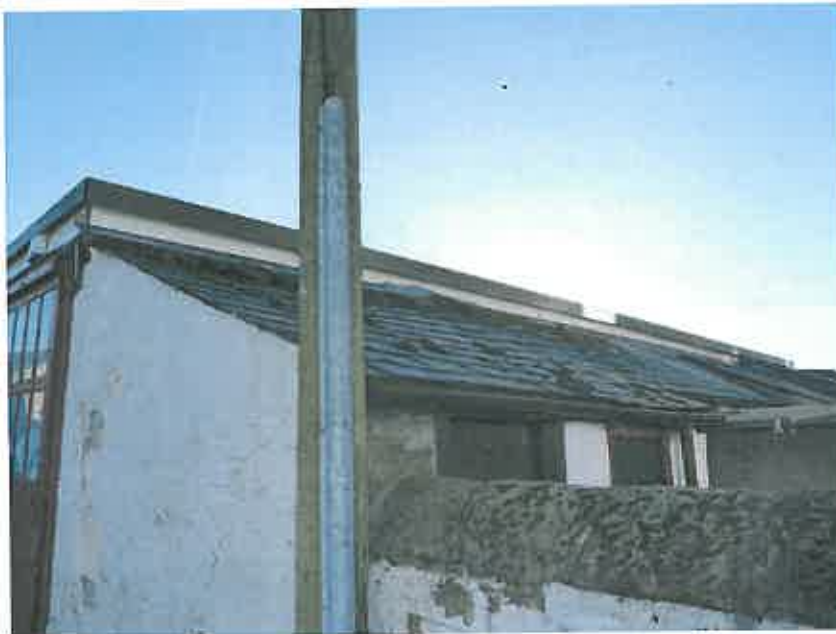
Photograph 3: The west elevation of the building abutting domestic outhouses (unaffected).
