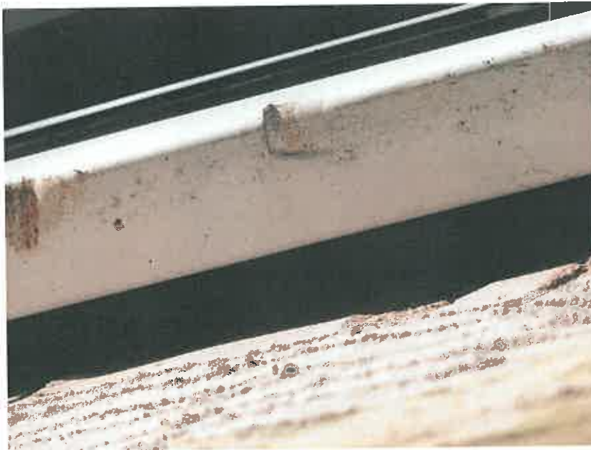
Photograph 7: Close-up of gap between UPVC fascia and wall. No viable void space for roosting bats present.
