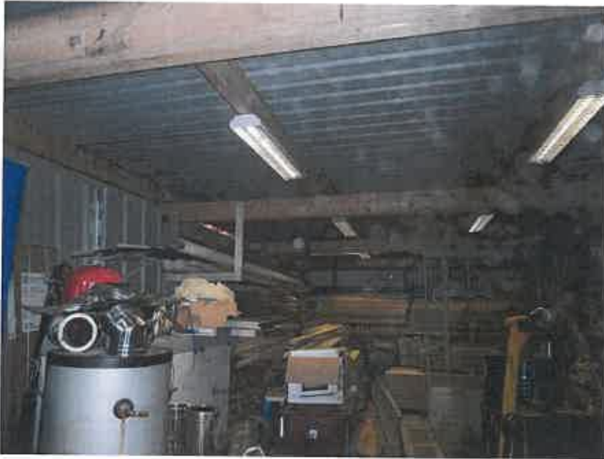
Photograph 4: General interior view showing simple construction and lack of loft/ceiling void space.
