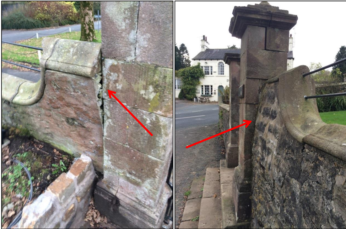
PL13: (Left) and PL14: (Right) discernable lean noted to east section of boundary wall.
