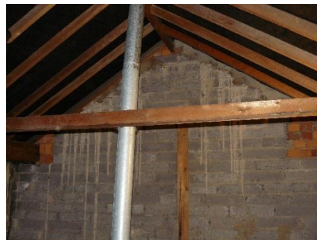
Figure 8: Loft space showing breeze block wall
