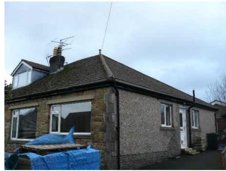
Figure 2: Western and southern elevation
