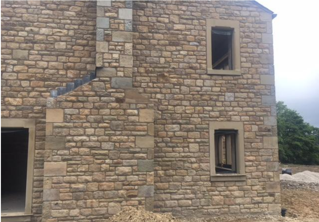
natural stone random stone walling brought to course with natural stone quoins ashlar stone stop chamfered window surrounds and cills
