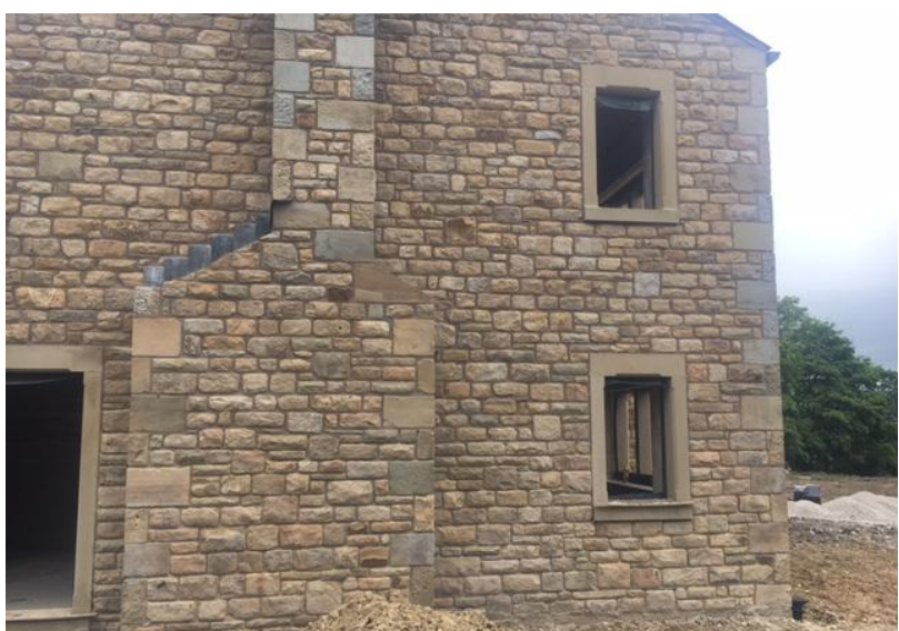
stone walling and stone window surrounds
