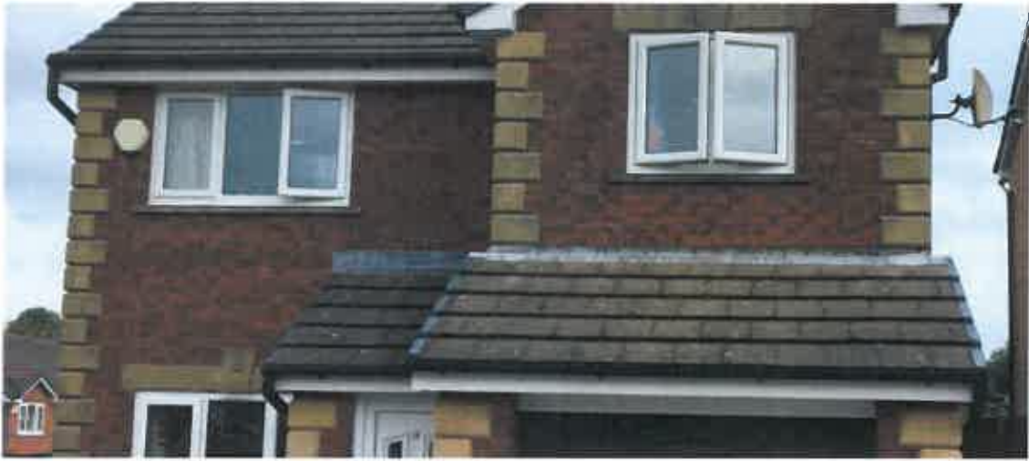
PL03: Existing rainwater goods to the dwelling.
