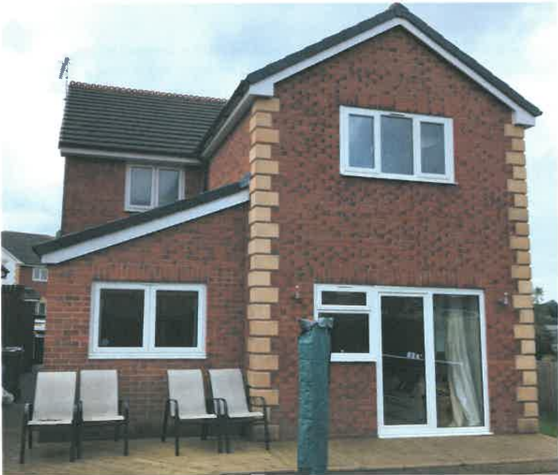
PL02: Existing walling materials to the dwelling.
