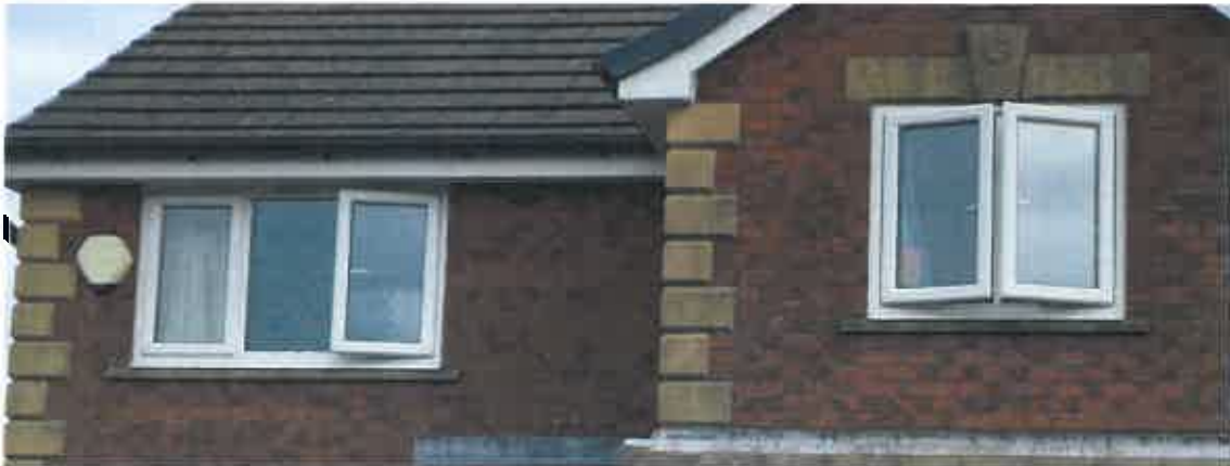
PL04: Existing uPVC double glazed windows to the dwelling.
