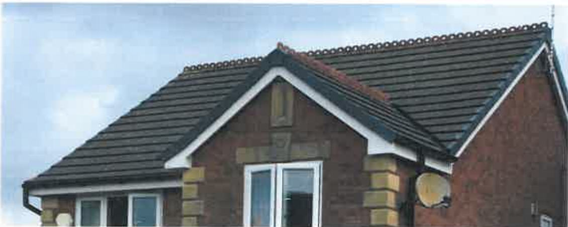
PL01: Existing roof covering to the dwelling.
