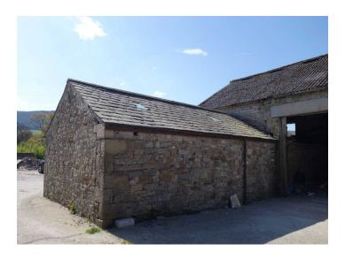
The outbuilding is a single storey stone built construction with double pitched stone slate roof. Roofing slates are in good condition.
