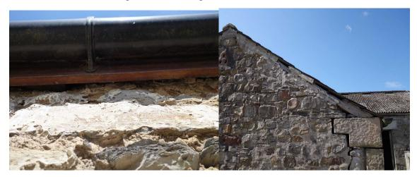
Gaps are present behind barge boards and cracks and crevices are present on external walls.
