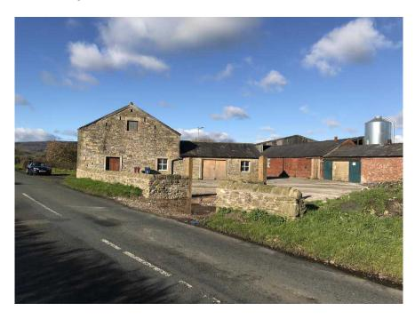
The property is a stone built semi detached barn with a double pitched fibreboard/asbestos roof. Pointing has some cracks or crevices present.
