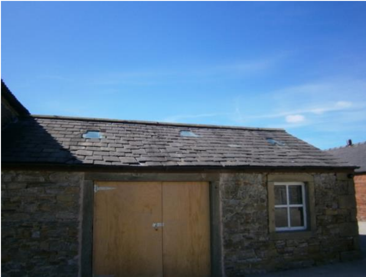
Photo 18 – Roof single storey
