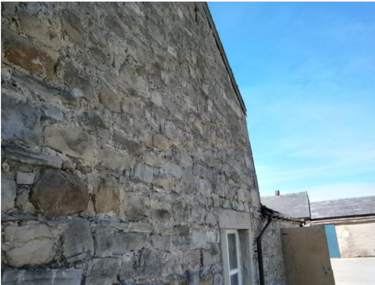
Photo 5 – Side elevation – bow to rear section
