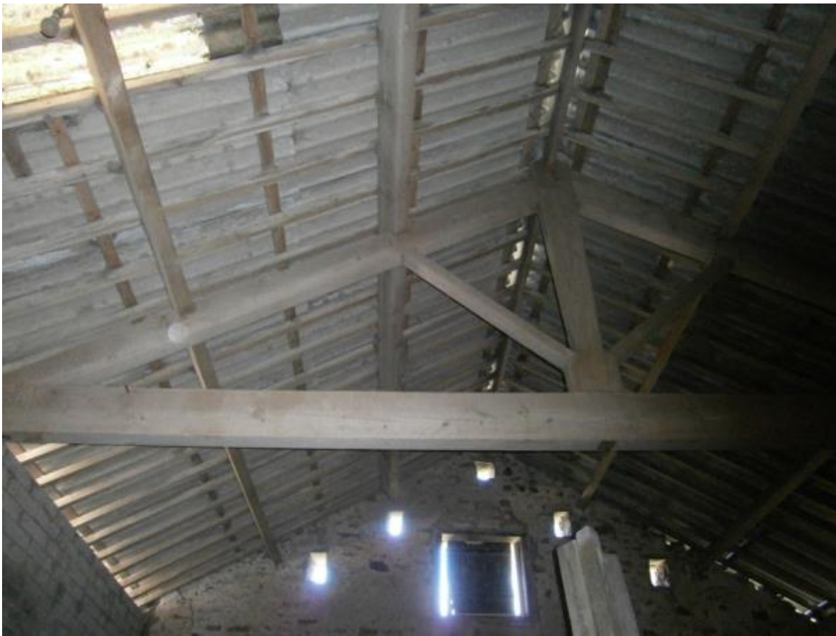
Photo 11 – Main barn roof truss
