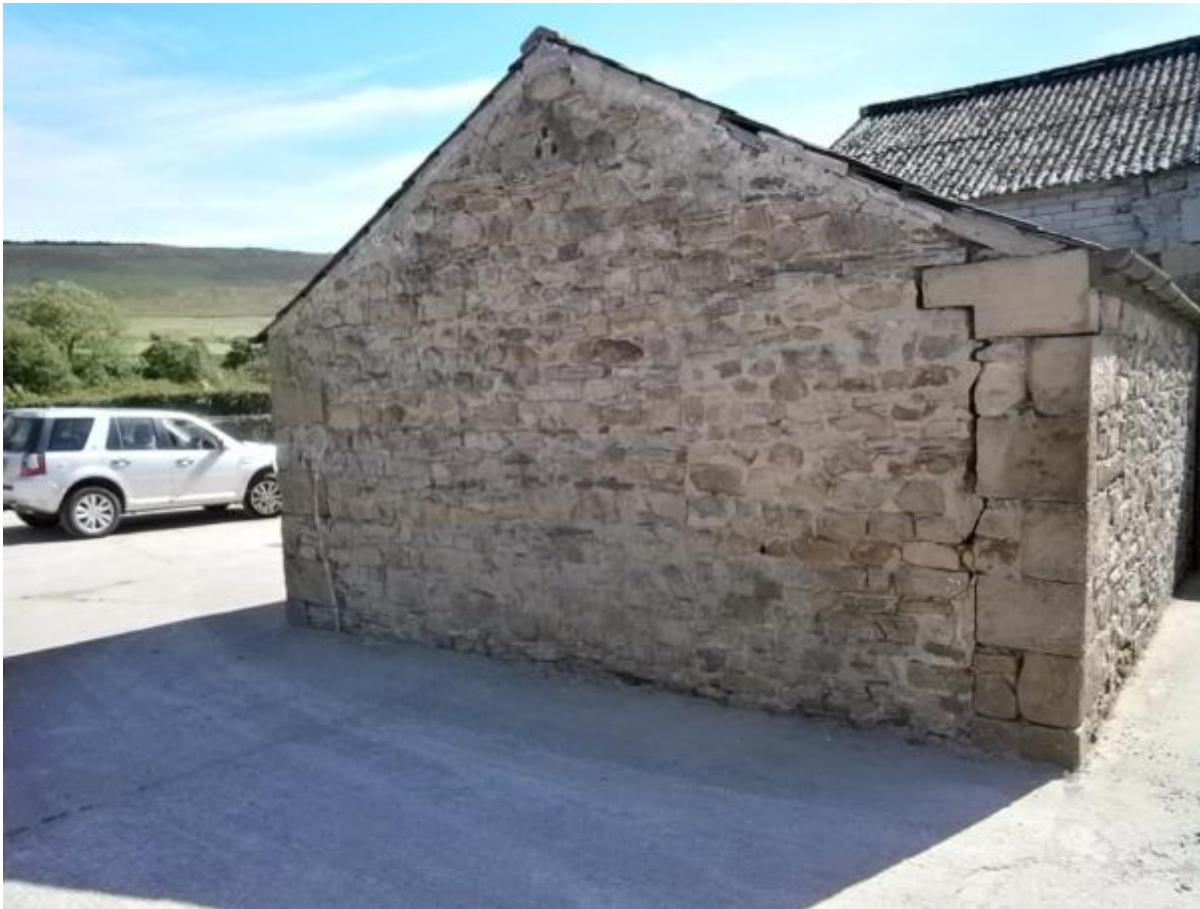
Photo 6 – Rear elevation of single storey
