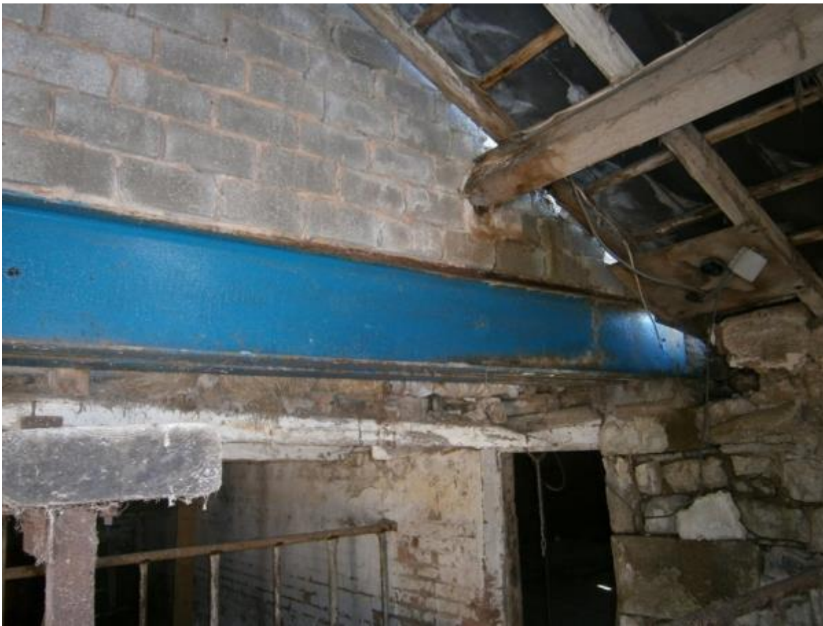
Photo 17 – Double steel beam to rebuilt rear elevation of main barn
