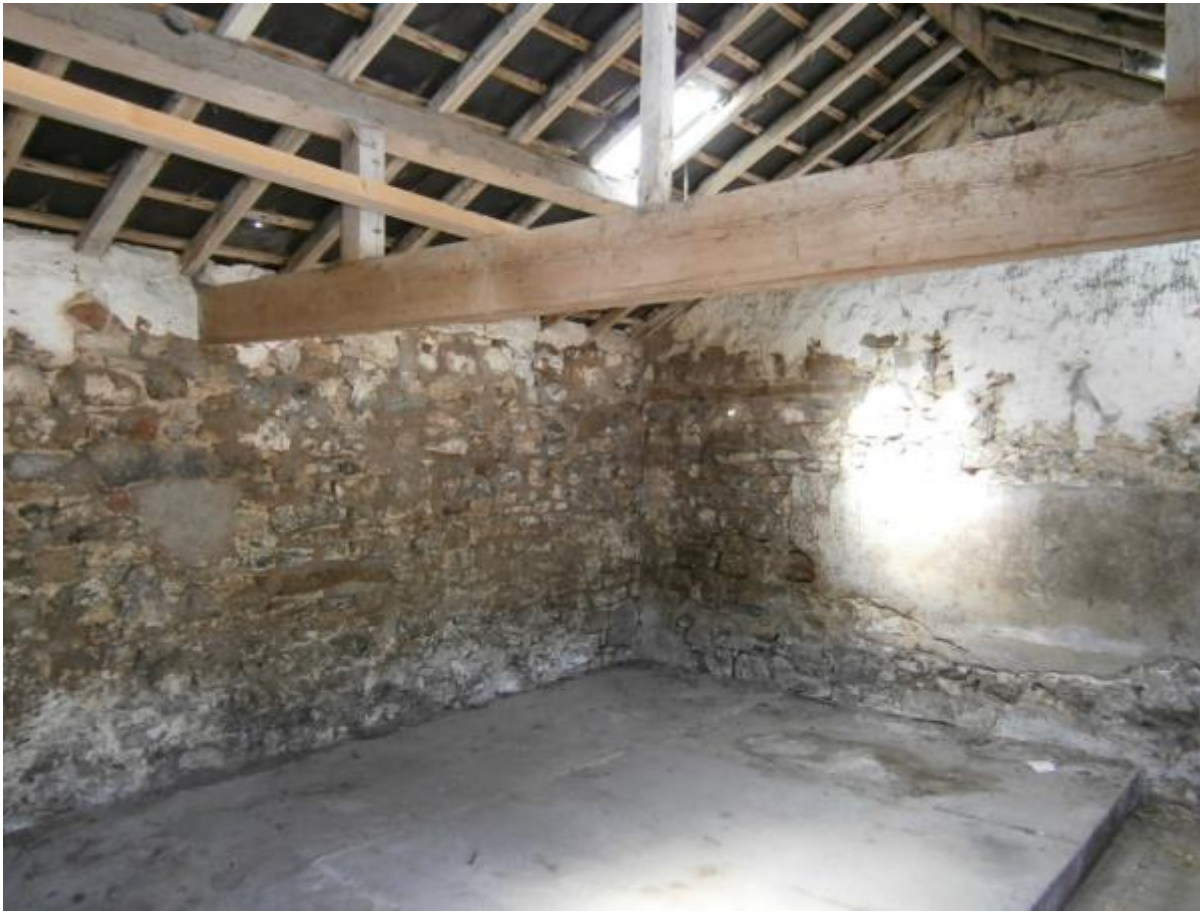
Photo 14 - Single storey internal
