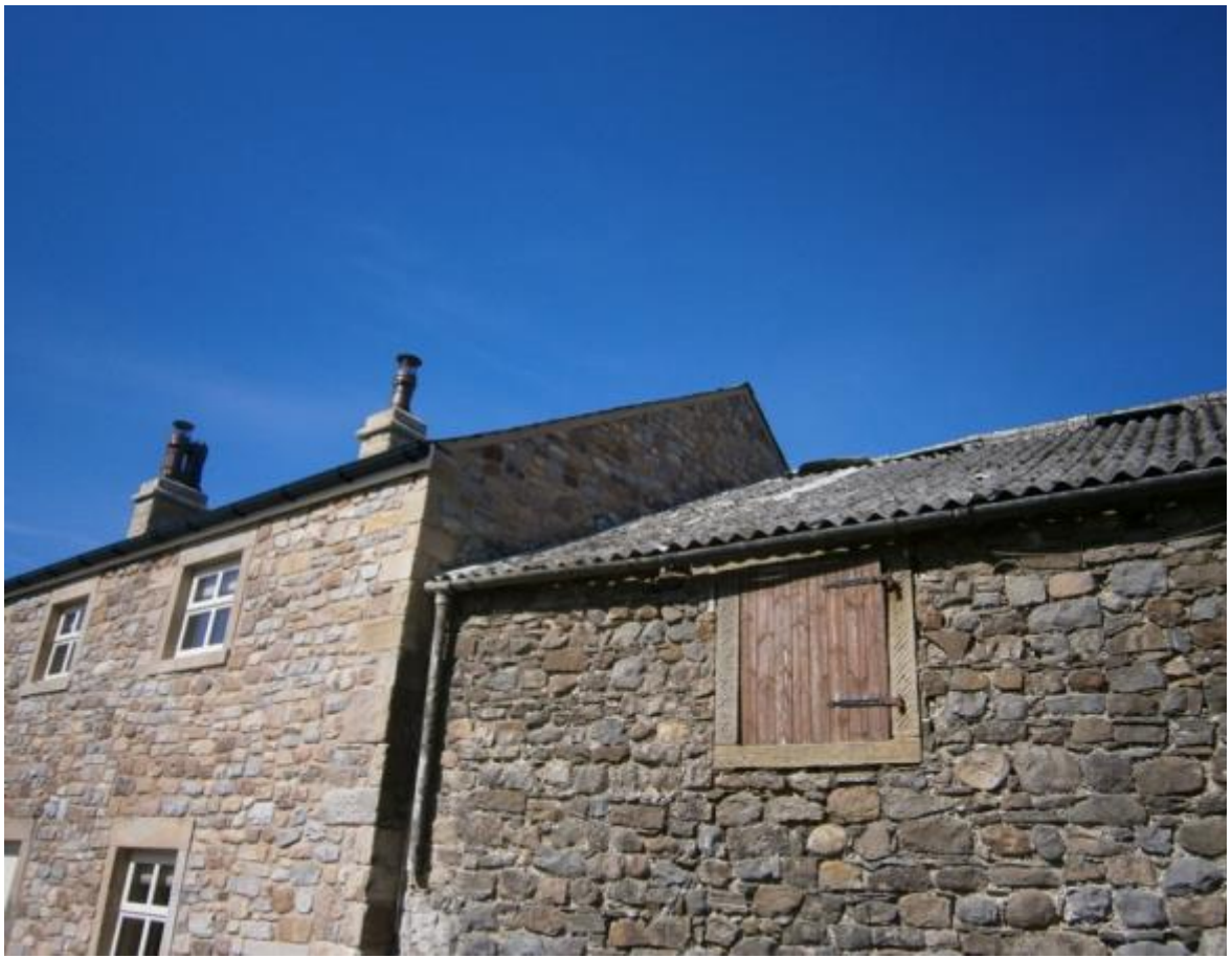
Photo 19 – Roof and junction with house – front elevation
