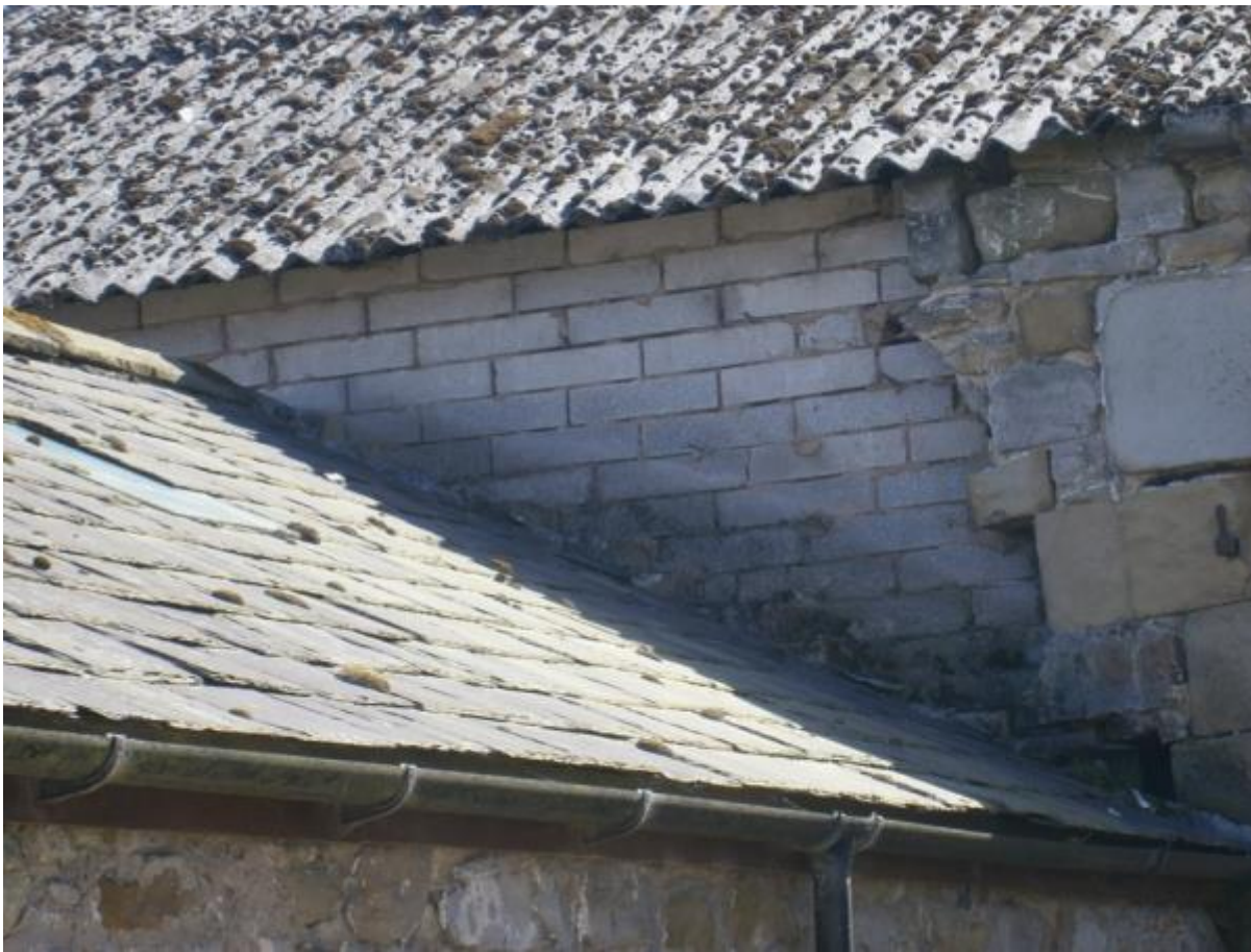
Photo 7 – Rear elevation block re-build
