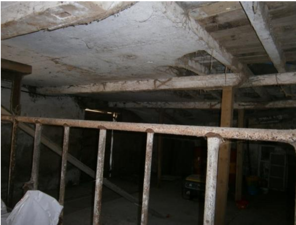
Photo 13 – main barn below below mezzanine
