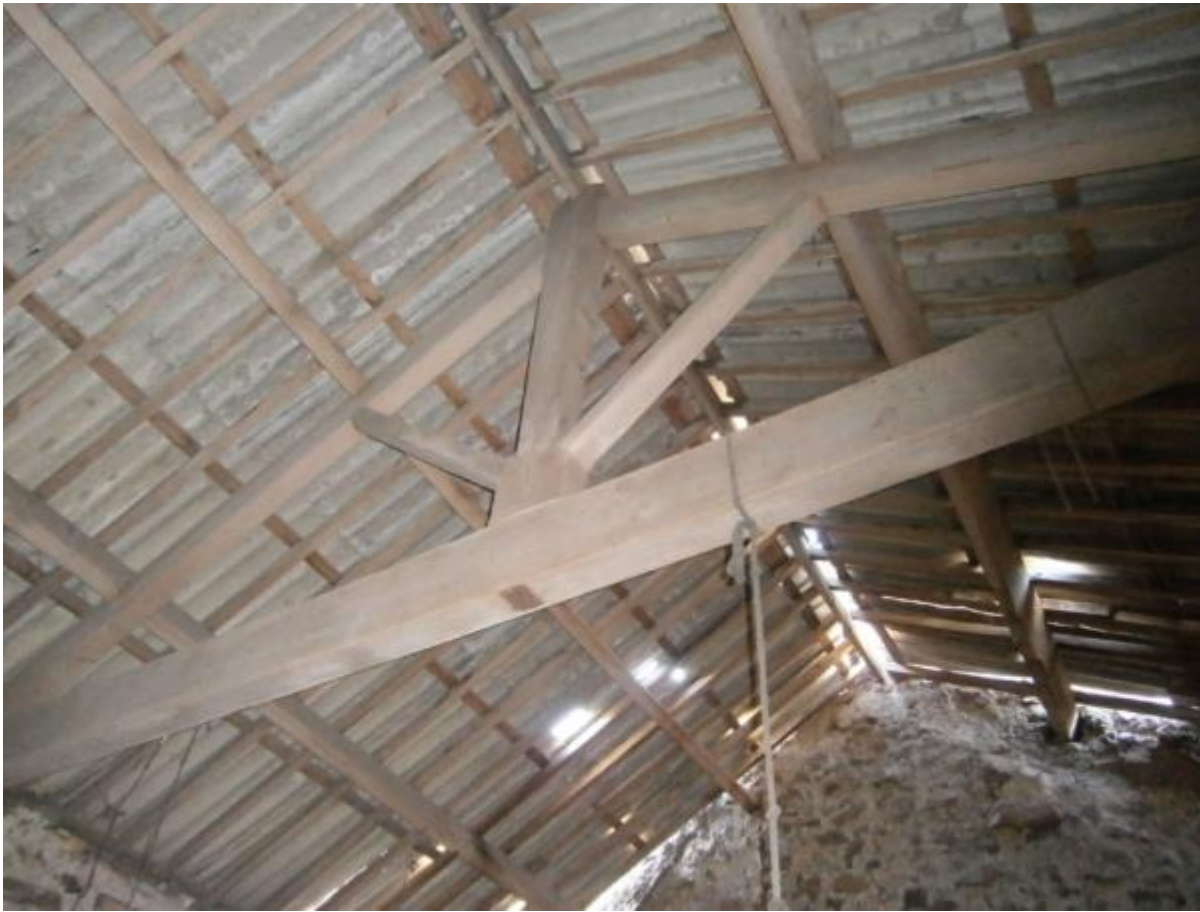
Photo 12 – Main barn roof truss, purlins and rafters
