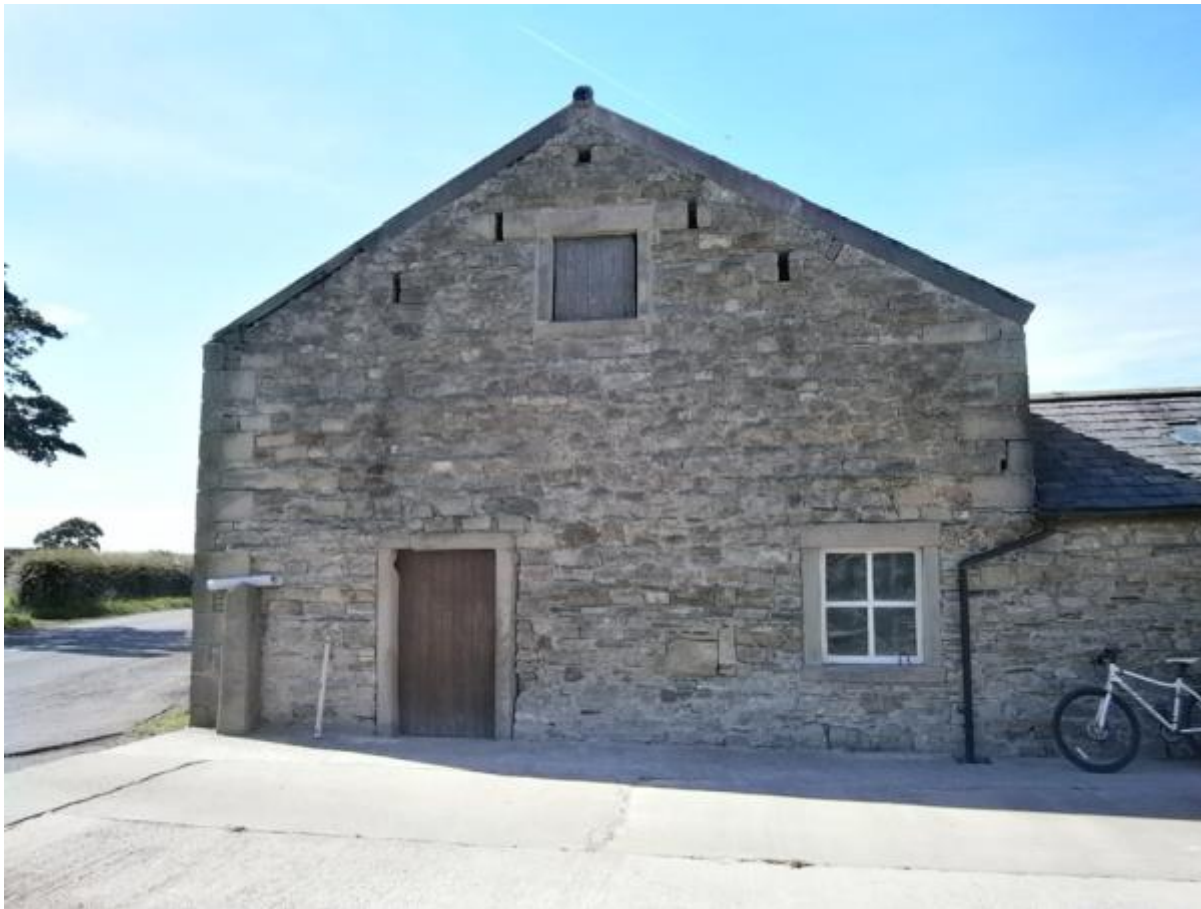
Photo 2 – Side elevation – Main Barn
