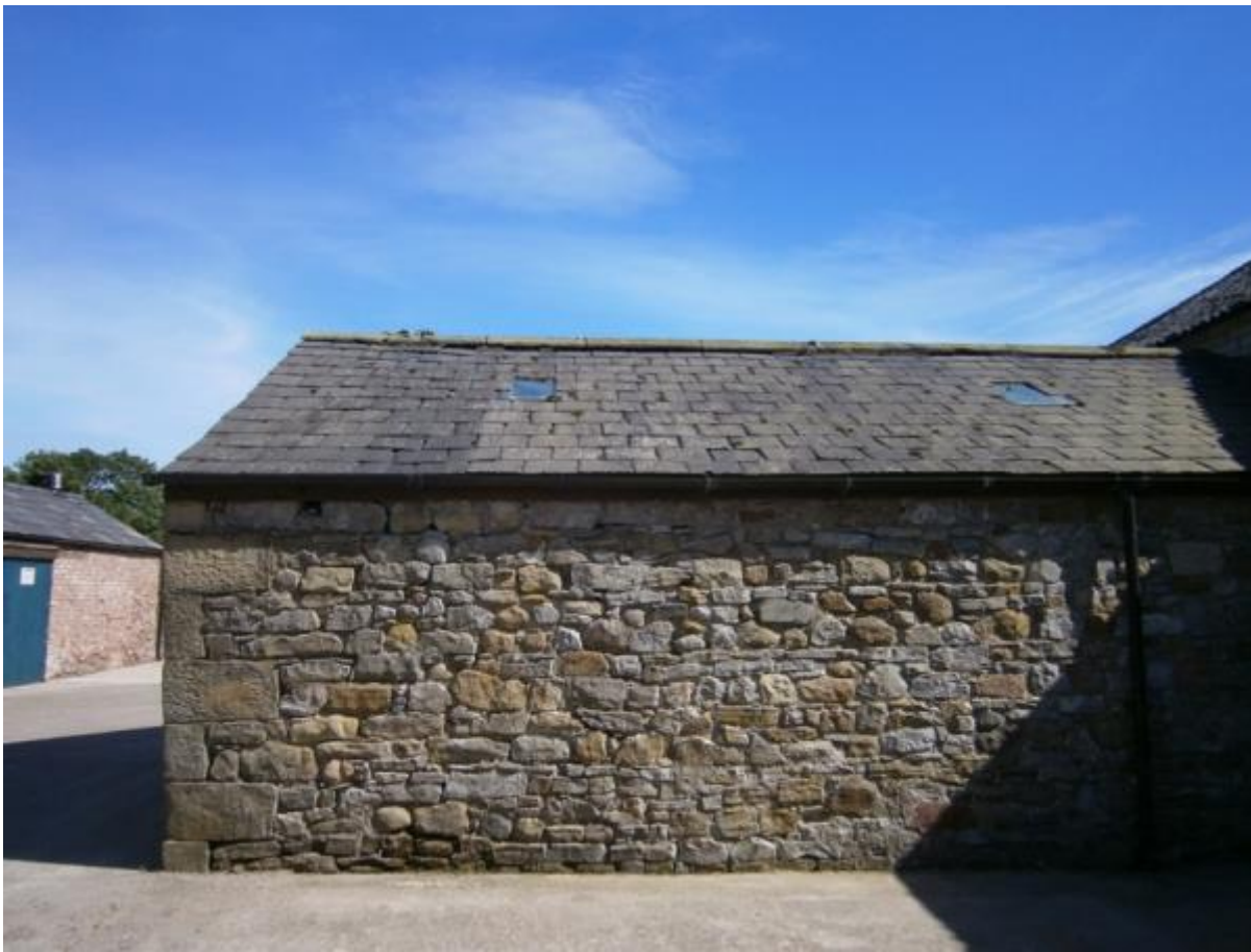
Photo 9 – Opposite side elevation of single story section
