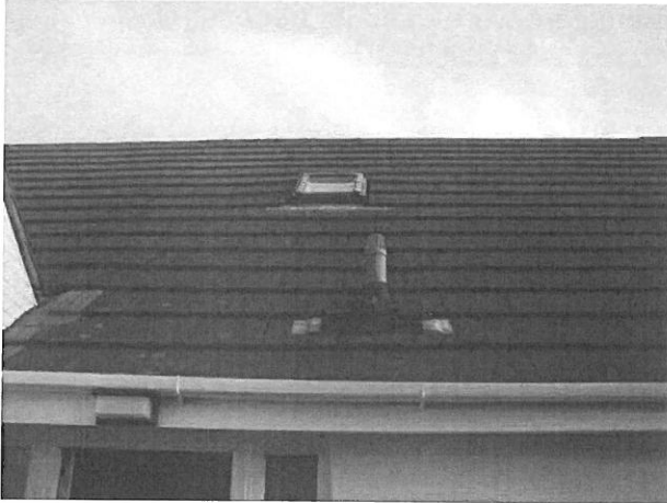
Figure 2 – Side view of roof above front door.
