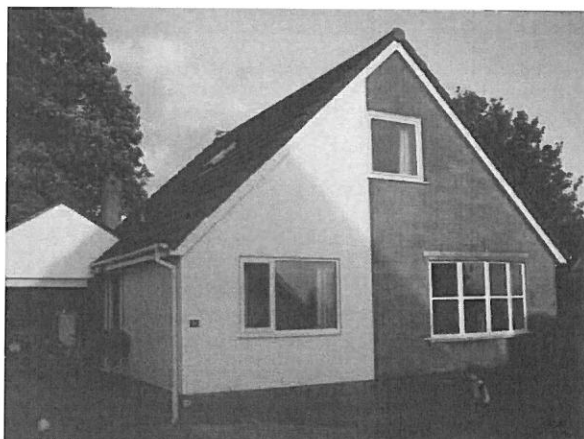
Figure 1 – Front view of the property.
