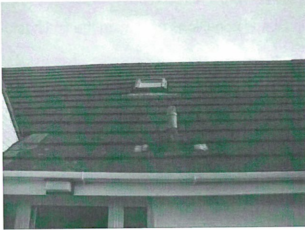
Figure 2 – View of the 'roof light' window.
