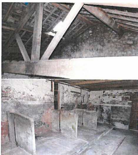
Figure 7: barn 'B' roof
