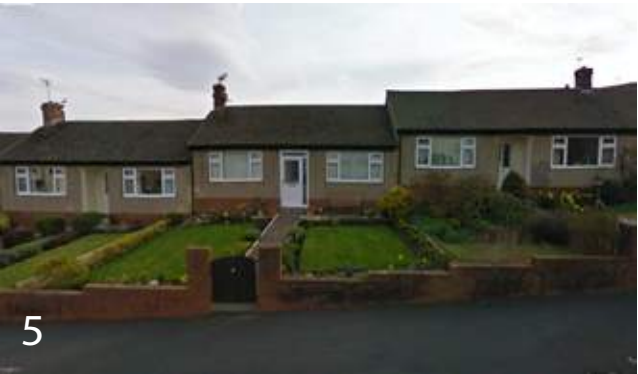
Terraced bungalow dwellings found on Standen Road. Finished in pebble-dash render with tiled roof tiles.
