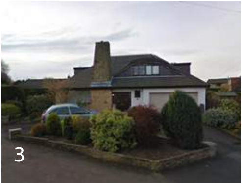
Example of detached dormer bungalow on Peel Park Avenue. Large chimney breast is a prominent feature in the elevation. Parking is to the front and side of the property with an integral garage.
