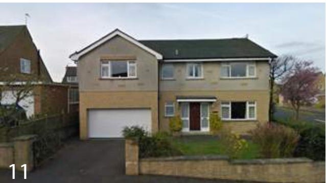
Large detached property on Shays Drive. Finished in render and brick with horizontal emphasis to the windows. Brick detailing within the render is a prominent feature.
