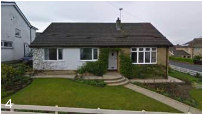
Detached bungalow finished in stone and render. Straight uninterrupted eaves line.
