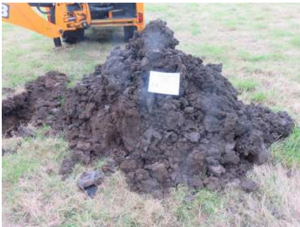
Photo 4 – Arising's Trial Pit 02
