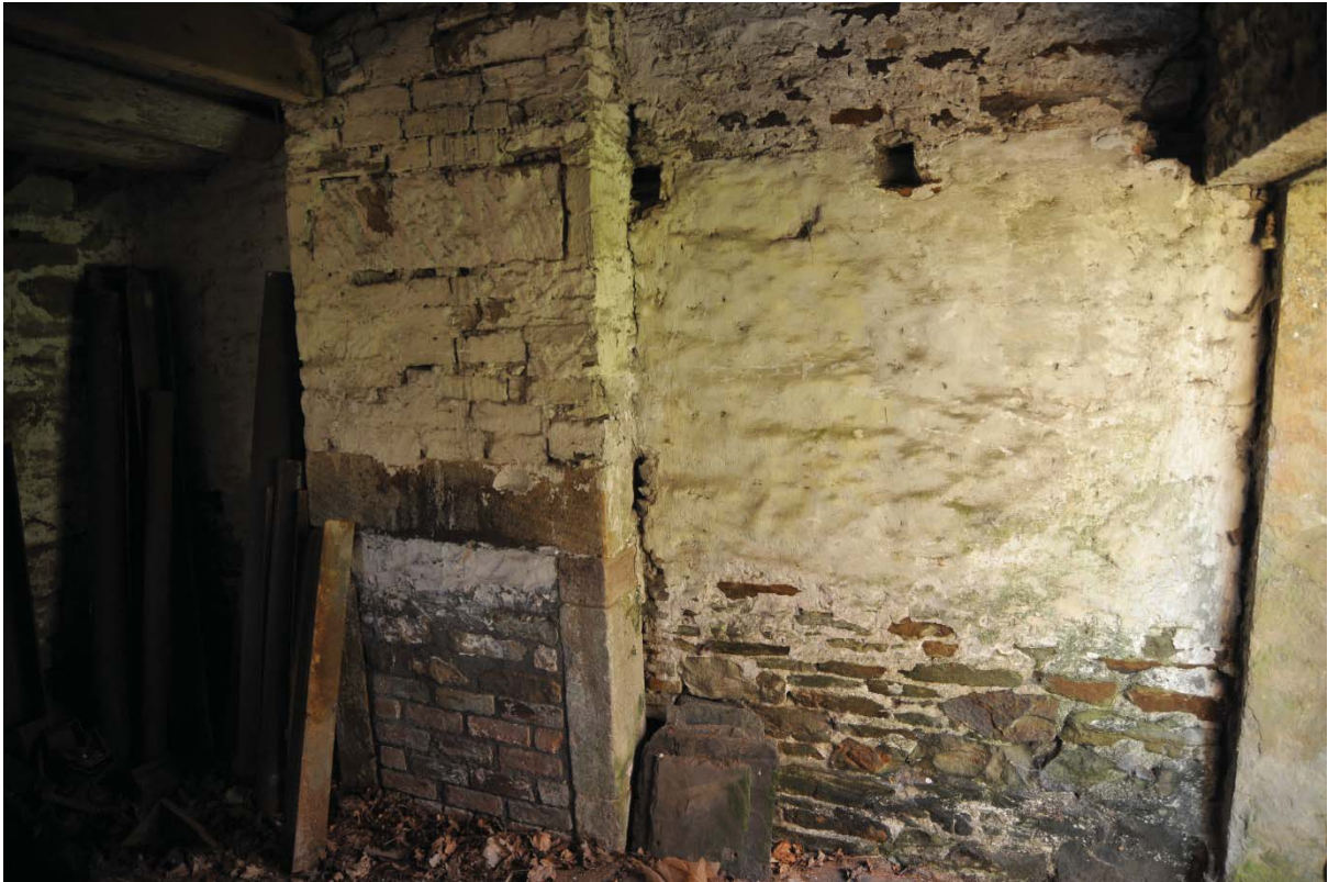
Pl.8: The stack and fireplace, and attic joist sockets, in the north room of the North Range.
