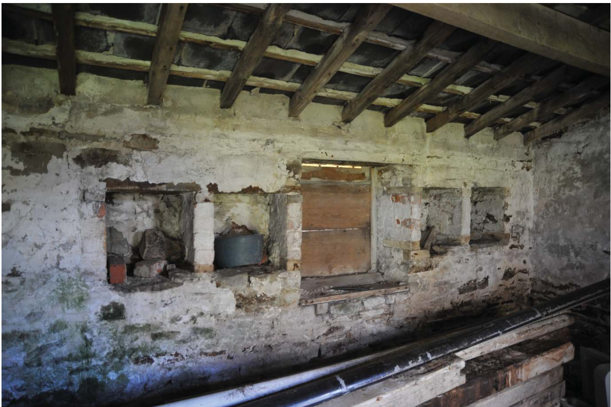
Pl.9: The inner face of the rear wall in the southern room of the North Range.
