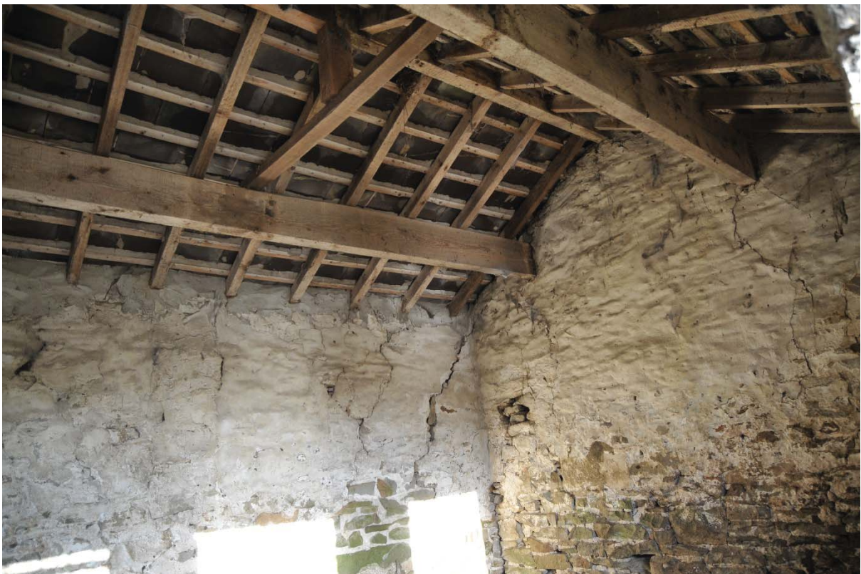
Pl.5: The longer eastern space, showing scar of removed cross-wall and added roof support.
