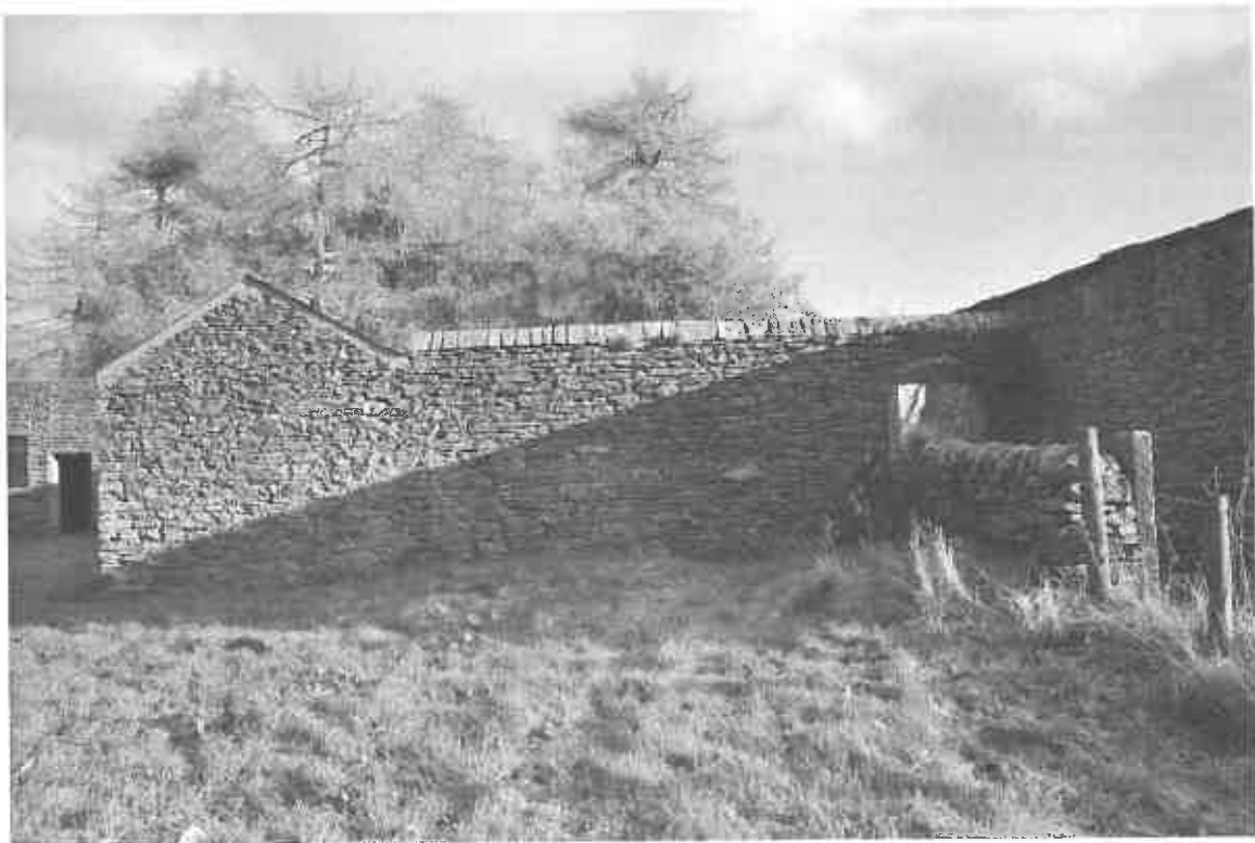
Pl.3: The west side of the South Range and the adjacent front yard.
