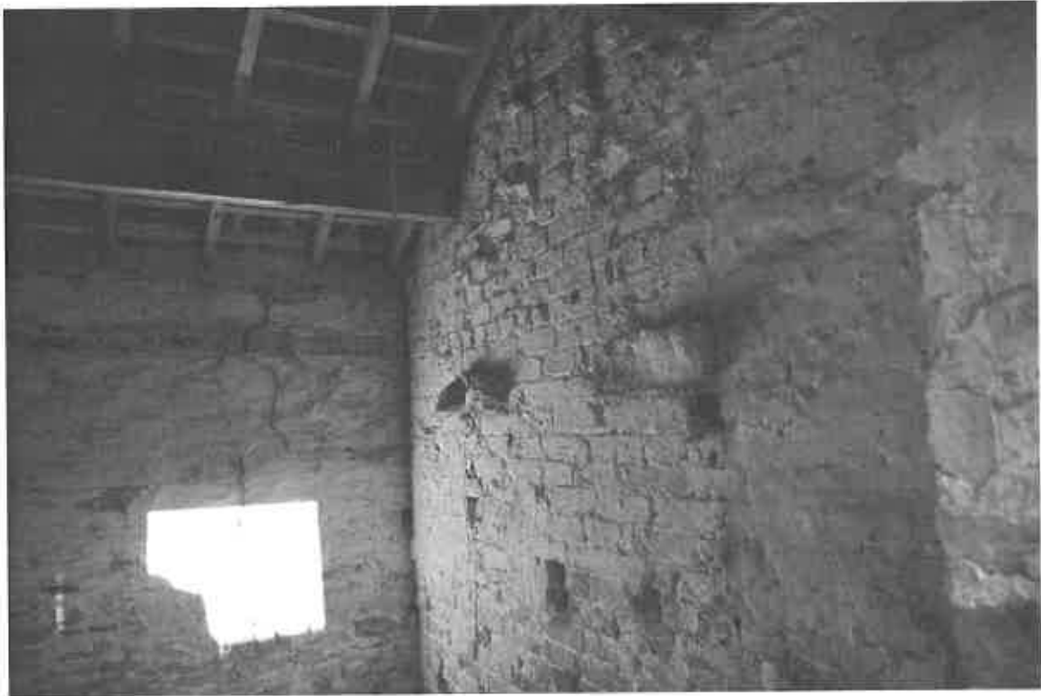
Pl.4: The west side of the western cross-wall, showing traces of the lost stack.
