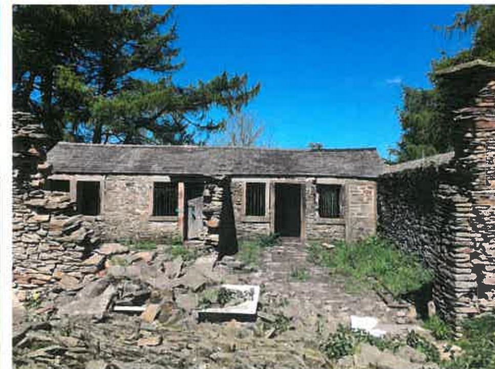
3. North West View
