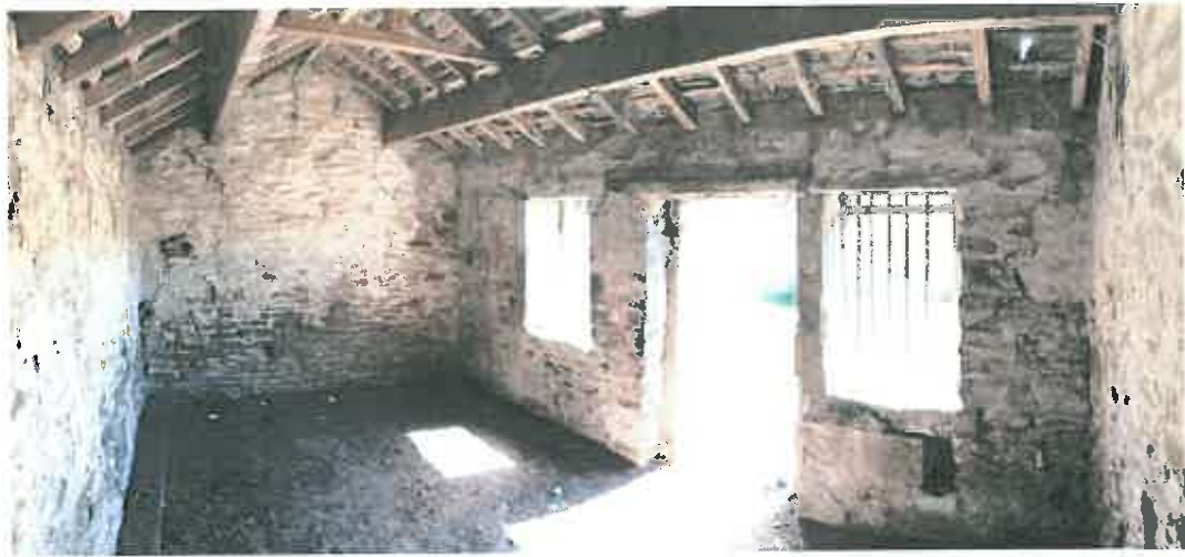
Figure 4. (Southern) Building's interior
