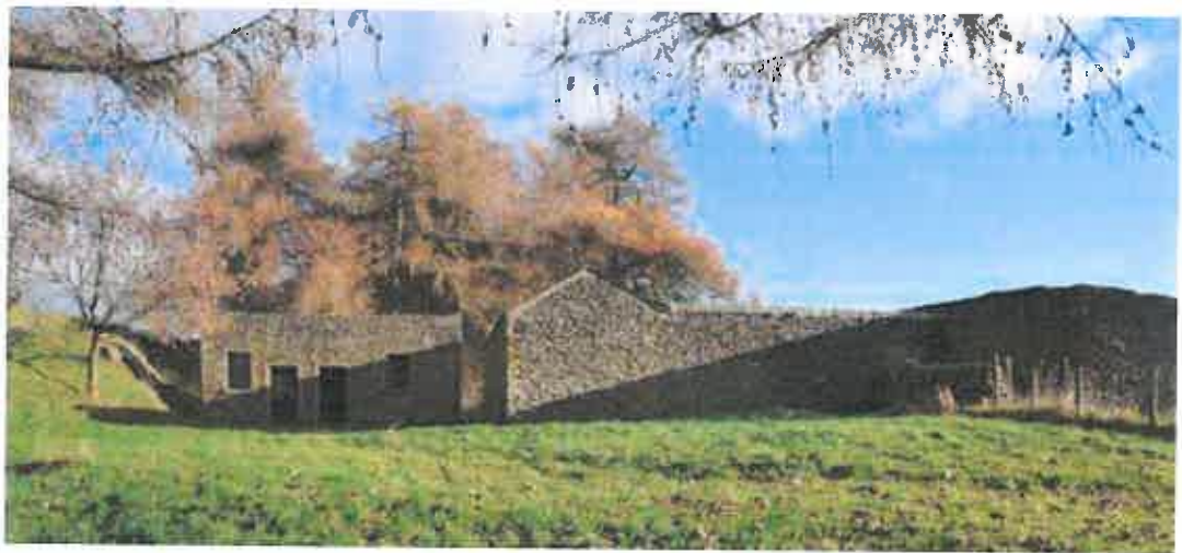
Figure 3. Existing outbuildings – View from West/South-West
