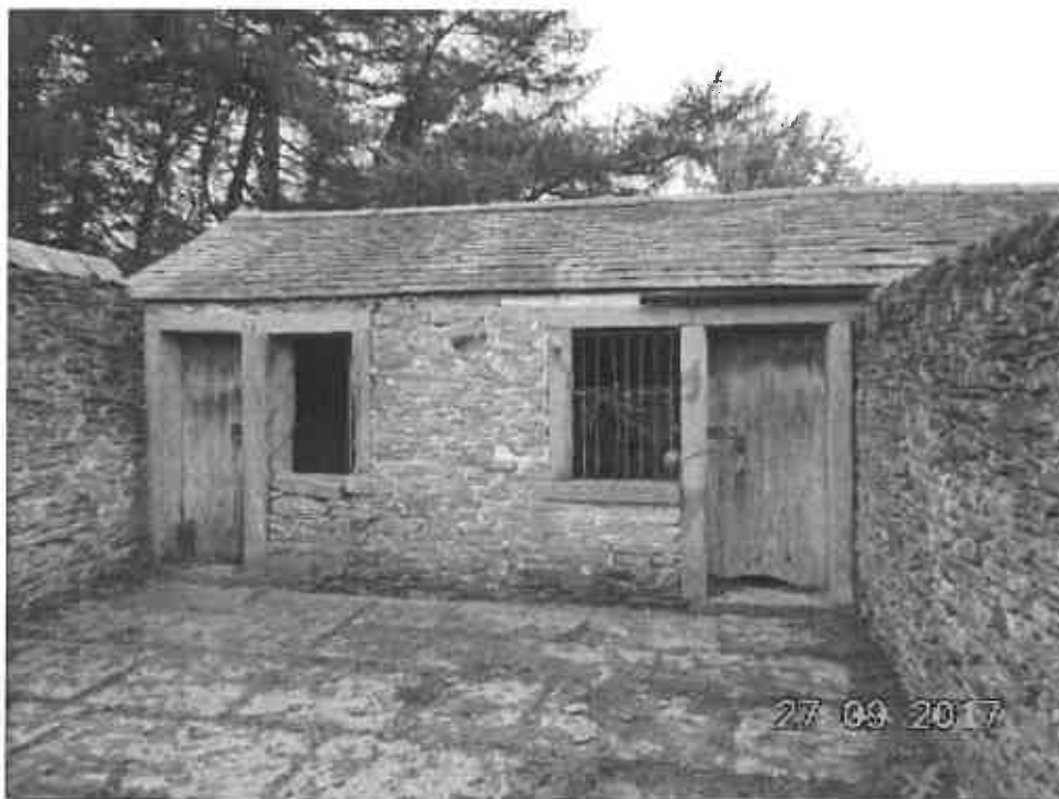
LEFT HAND SIDE OF FRONT ELEVATION (PIGGERY)
