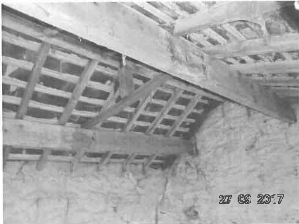
INTERNAL ROOF TO PIGGERY
