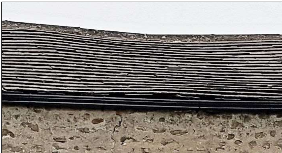
Plate 2. The stone tiled roof was intact but with numerous gaps under tiles.
