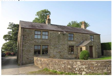
The property is two storey traditional stone built farmhouse with double pitched slate roof, to the front of the farmhouse is a porch with slate roof. Stonework is in good condition and pointing is generally good with no obvious crevices, gaps or cracks present.
