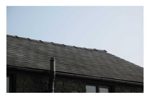
The roofs are in good condition with no lifted or missing slates, ridge tiles are close fitting and pointed leaving no gaps or crevices.
