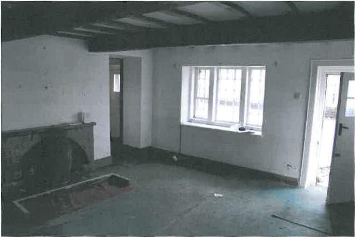
Front ground floor room No 11 fireplace to be removed and replaced with one more in keeping, window and beams to be retained.
