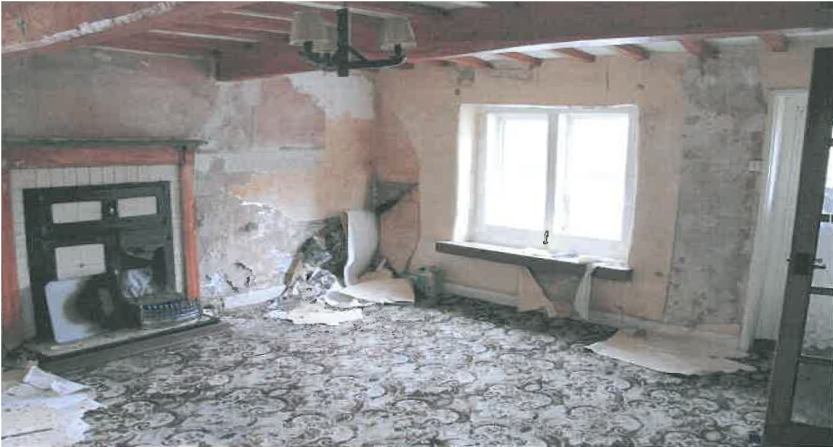
Front ground floor No 13 with Range/fire, window and beams to be retained
