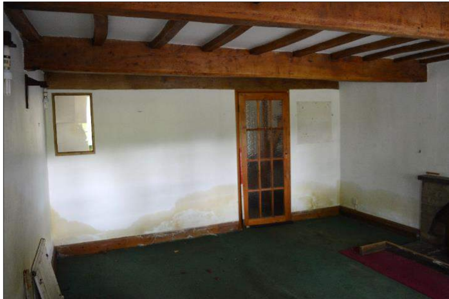
Plate 6: Interior view of No 11 with original timbers in the ceiling and later partition. Looking north, 1m scale
