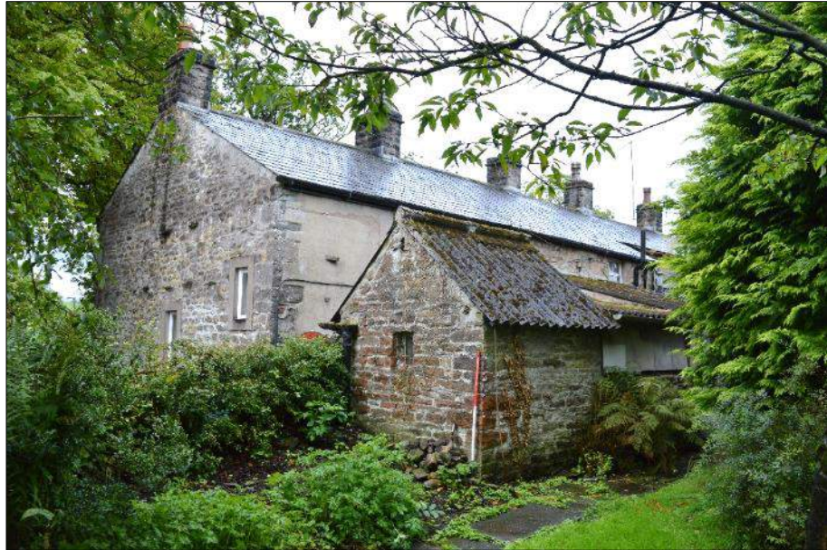
Plate 2: East elevation with through stones shown as ledges and small outbuilding to the rear of the building, looking southwest, 1m scale
