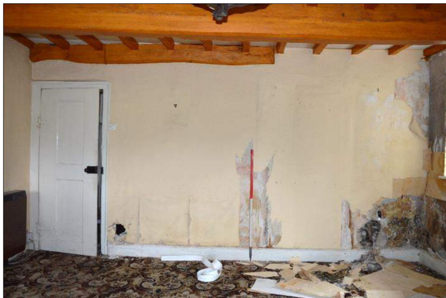
Plate 7: Interior view of No 13 showing original timbers and partition with later doorway to the left and blocked opening to the right. Looking north, 1m scale
