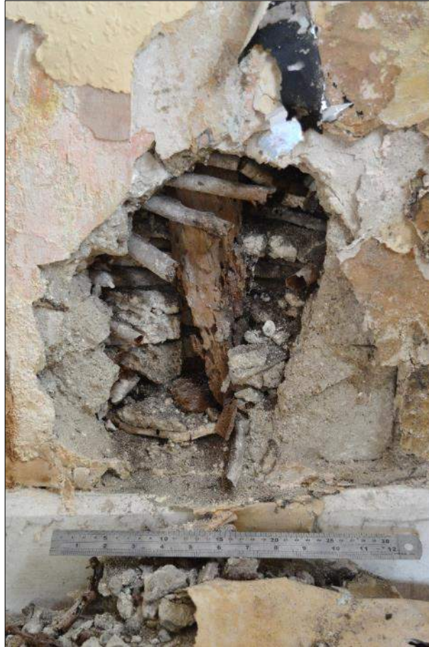
Plate 8: Close up of wattle in partitioning wall in No 13, looking north, scale 0.3m
