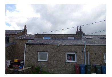
The property is a traditional stone built farmhouse with a double pitched slate roof. The building has a single storey extension with single pitched slate roof to the north. It is well pointed and maintained, roof slates are in good condition and ridge tiles pointed.
