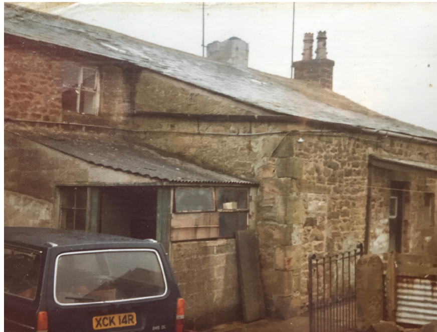
Figure 4 Photo taken in 1979 showing lean-to extension (before the barn was extended)
