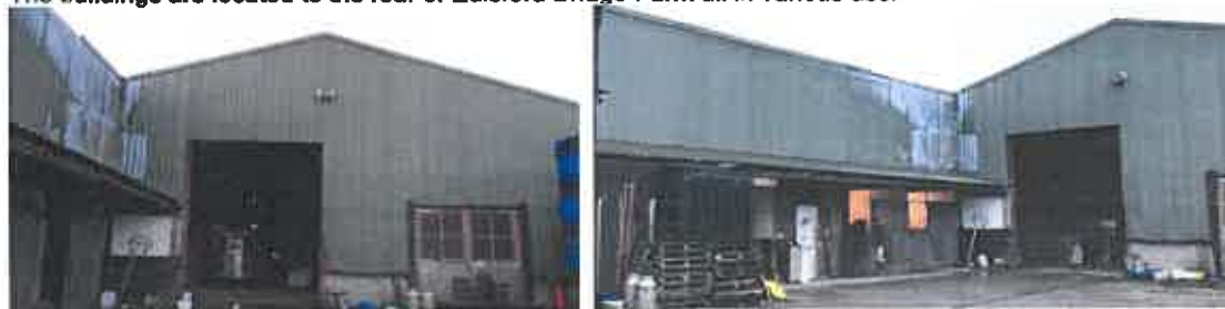
Steel portal frame farm building.
