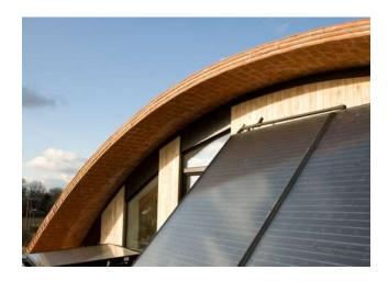
PV-T is an integrated panel that produces both electricity and heat.
