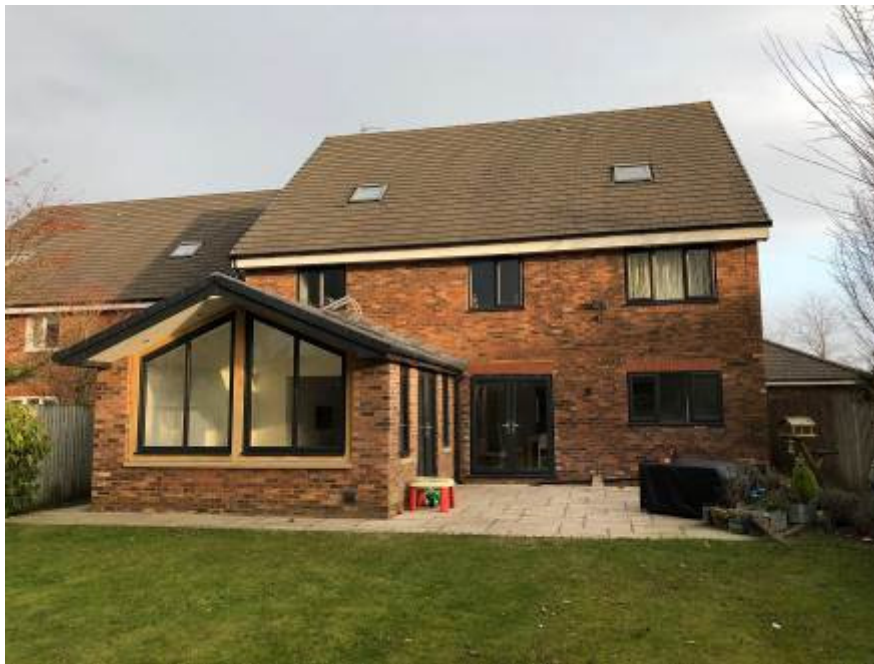
Figure 3. Current photograph of the rear elevation.
