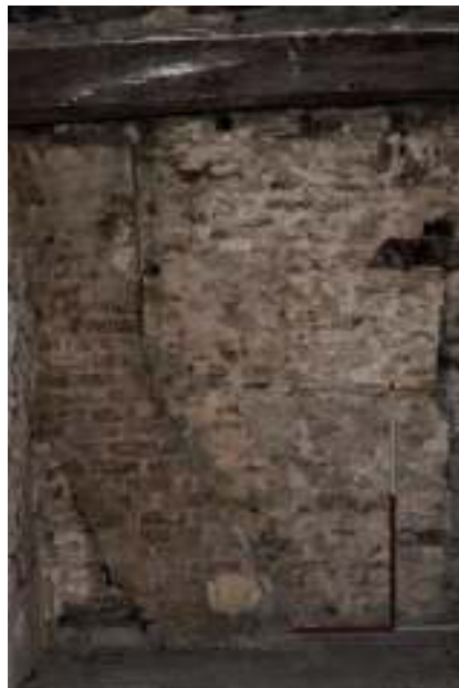
Figure 128. Upper north west room, flue built from ground floor fireplace.
