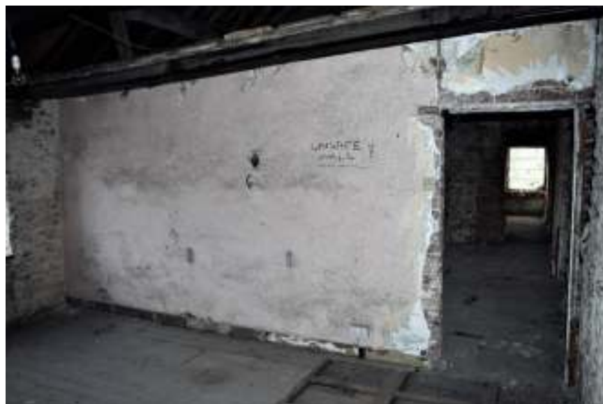
Figure 92. Upper floor, south east, room west wall.
