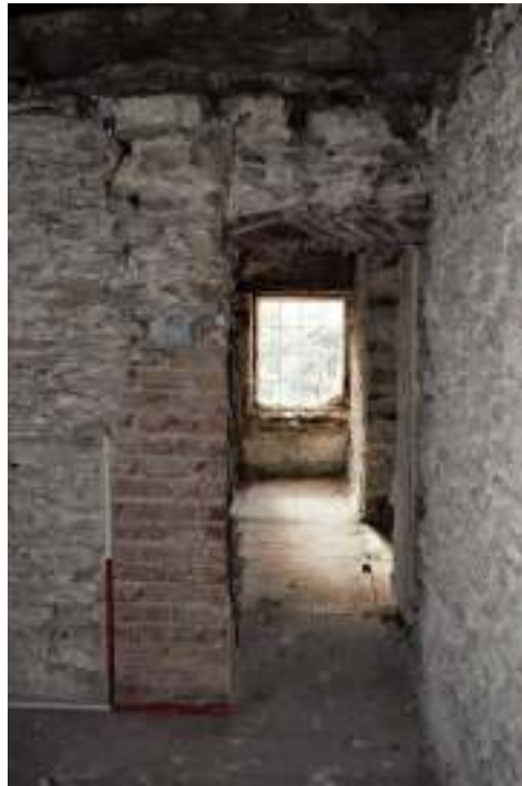
Figure 100. Upper south central room, west wall doorway.
