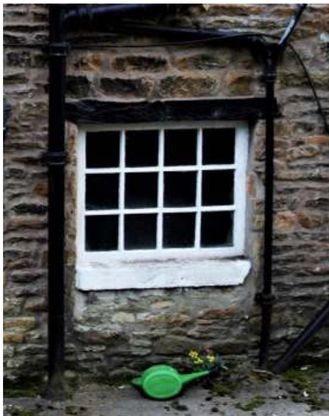
Figure 21. GF4 West end window in former door opening.
