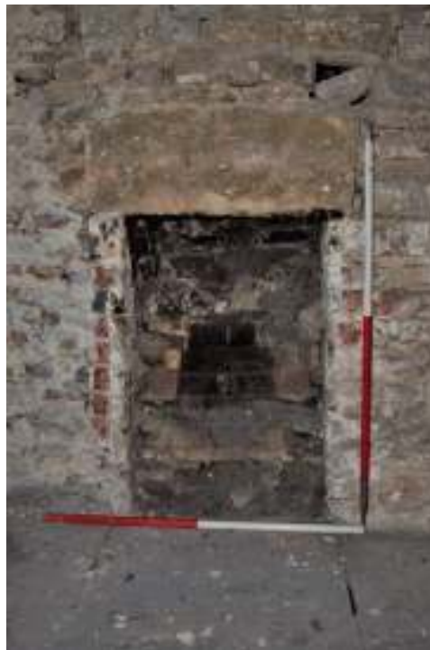
Figure 99. Upper south central room fireplace.
