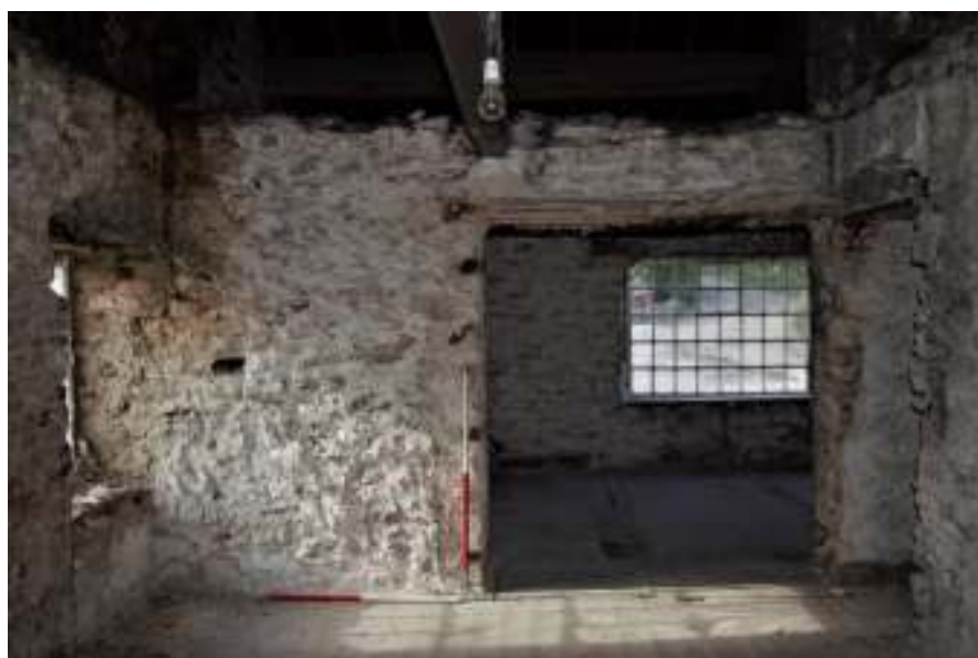
Figure 113 Upper south west room, north wall.
