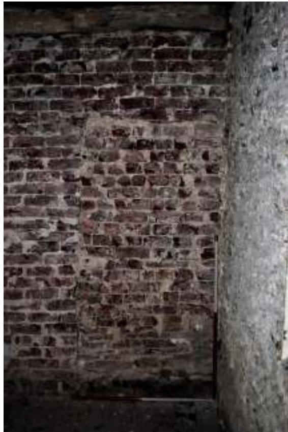
Figure 31. South east room, west elevation, blocked door at northern end.
