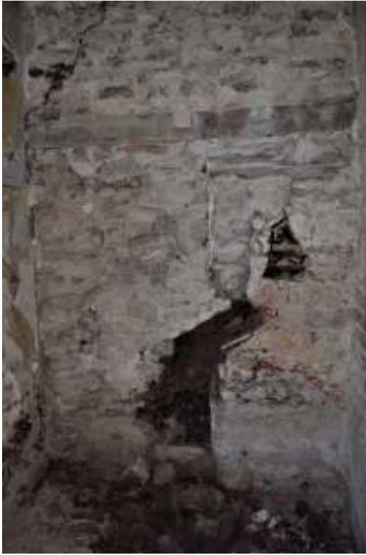
Figure 46. Centre room, opened up flue.
