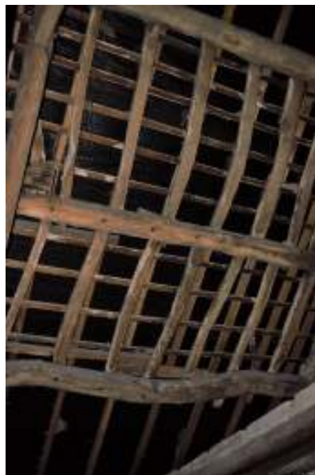
Figure 132 Roof structure with surviving common rafters and re-used timbers as purlins.
