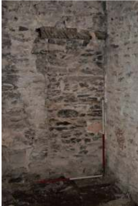
Figure 49. Centre room W elevation north blocked doorway.
