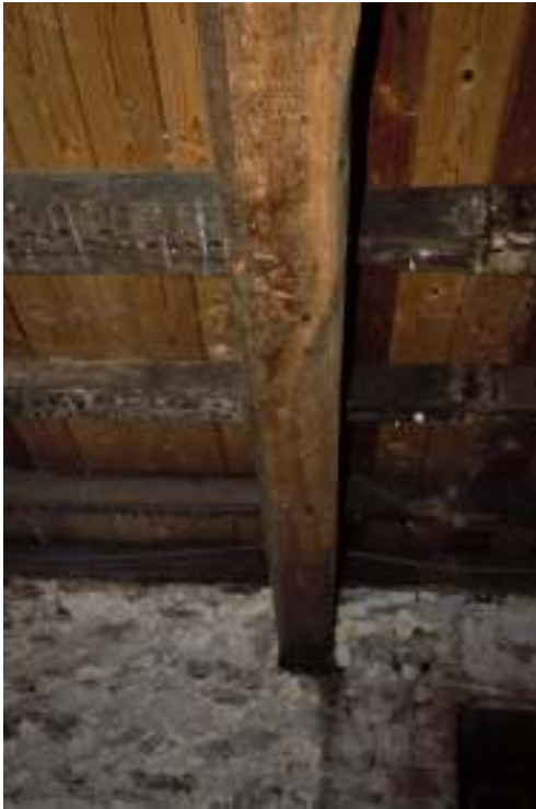
Figure 86. North west room, ceiling beam with sapwood on right.
