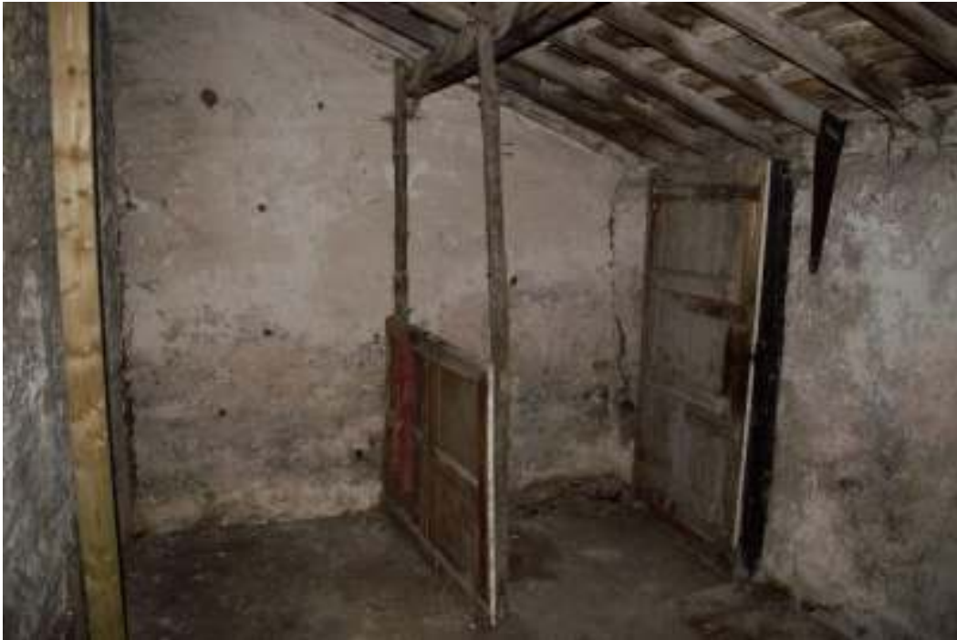
Figure 143 Stalls against south gable of lean-to.
