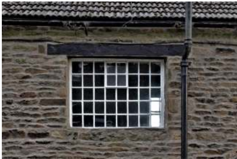
Figure 20. FF4 West end first floor window.
