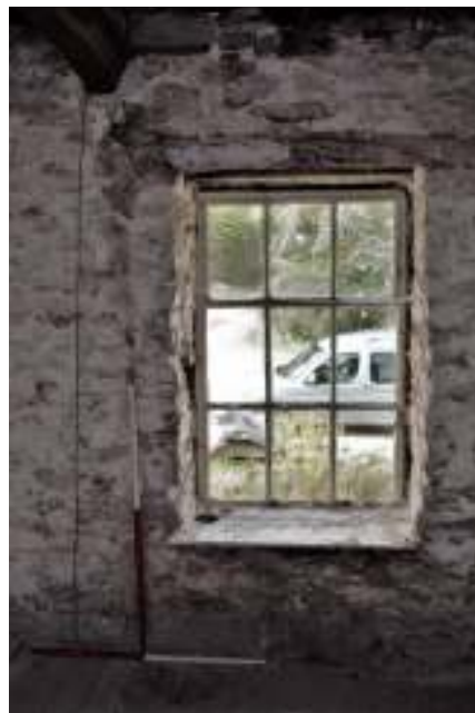
Figure 116. Upper north east room central window.
