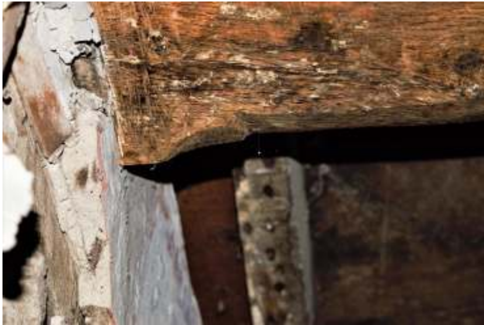
Figure 87. North west room, detail of stop on beam.
