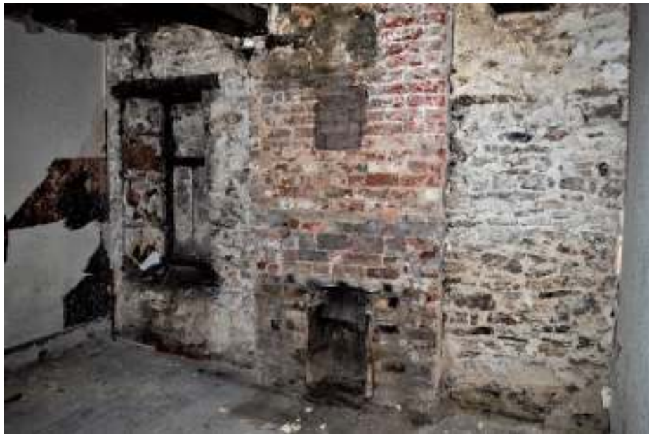
Figure 55. Southwest room, west elevation.
