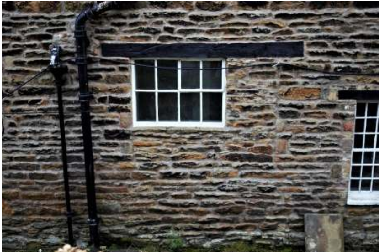
Figure 15. Window in part blocked opening under wooden lintel.
