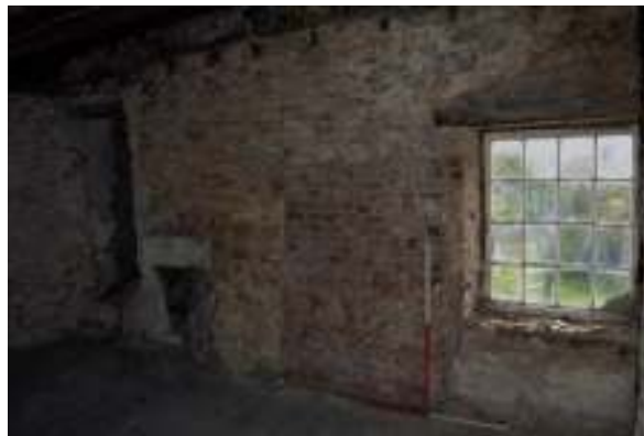
Figure 108. Upper south west room, west wall.
