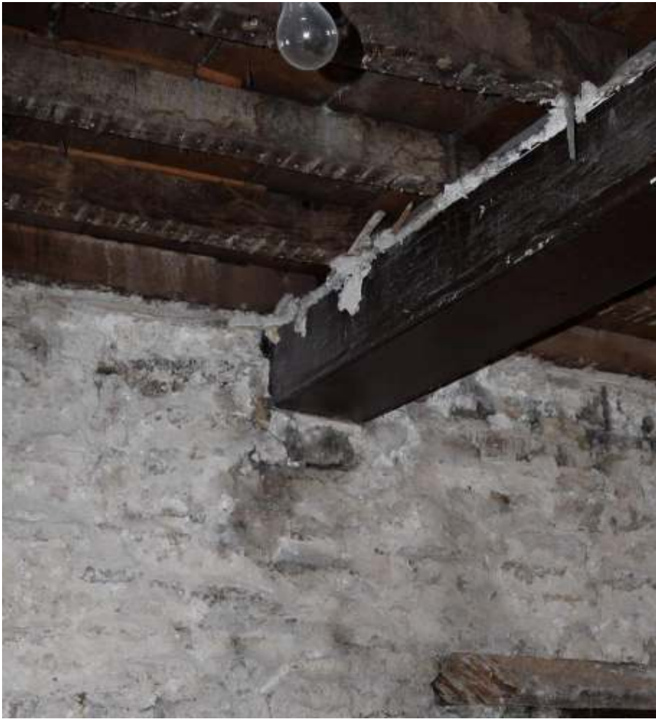
Figure 65. Southwest room ceiling beam entry point to eastern wall.
