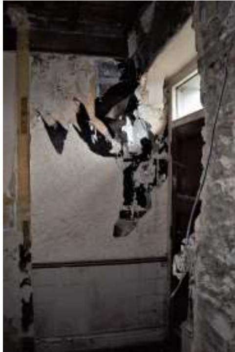
Figure 53. Entrance lobby traces centre room west elevation.
