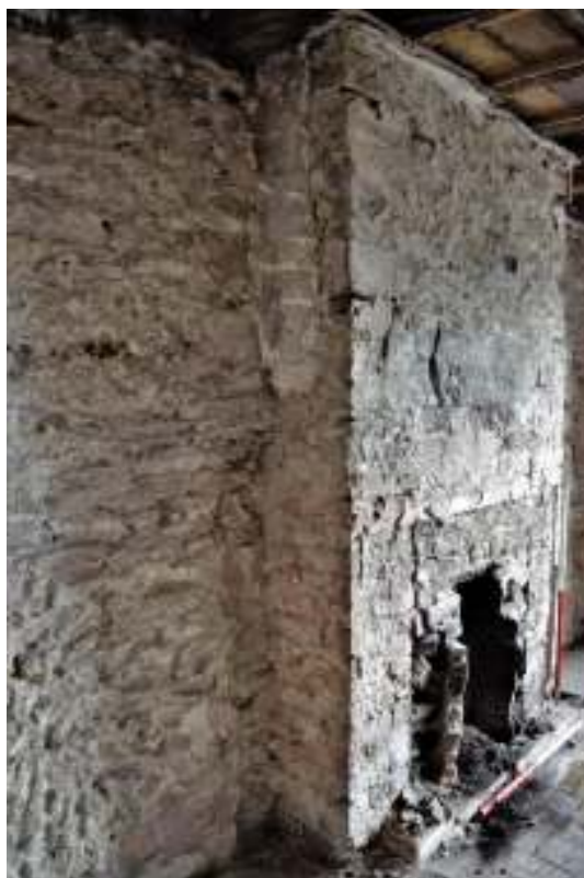
Figure 37. South east room, chimney breast straight joint with wall.
