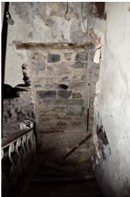
Figure 74. Stairwell , blocked door in south wall.
