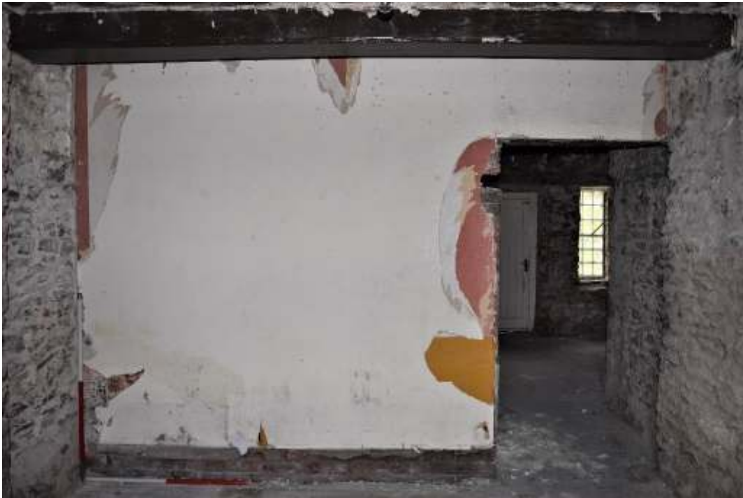
Figure 61. Southwest room, north elevation.
