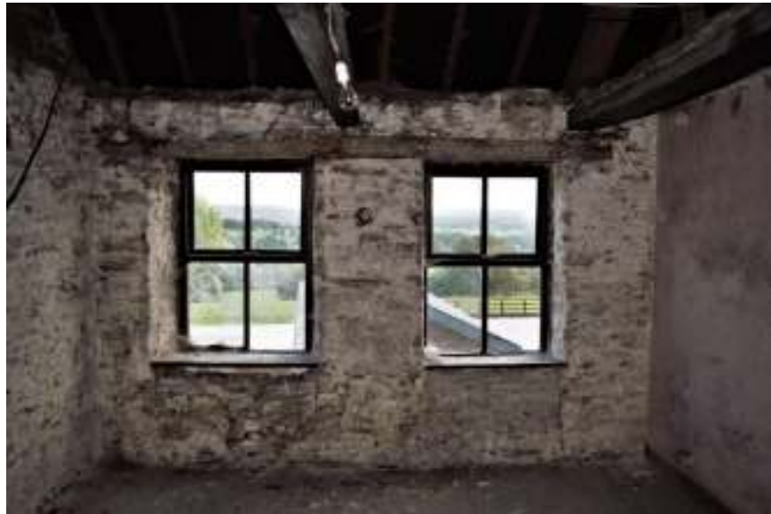
Figure 91. Upper floor south east room, south wall.
