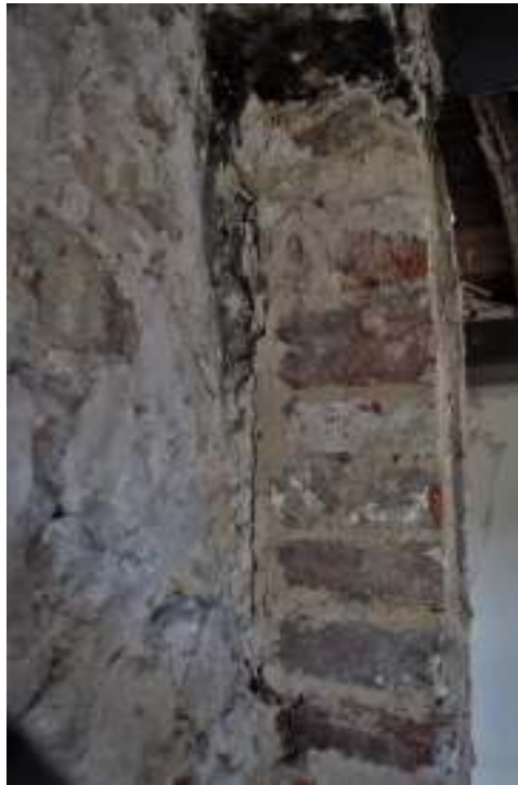
Figure 59. Southwest room chimney breast over original wall plaster.
