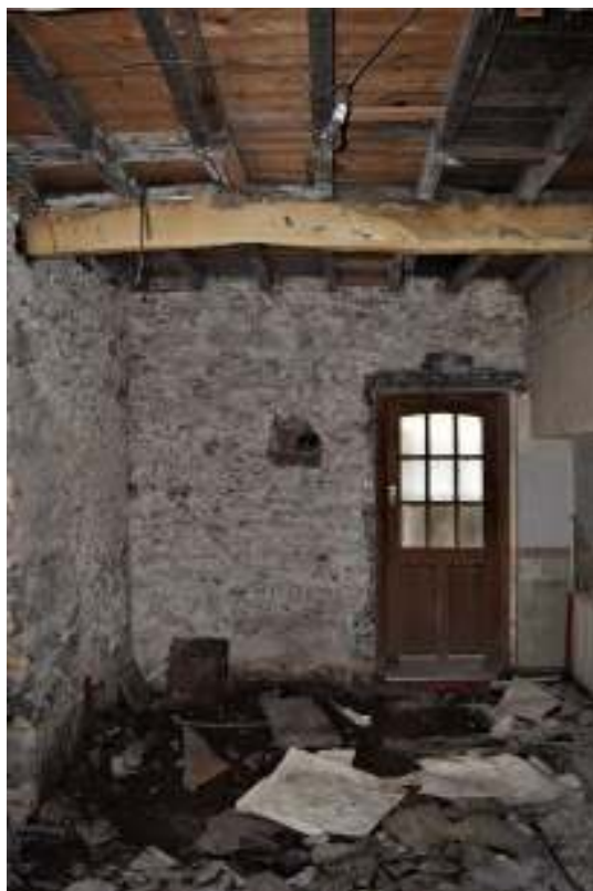
Figure 67. Northeast room east elevation.
