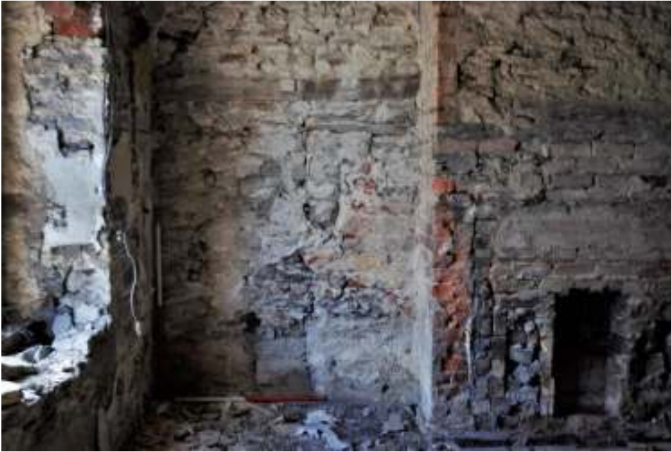
Figure 45. Centre room flue inserted into south door blocking.
