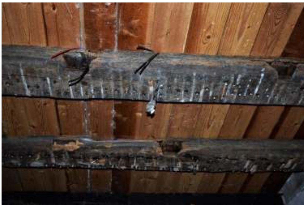
Figure 88. North west room, ceiling joists of re-used timbers.
