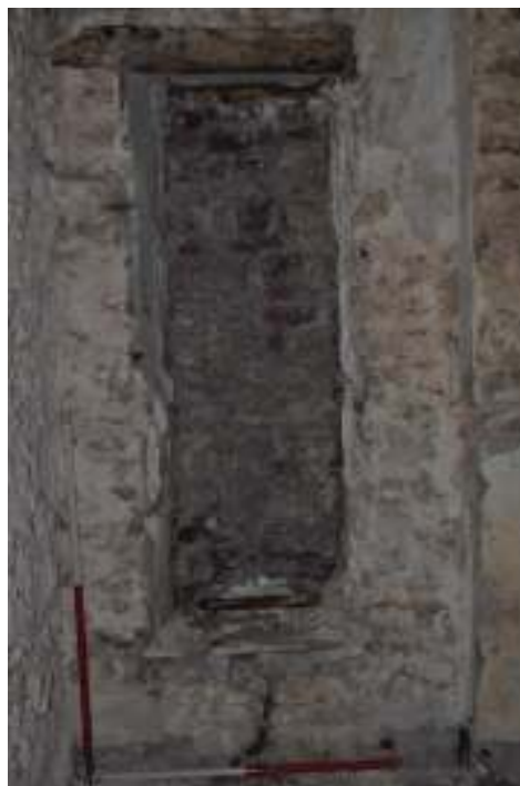
Figure 109. Upper south west room, blocked window in west wall.
