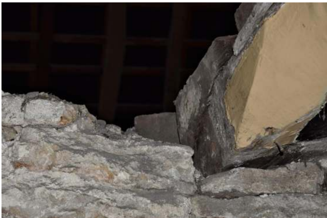
Figure 123 Upper north east room ceiling beams.
