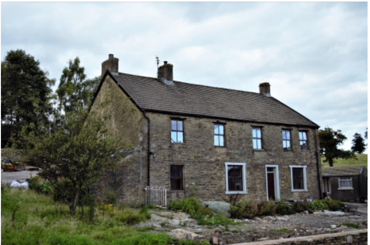
Figure 5. South elevation from south west.
