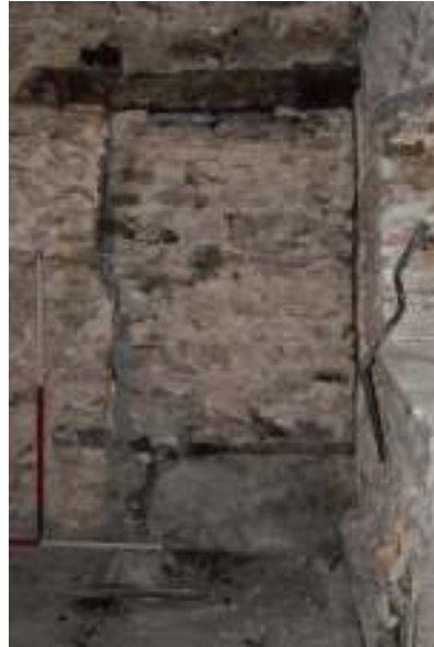
Figure 129. Upper north west room, west wall blocked window.
