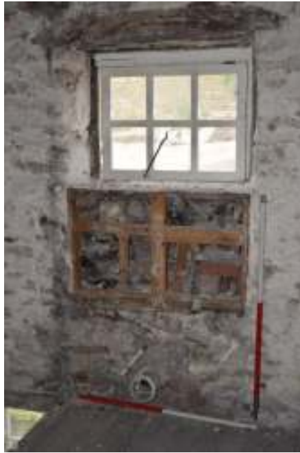
Figure 117. Upper east room, western window.
