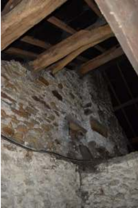
Figure 114. Upper south west room gable former window.
