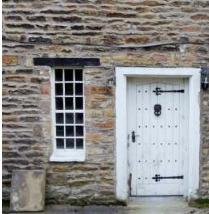
Figure 18. Ground floor window.
