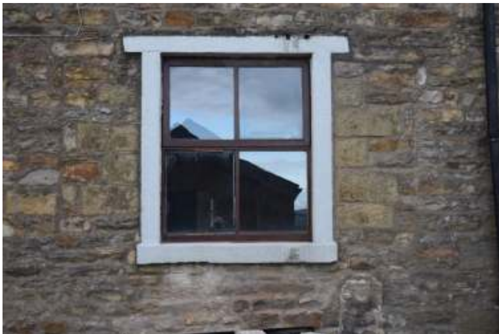
Figure 8. South elevation, east window with blocking of earlier opening.
