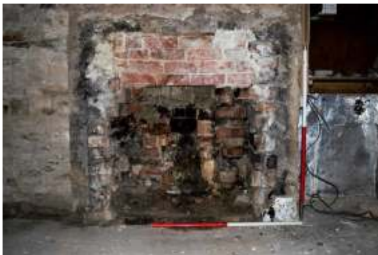
Figure 83. North west room, details of firebox reduction in fireplace.
