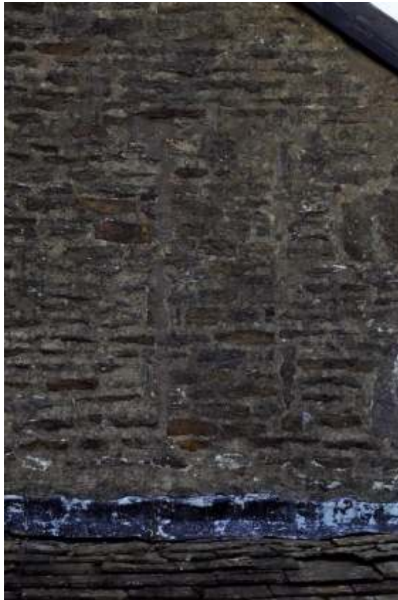
Figure 27. Blocked window to south west first floor room.
