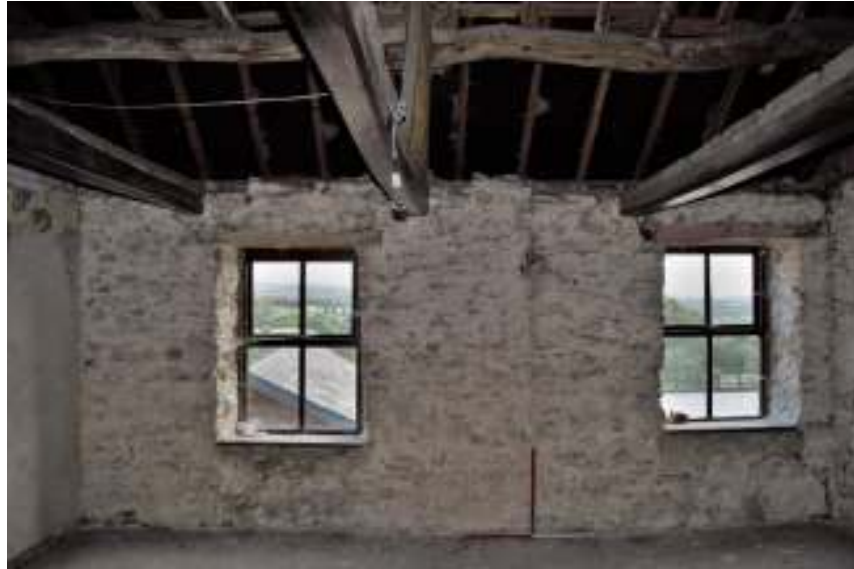
Figure 97. Upper south central room south wall.
