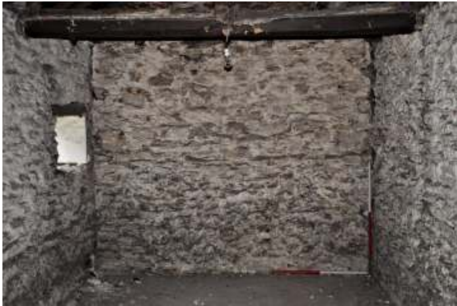
Figure 122 Upper north east room, east elevation.
