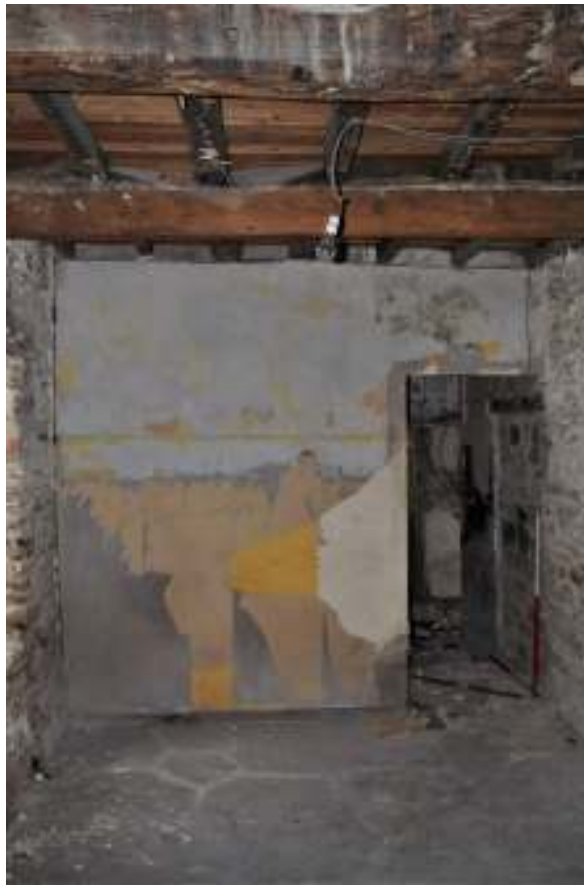
Figure 77. North west room east wall.
