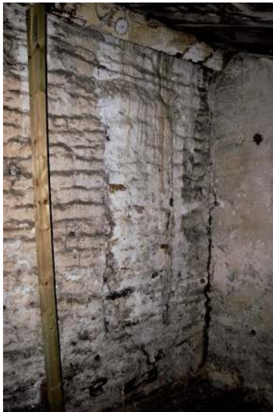
Figure 26. West gable, blocked window to SW room of house. For the use of PWA Planning and Mrs and Mrs McHugh.
