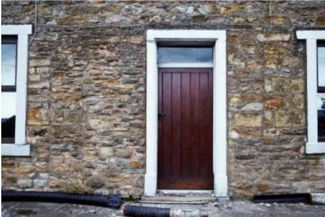
Figure 7. South elevation, door and altered door and windows.
