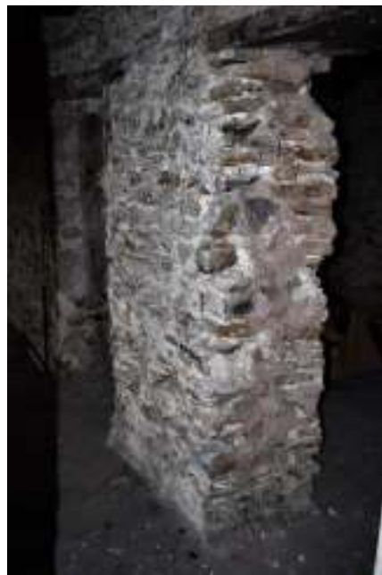
Figure 107. Upper south central room east door jamb detail.
