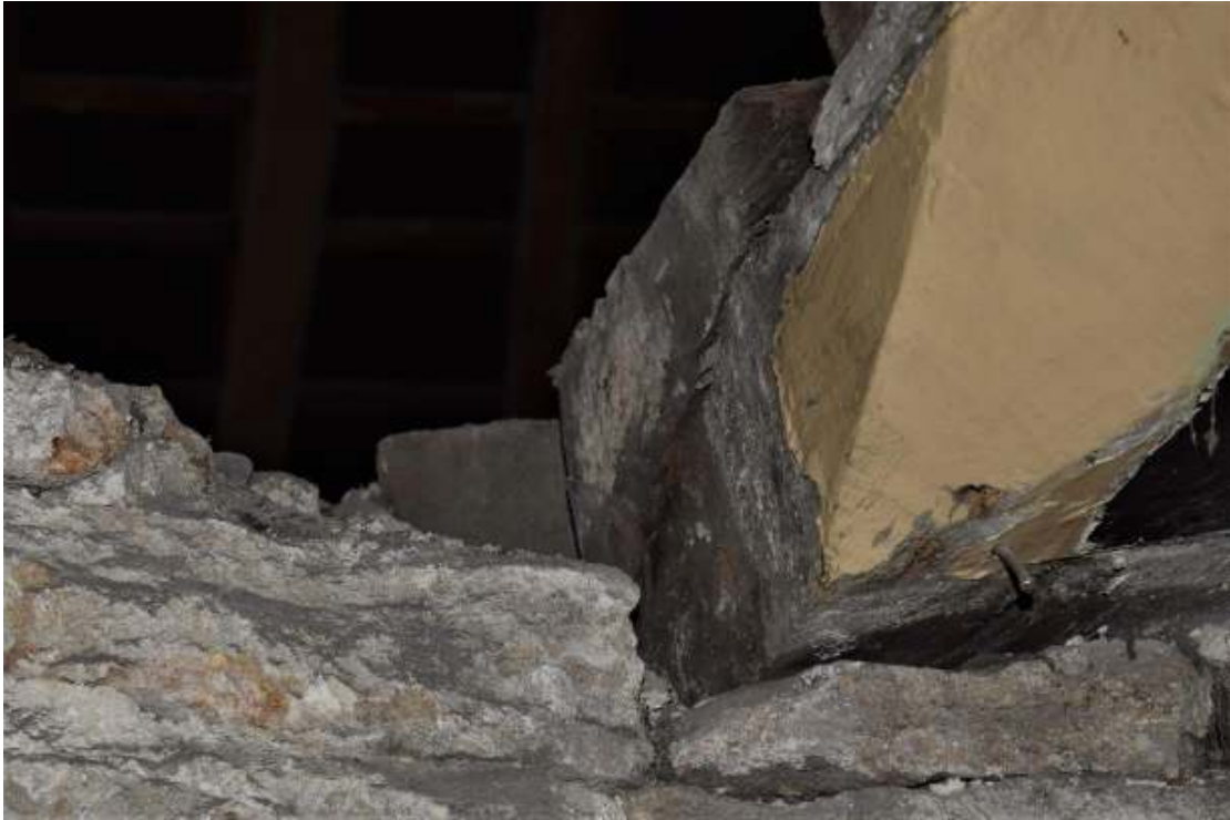
Figure 124. Upper north east room, butted ends of ceiling beams.
