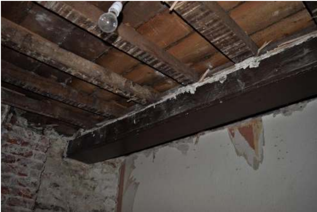
Figure 64. Southwest room ceiling beam.
