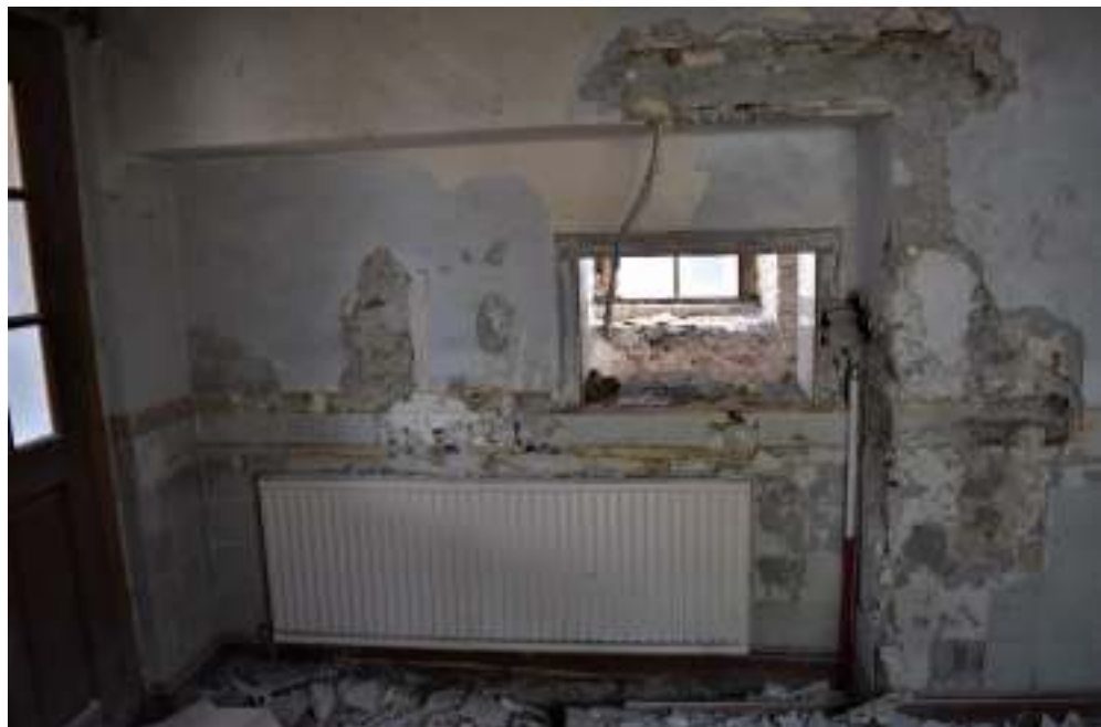
Figure 69. Northeast room south wall recess features detail.
