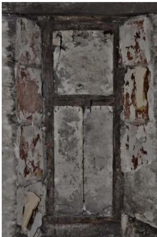
Figure 57. Southwest room, west elevation window frame.
