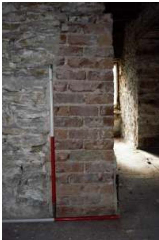
Figure 101 Brick corner on north of chimney breast.
