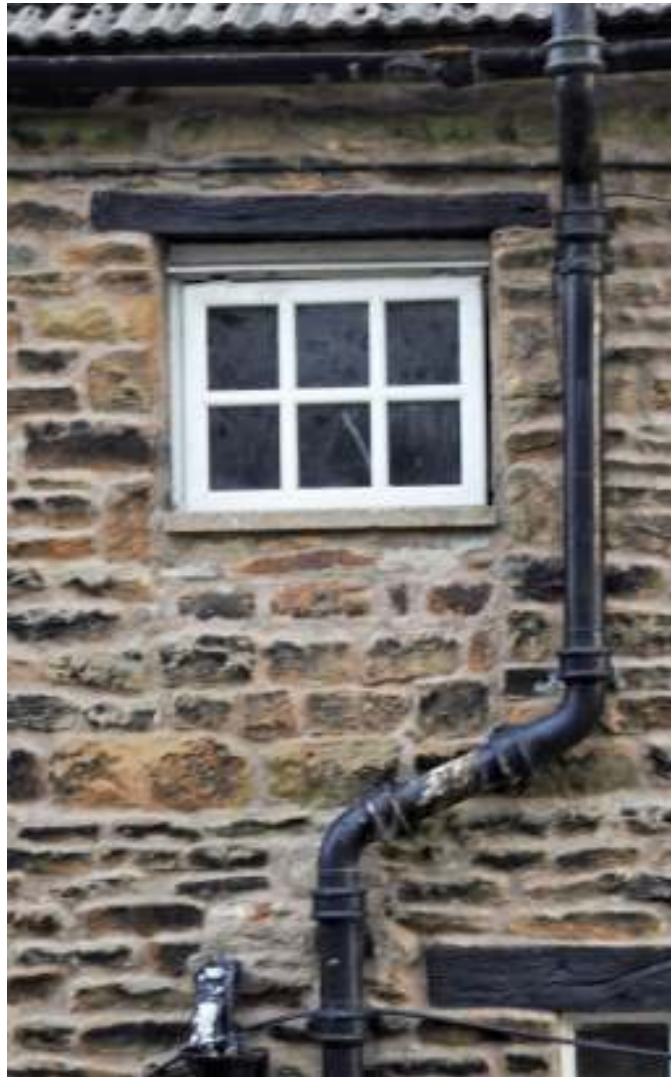
Figure 16. First Floor 3, window in reduced opening.
