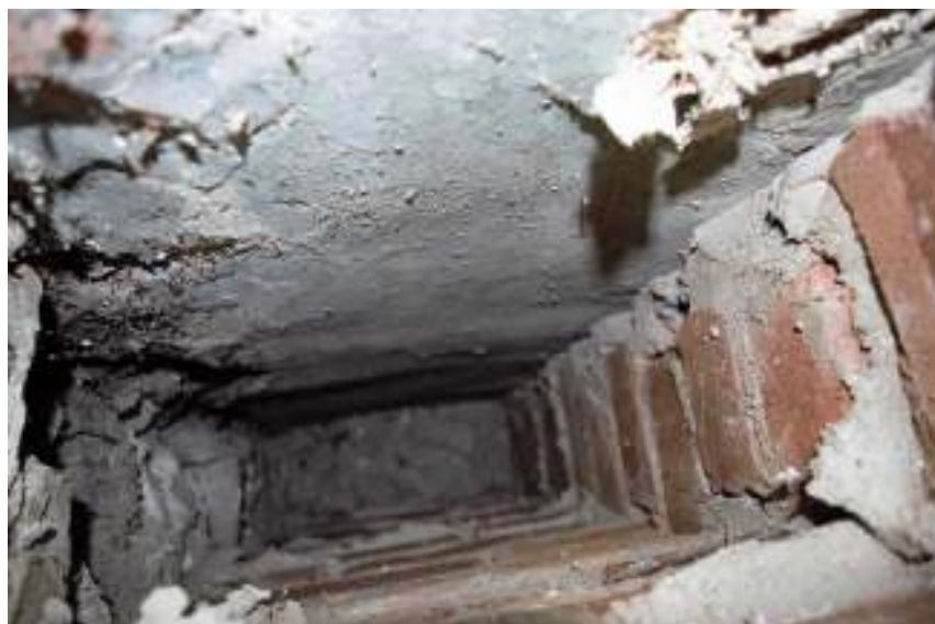
Figure 103. Interior of brick corner from top.
