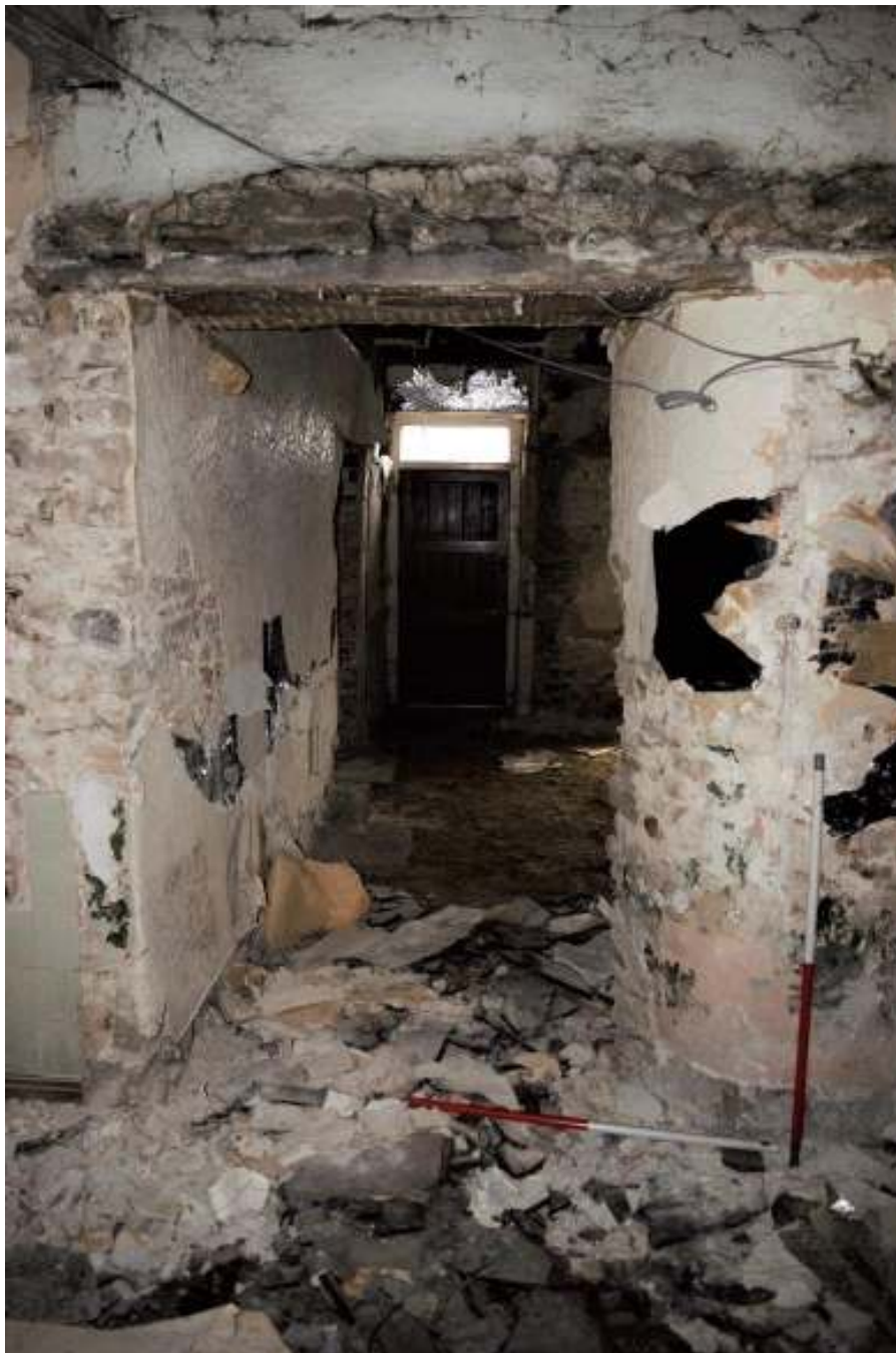
Figure 70. Northeast room S wall, door to S rooms and front door.
