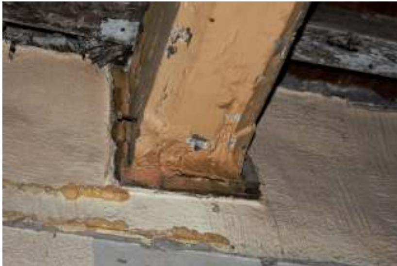
Figure 73. Northeast room, ceiling beam chamfer and stops.
