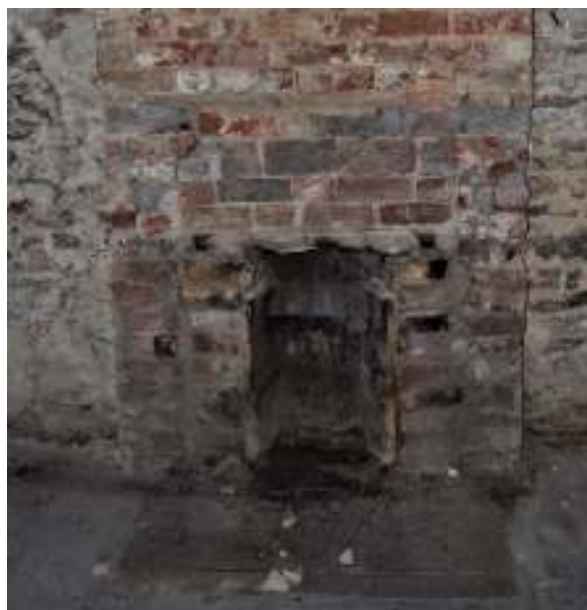
Figure 60. Southwest room west elevation fireplace with details of alteration.
