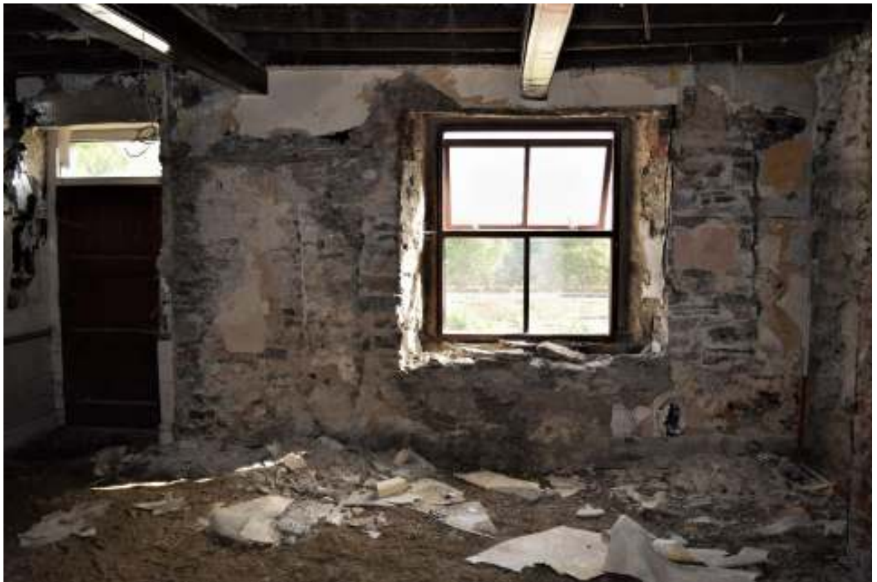
Figure 41. Centre room, south elevation.
