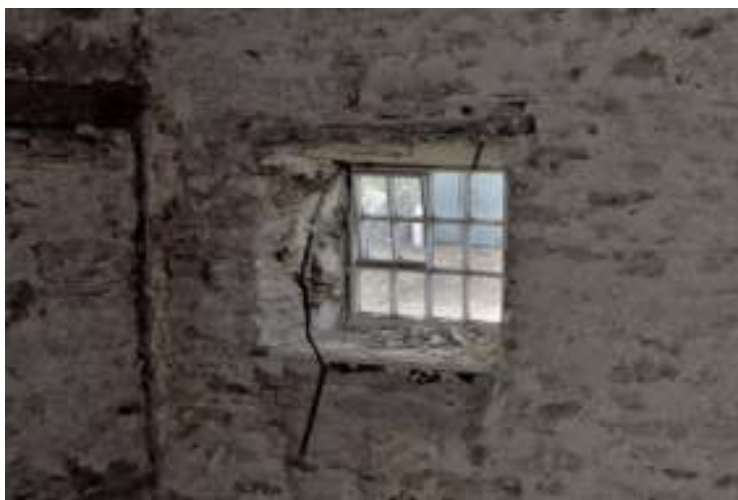
Figure 126. Upper north west room, north wall, west window.
