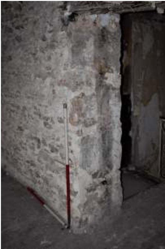
Figure 106 Upper south central room, west doorway, jamb detail.
