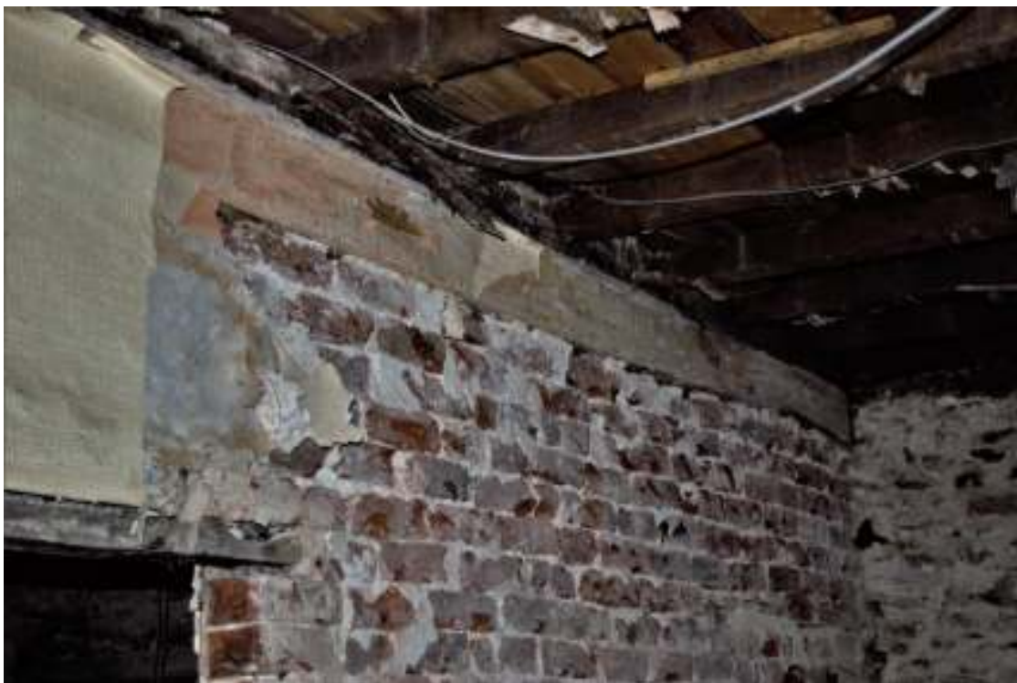
Figure 34. South east room, inserted brick wall below ceiling beam.
