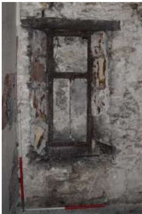
Figure 56. Southwest room, former window splay in west elevation.
