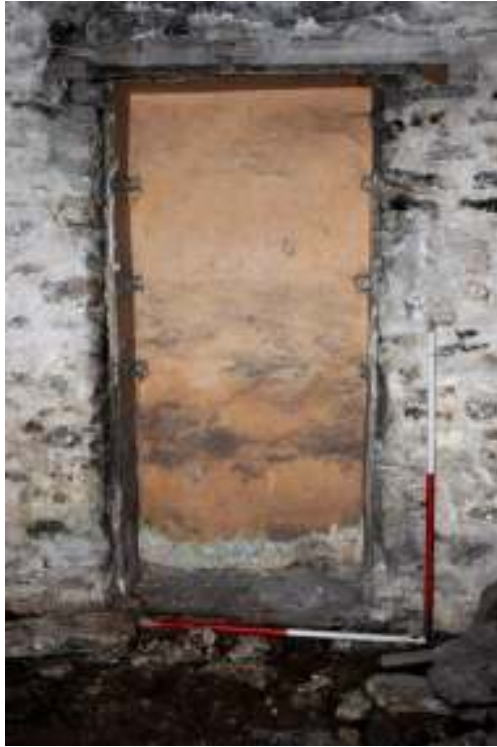
Figure 51. Centre room north elevation cupboard in blocked doorway.
