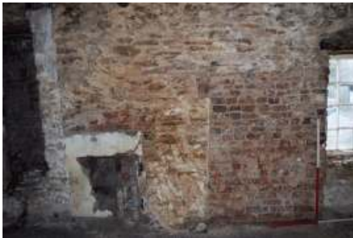
Figure 111. Upper south west room, chimney breast.
