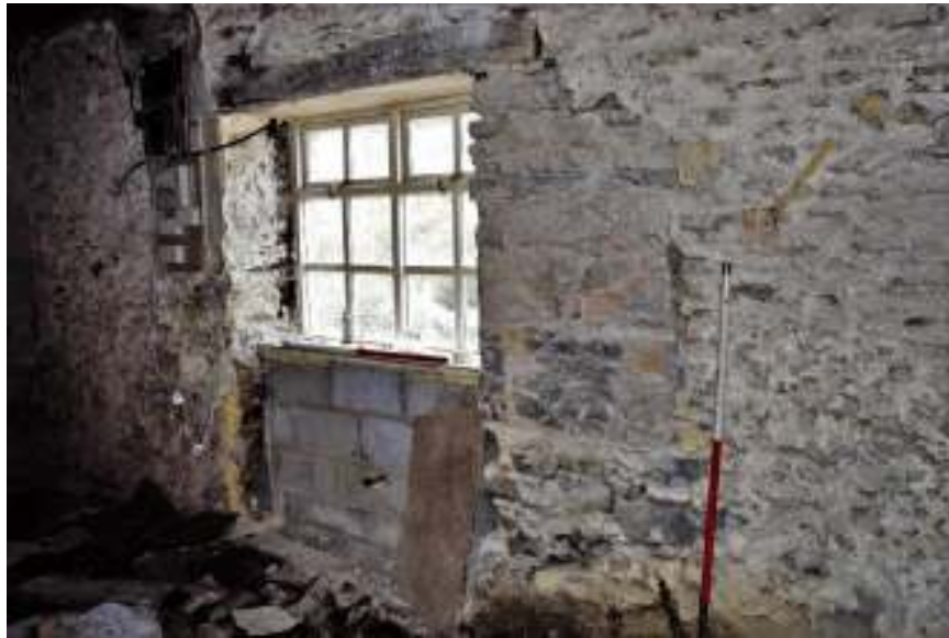
Figure 66. Northeast room, north elevation window detail.
