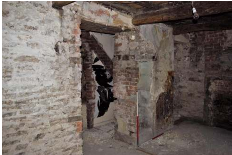
Figure 78. North west room, south wall doorways.
