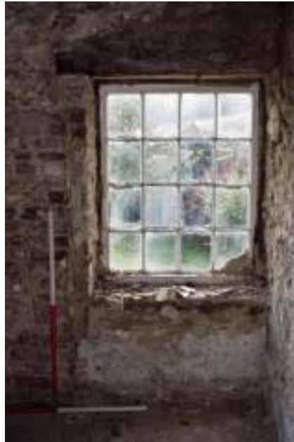
Figure 112. Upper south west room west wall window.
