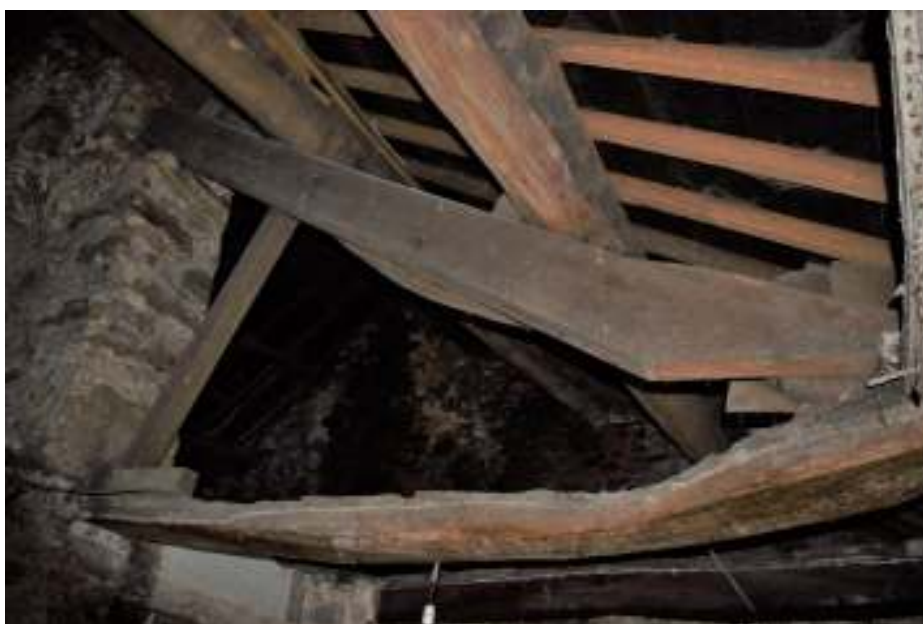
Figure 134 West half truss with reinforcing members.
