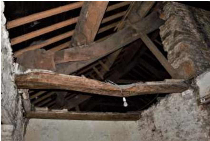
Figure 133 Upper floor, north west room, roof half truss.
