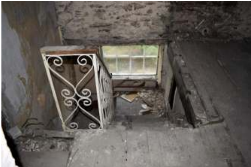
Figure 118. Upper north east room stairwell.
