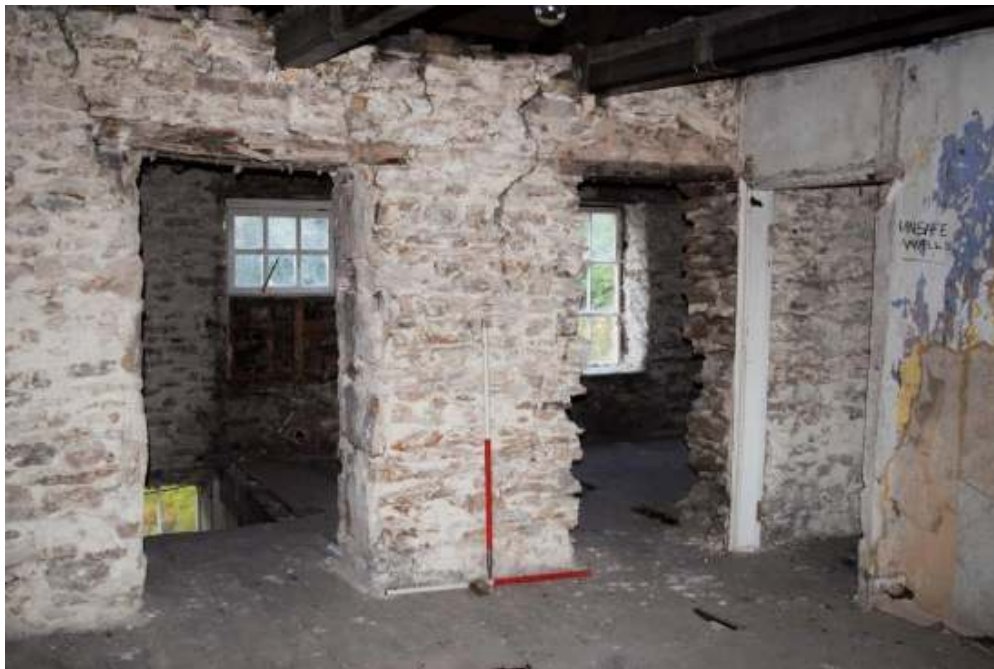
Figure 104 Upper south central room, north wall.
