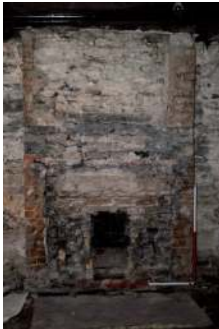
Figure 47. Centre room W elevation Fireplace and chimney breast.
