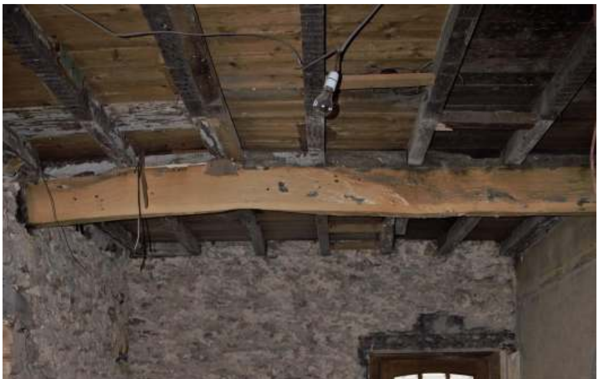
Figure 72. Northeast room, ceiling beam.
