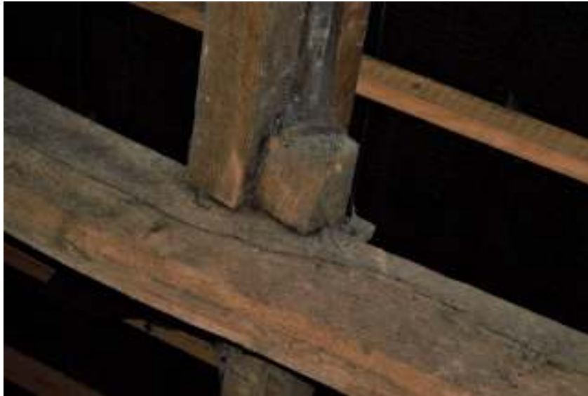
Figure 131. Purlin overlap at truss with retaining peg below.
