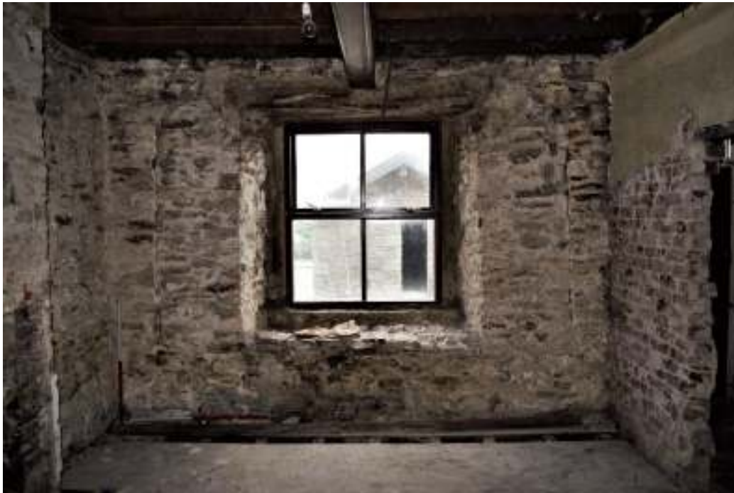
Figure 30. South east room, south elevation, window replacing two narrower openings.
