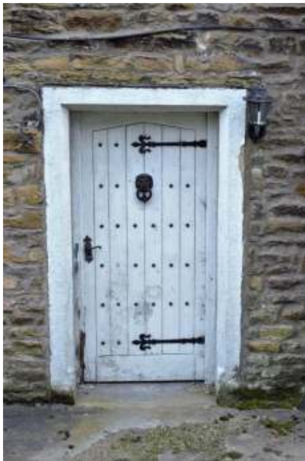
Figure 19. North elevation ground floor door.
