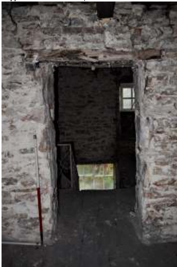
Figure 105 Upper south central room, west doorway.
