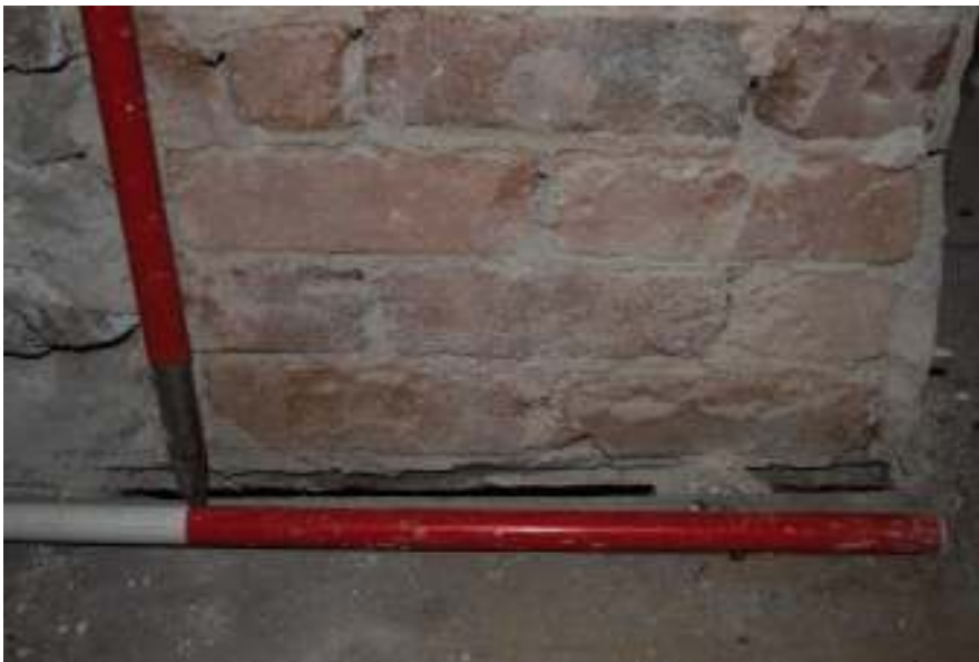
Figure 102. Base of brick corner.
