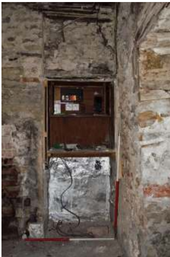
Figure 85. North west room, west wall cupboard in blocked doorway.
