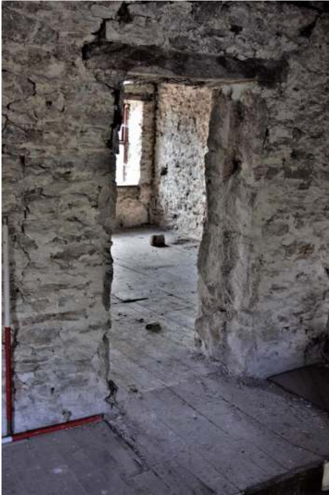
Figure 121 Original doorway between north east rooms in north and south ranges.
