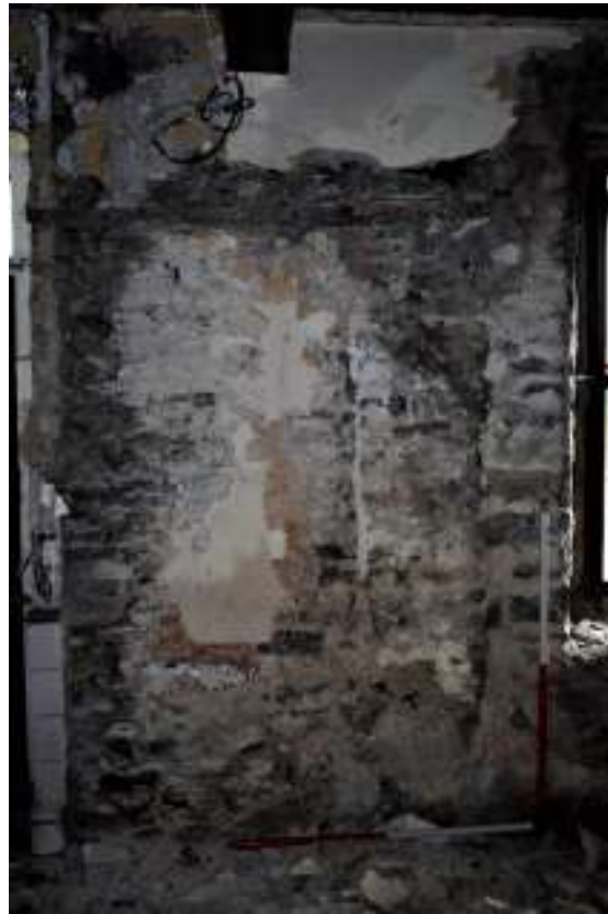
Figure 42. Central room, south elevation masonry joints.
