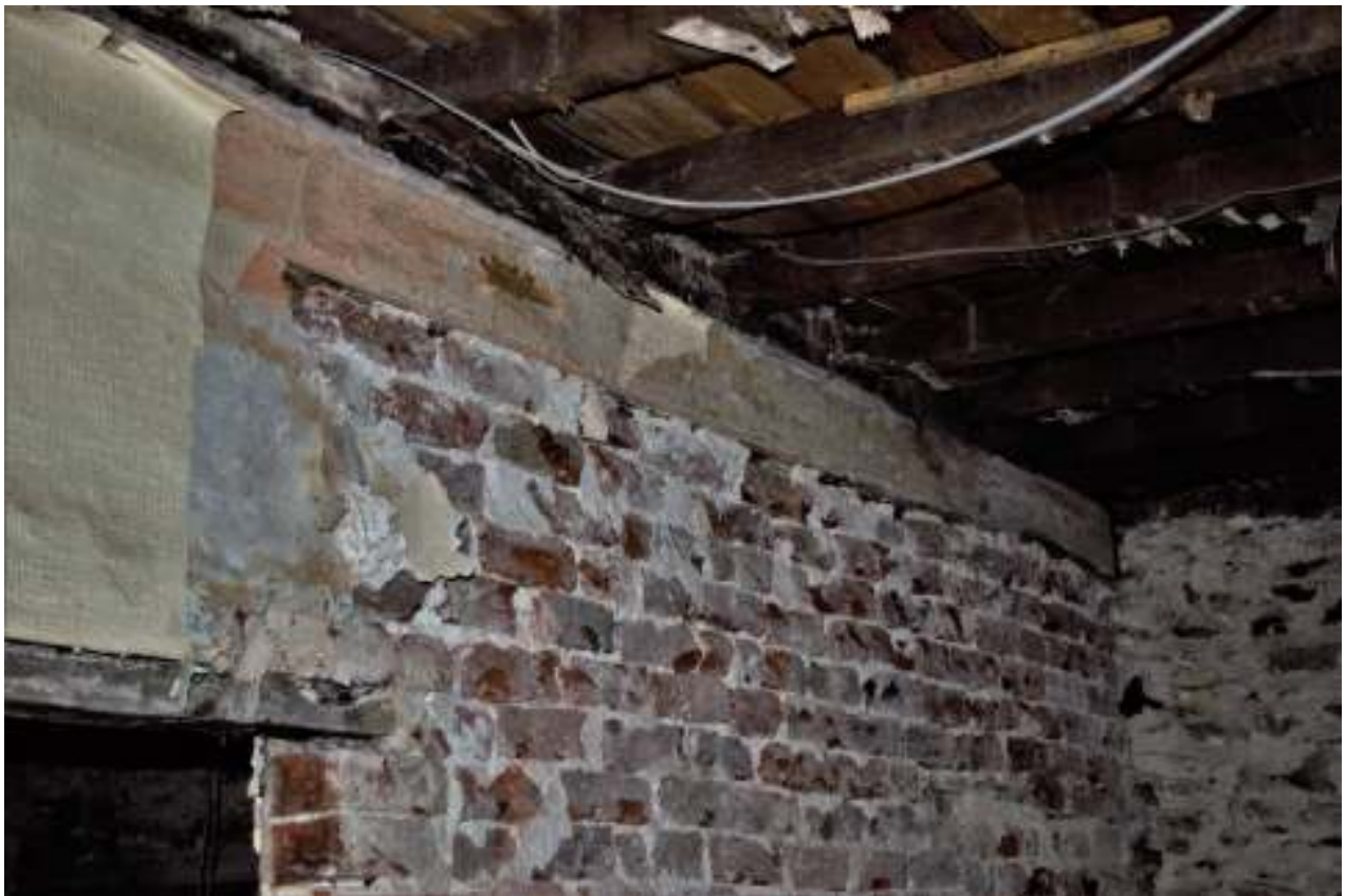
Figure 33. Door in W elevation SE room cut through inserted wall.
