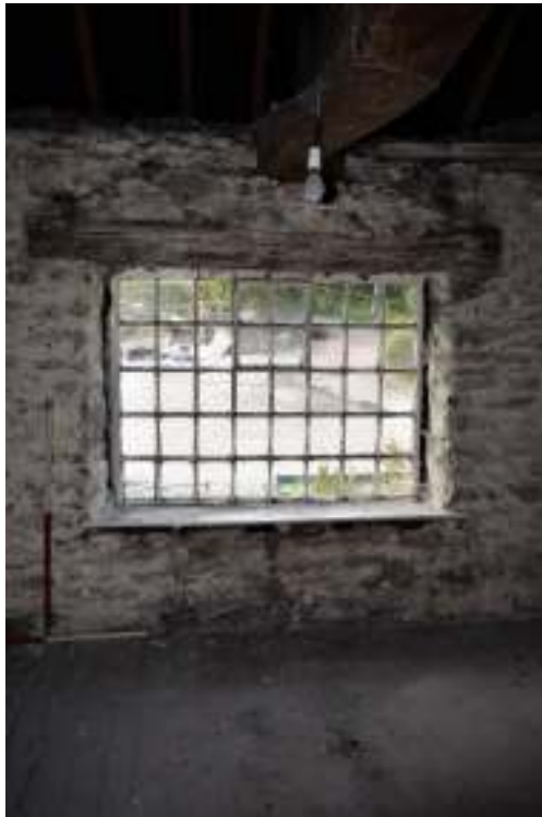
Figure 125. Upper north west room, north wall, east window.
