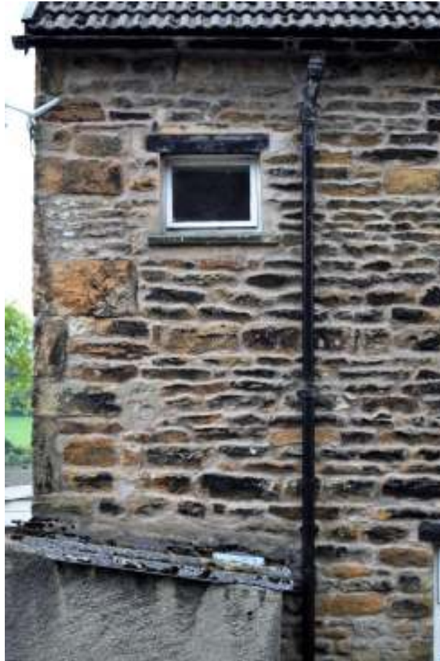
Figure 12. North elevation, eastern window to first floor NE room.
