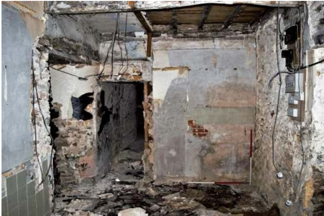
Figure 71. Northeast room, west elevation.
