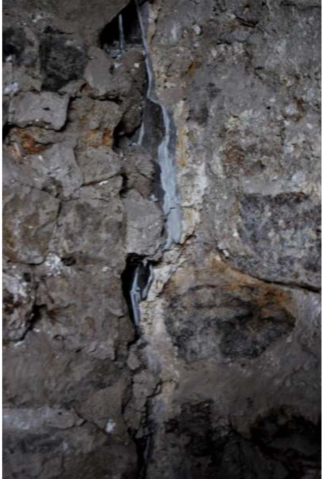
Figure 38. South east room, chimney breast butted against wall plaster.
