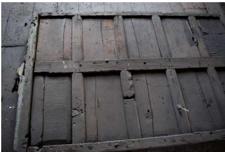
Figure 138 Section of panelling, rear face.
