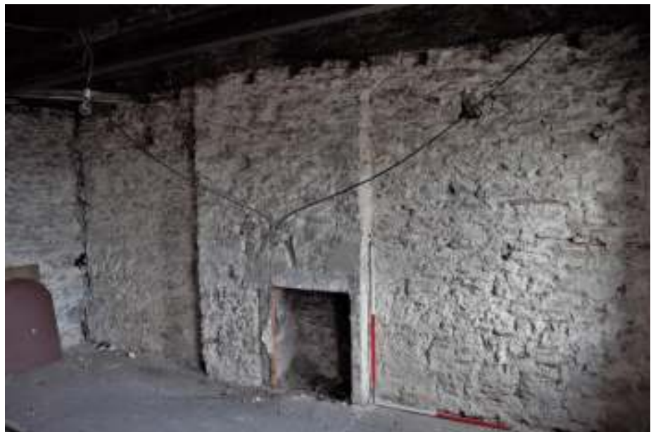
Figure 94 Upper south east room, east wall.
