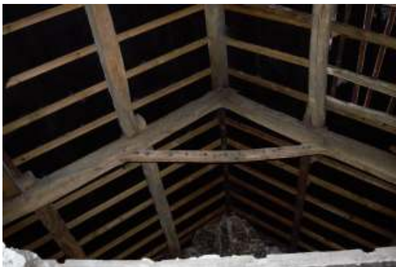
Figure 130 Eastern roof truss from west.
