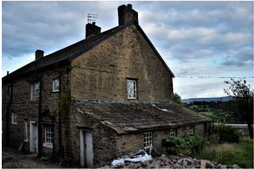
Figure 23. West gable end with lean-to.
