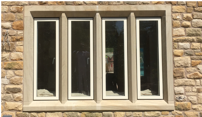
Windows/Doors Powder coated aluminium frames
