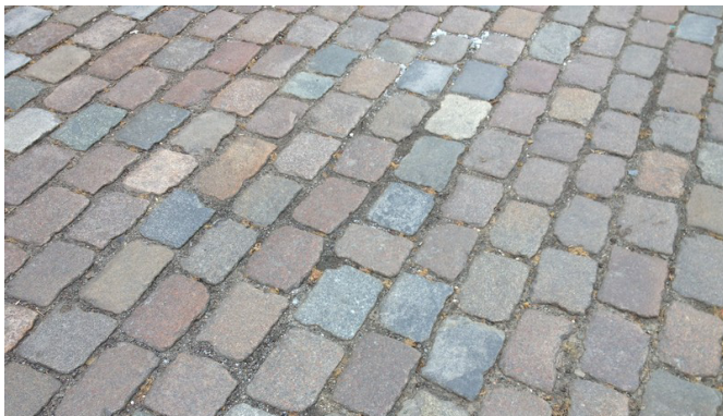
Setts/Cobbles Granite to be approx. 100x100x200mm laid to stretcher bond
