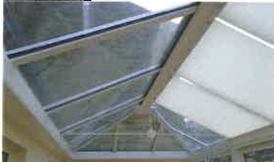
under side of conservatory roof
