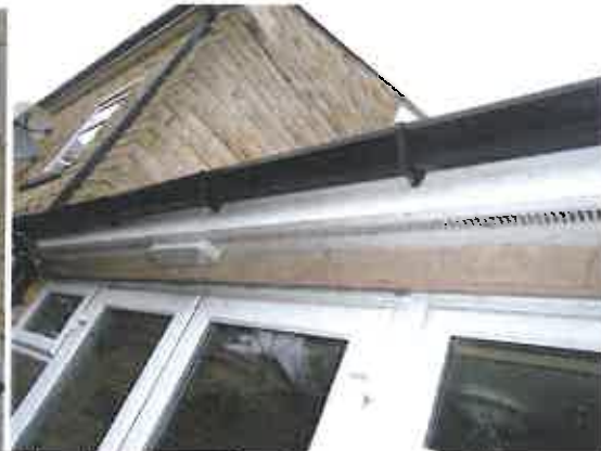
Lean to roof with slate finish, lead flashing at abutment with walls and upvc fascia with vented soffit.
