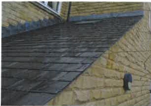
Lean to roof with slate finish, lead flashing at abutment with walls and upvc fascia with vented soffit.
