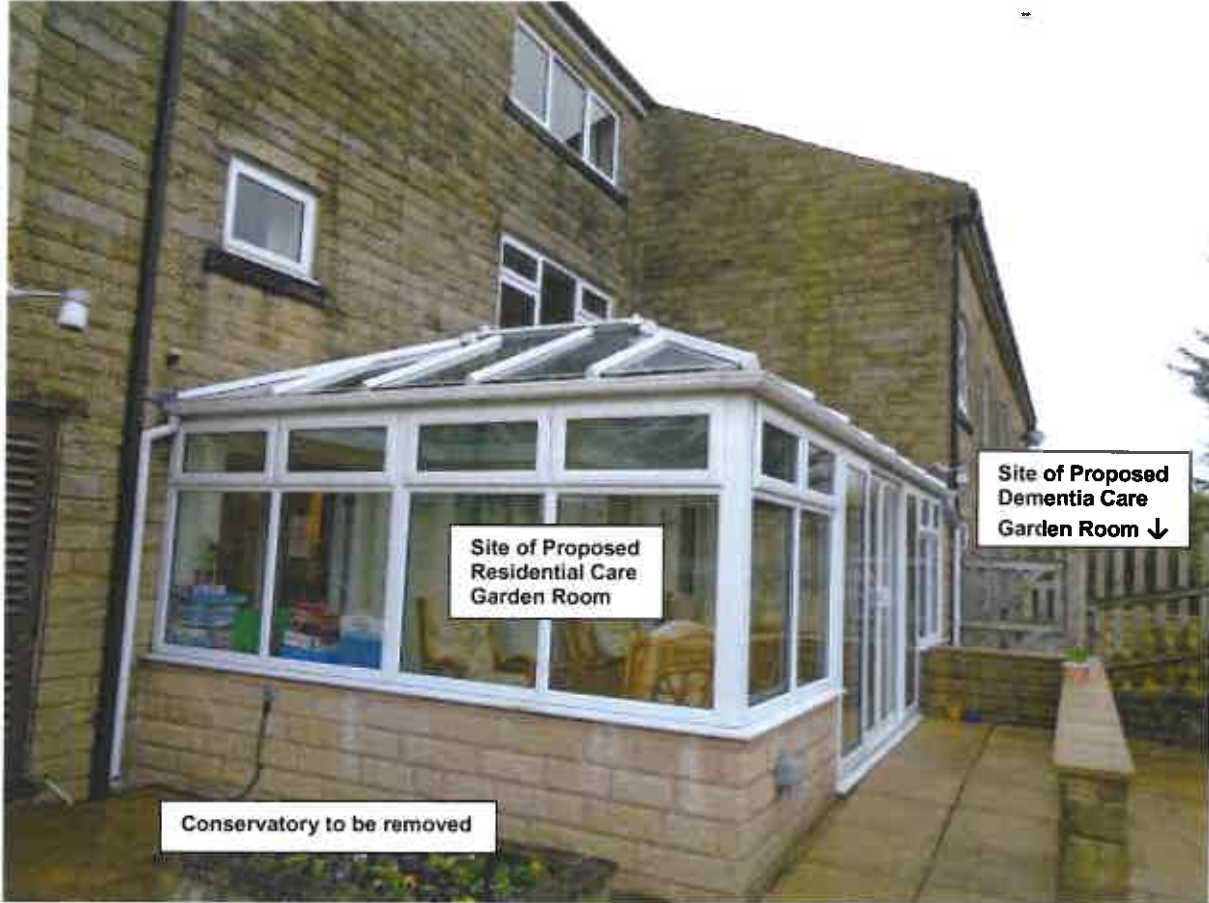
Photograph 15.1 – South west elevation
