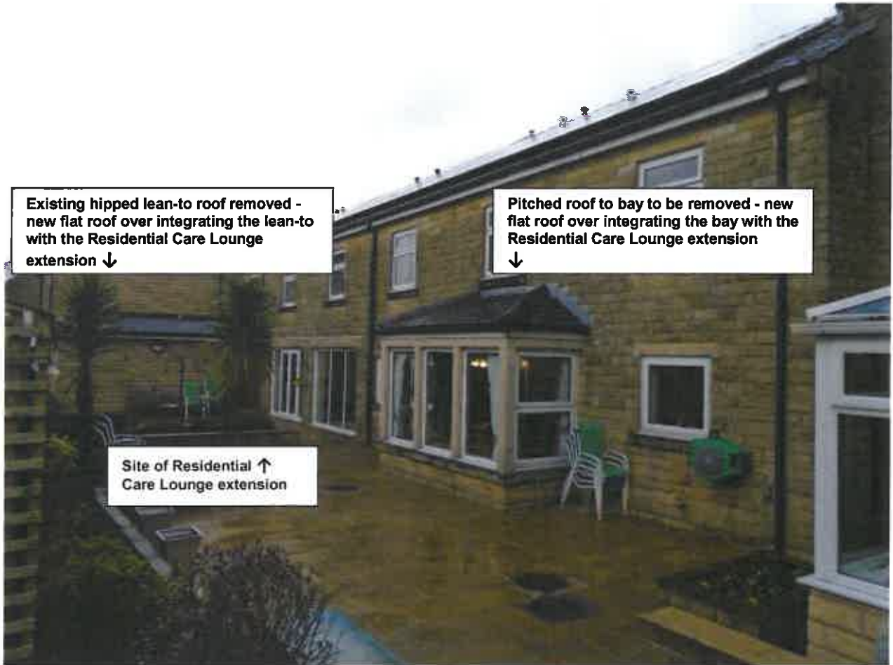
Photograph 15.2 – South west elevation
