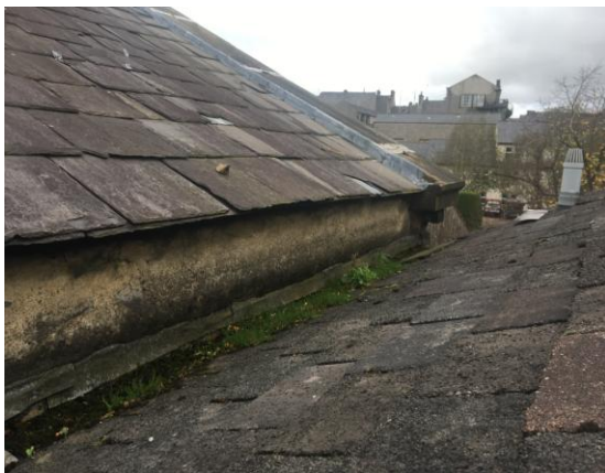
Abutment of the two pitched roofs
