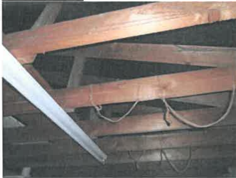
Timber truss rafter roof with underlay all in perfect condition. No enclosed roof void
