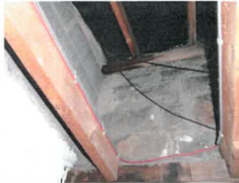
Timber truss rafter roof with underlay all in perfect condition. No enclosed roof void
