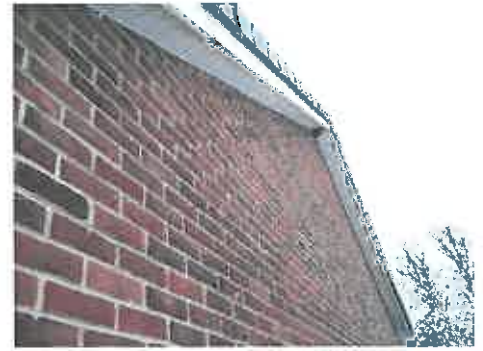
Figure 7: Side (west) elevation
