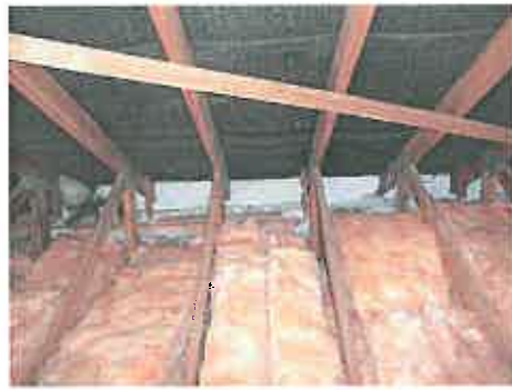
Figure 6: roof void (rear roof pitch)
