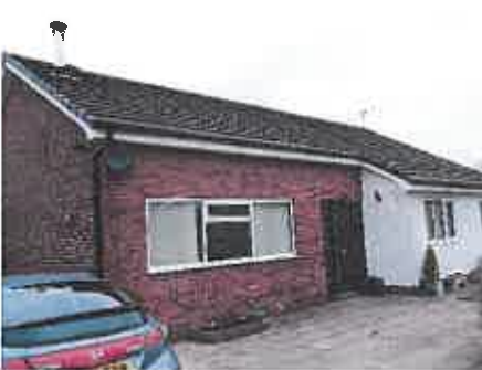
Figure 2: Front (south) elevation
