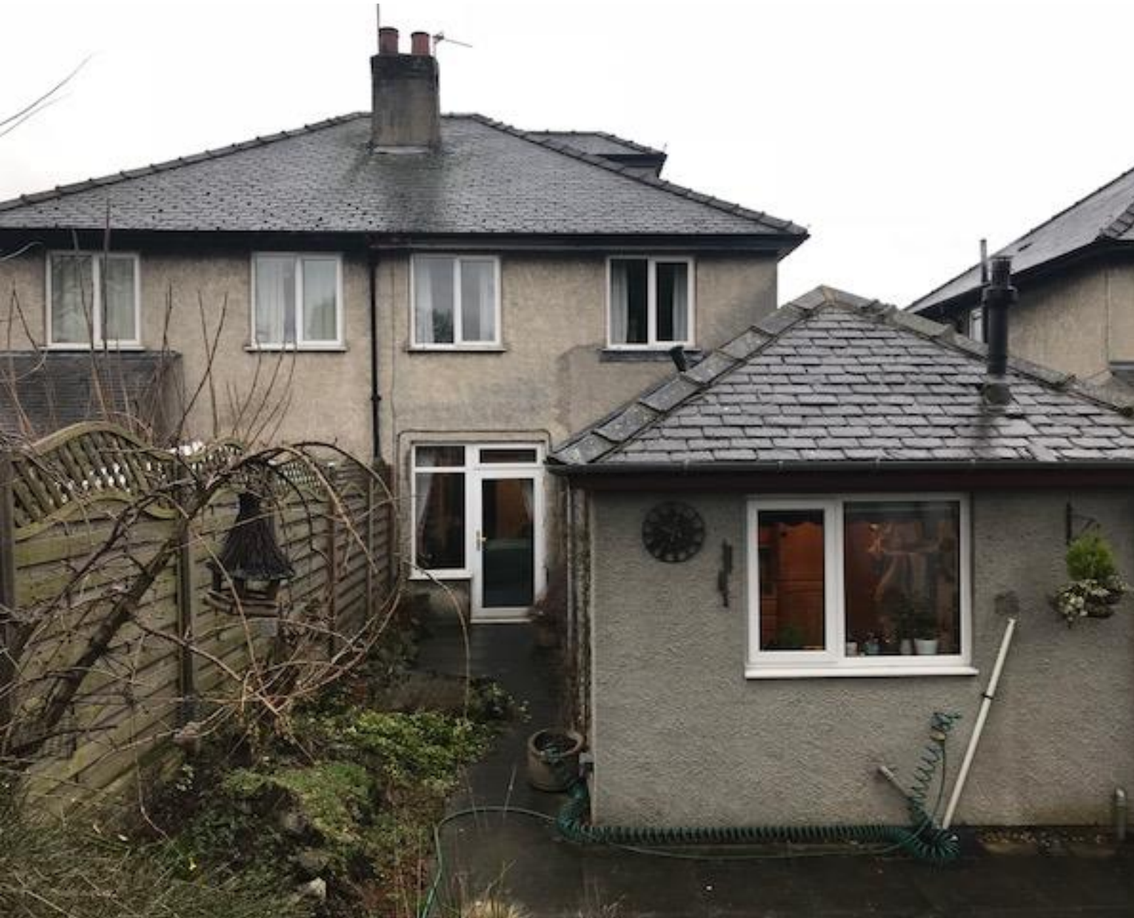
Rear view of the property showing the area of the extension
