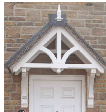
Timber door canopy & gallows brackets - tiles to match main roof (Or similar approved)
