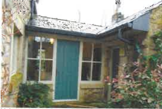
Link elevation and part outbuilding
