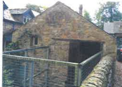
Gable of outbuilding
