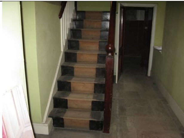
1. GF Level: Narrow stair without handrail
