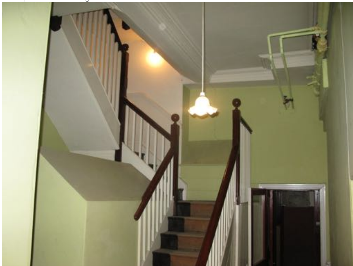
Existing staircase at ground floor level showing the convoluted route around the old brick built safe.
