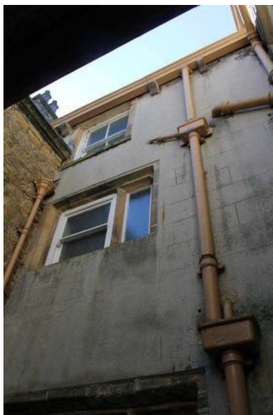
Plate 18: South wall of central yard
