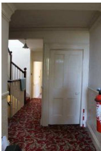
Plate 81: Four-panel timber door, with moulded margins. Upper panels larger than lower panels. Hinged to the west, with brass door knobs. Late 19th century.
