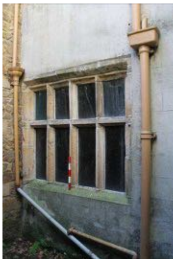
Plate 73: Eight-light cross window with stone surrounds. Mullions cut with hollow chamfers, transoms with single plain chamfers both internally and externally. The cream coloured stone is heavily weathered to the north revealing a relatively coarse texture. Thick joints and worn arrises suggest an earlier period as does the semi-regular off perpendicular tooling where it survives. Early 17th century.
