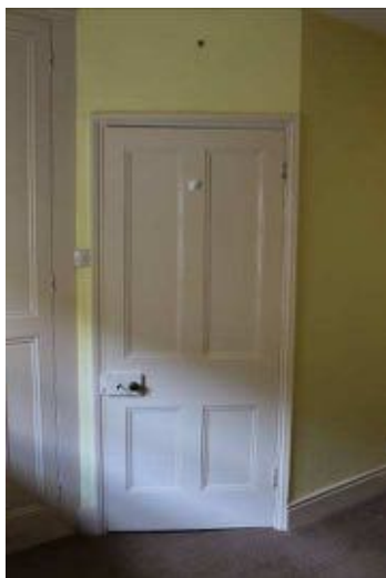
Plate 90: Four-panel timber door, with moulded margins. Upper panels larger than lower panels. Hinged to the north, with brass door knobs and locking plate on the east face. Late 19th century.
