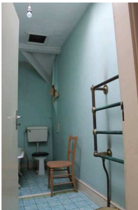
Plate 31: Room F14h , facing north
