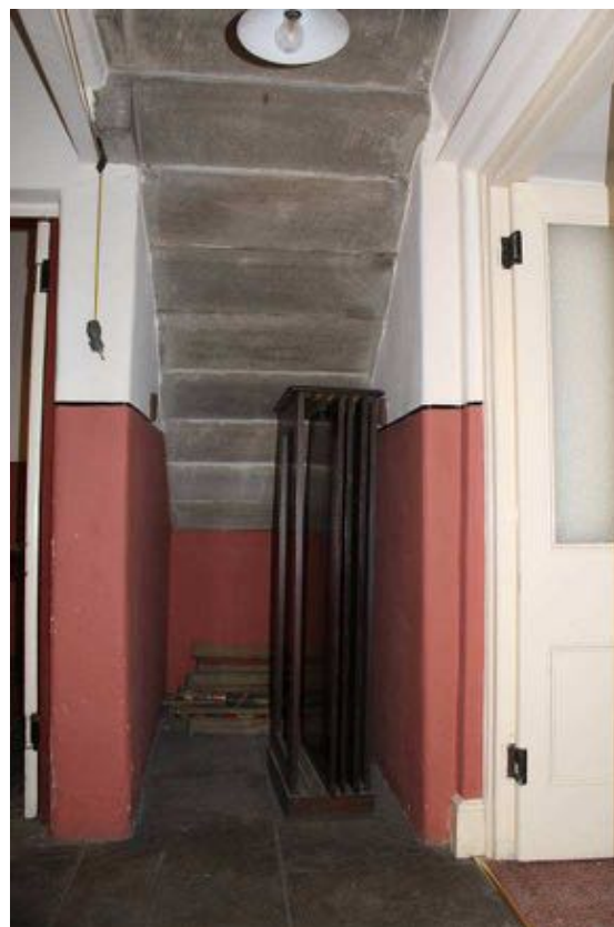
Plate 12: Room G9d, facing south
