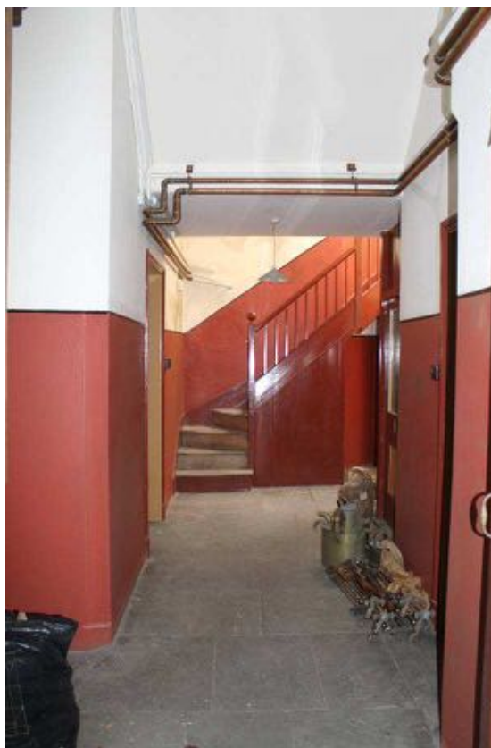
Plate 10: Room G9b facing north
