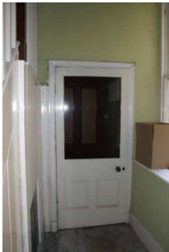
Plate 56: One large glazed panel above two small panels with moulded margins. Hinged to the west, with brass door handle. Late 19th century
