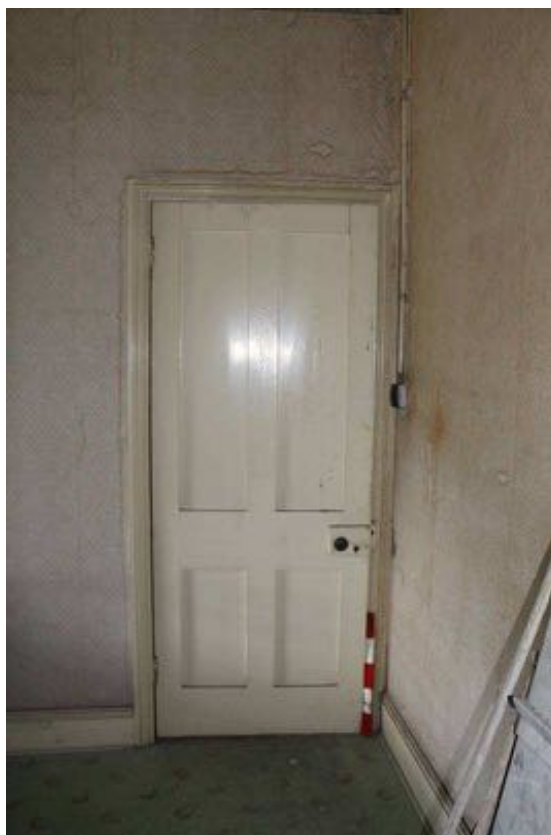
Plate 51: Room F21b, facing south, 0.5m scale
