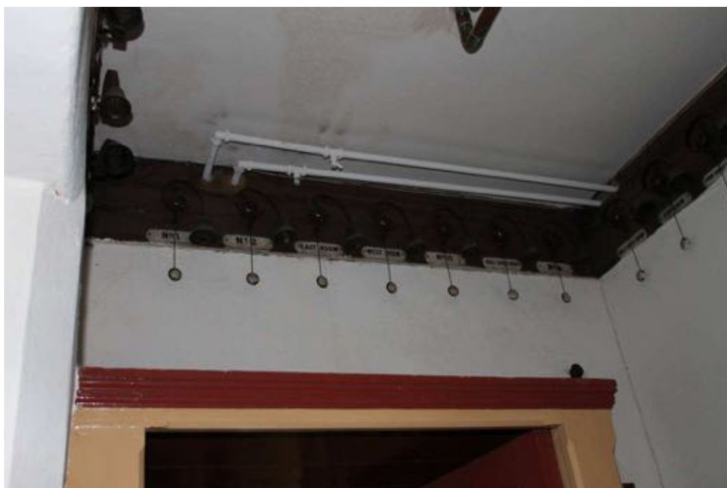
Plate 8: Servants bells at western end facing south
