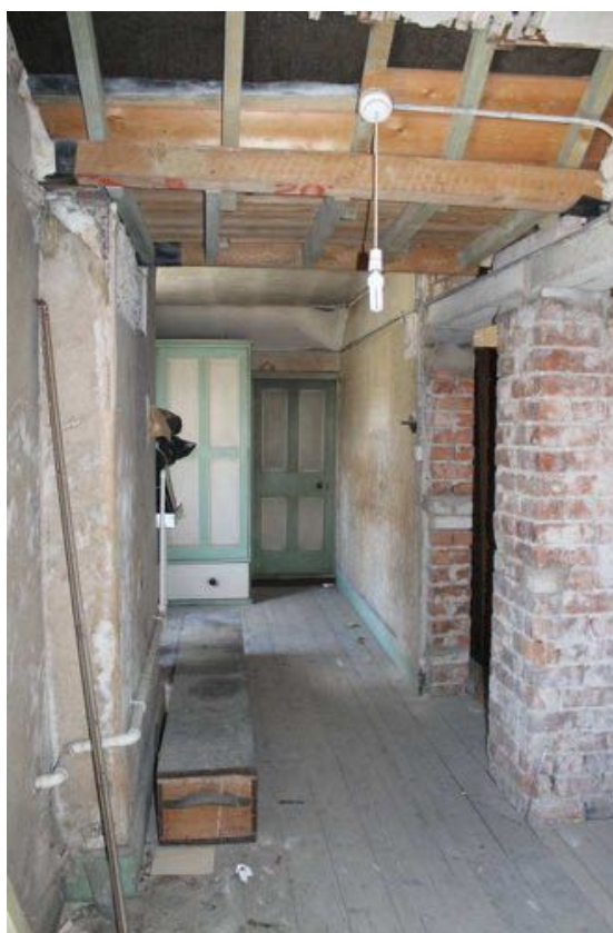
Plate 35: Corridor Room S3 , facing south
