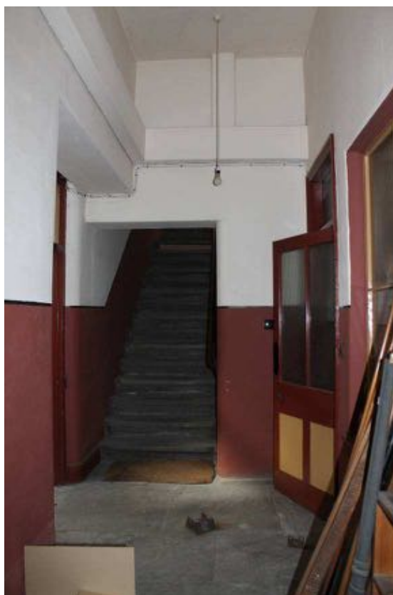
Plate 14: Room G9g , facing north
