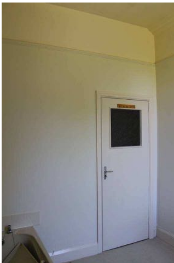
Plate 39: Room F16, facing east
