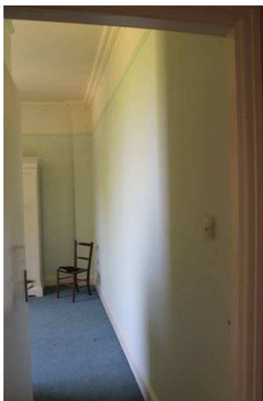
Plate 41: Room F17b, facing north
