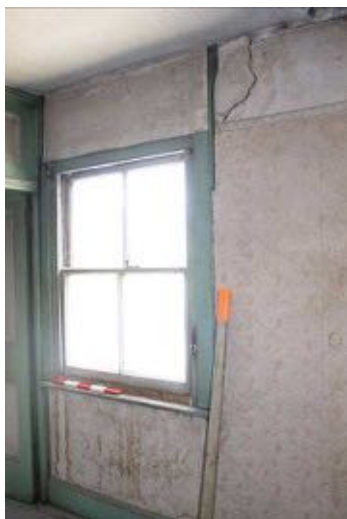
Plate 112: Two-over-two light timber sash window. Plain square section external stone surrounds, not closely inspected but appear similar to SW13. Sash fastener on interior meeting rail. Mid- late 19th century.
