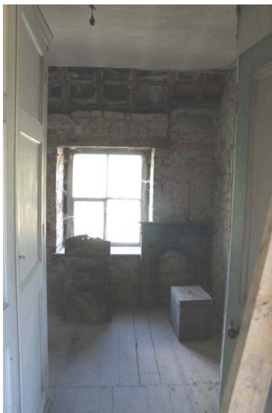
Plate 36: Room S9 , facing north
