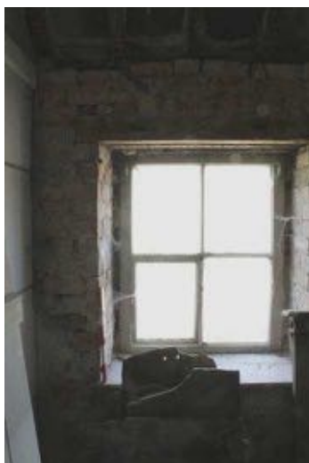
Plate 113: Faux two-over-two light timber sash window. Only the lower western light opens upon a central pivot hinge. Not observed externally. Late 19th century
