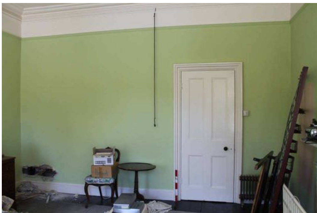
Plate 55: Western wall of Room F22b , facing west, 0.5m scale
