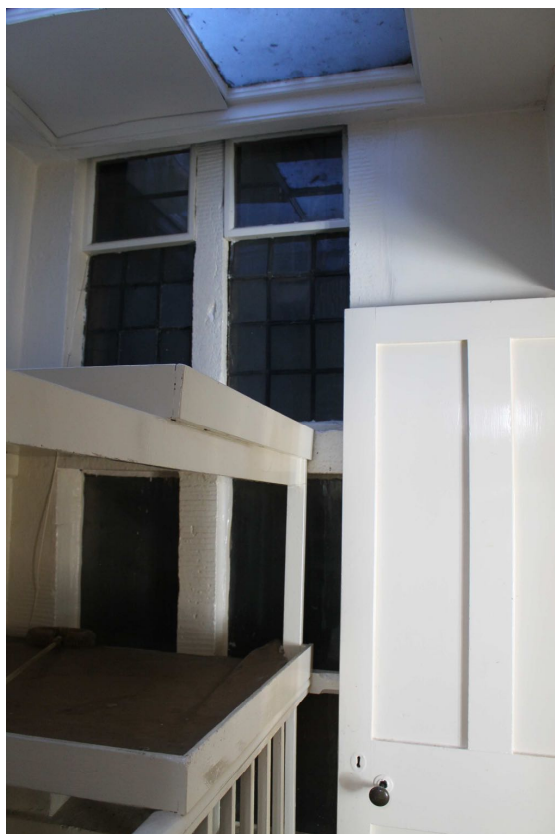
Plate 32: Mullion and transom window in Room F14i
