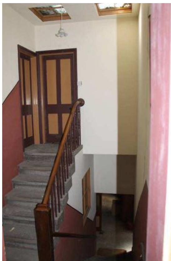
Plate 30: Stairwell Room F14g , facing south
