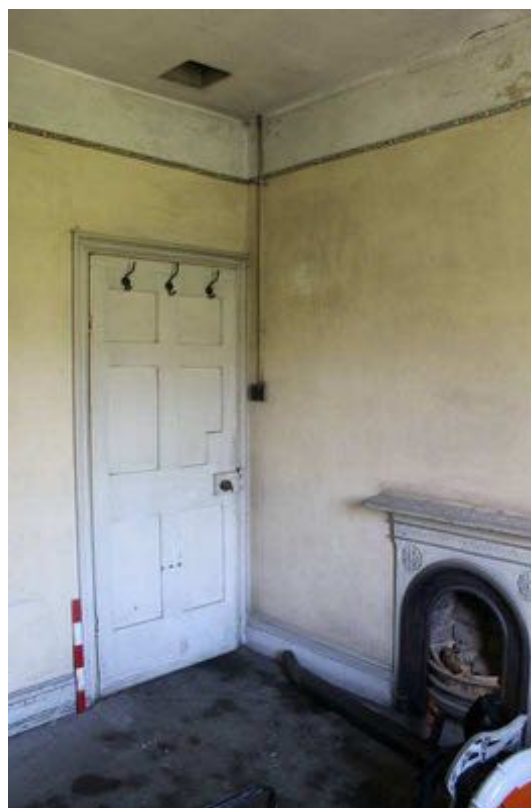
Plate 45: Room F19a , facing south-east, 0.5m scale
