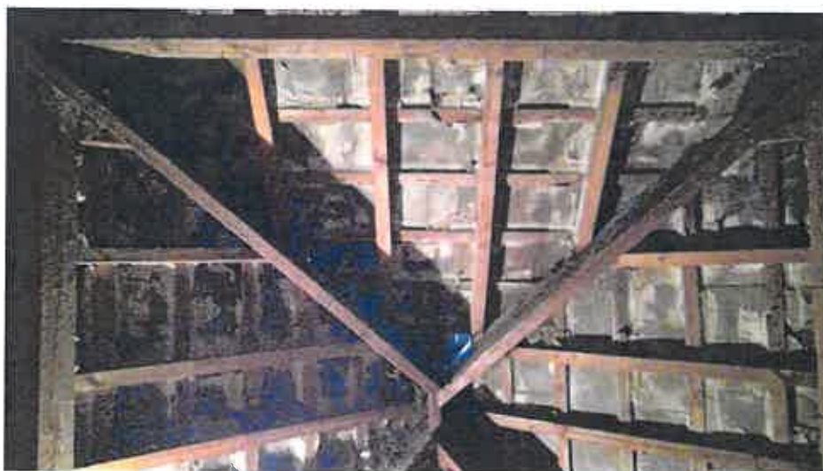
Photographs Eight: Internal apex of hipped roof, showing wooden hip rafters
