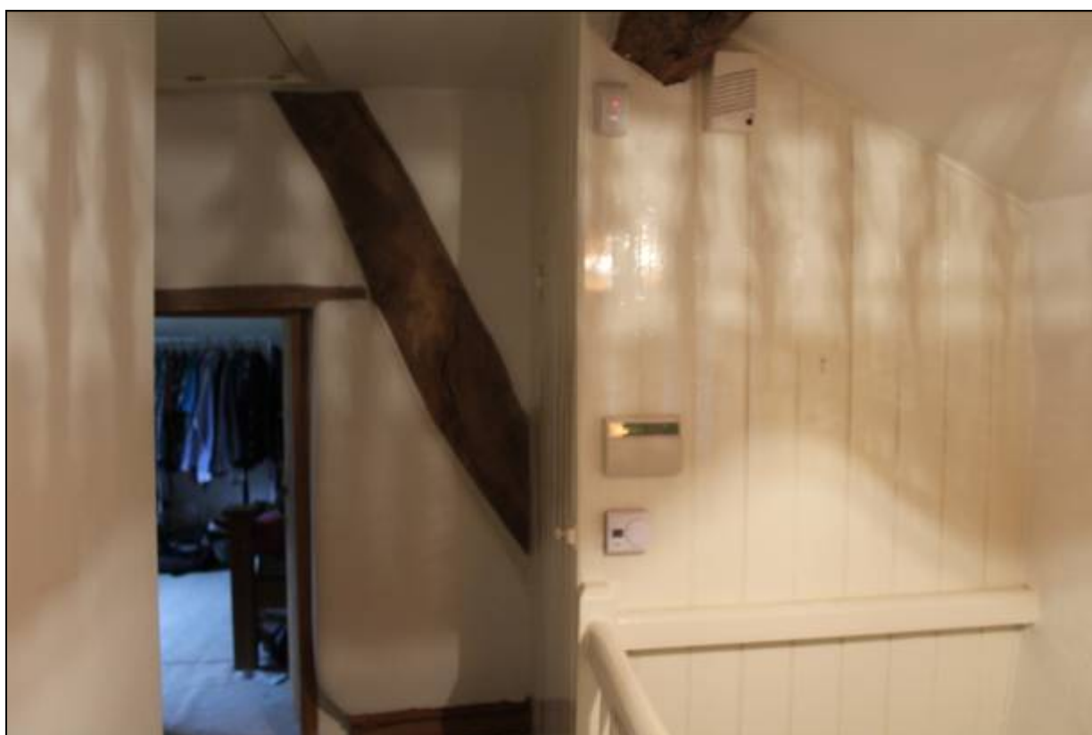
15. The northern cruck blade, viewed from stair landing
