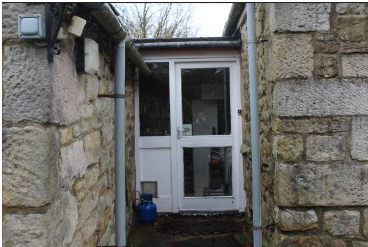
30. The flat-roofed 1970s link between former cartshed and garden room
