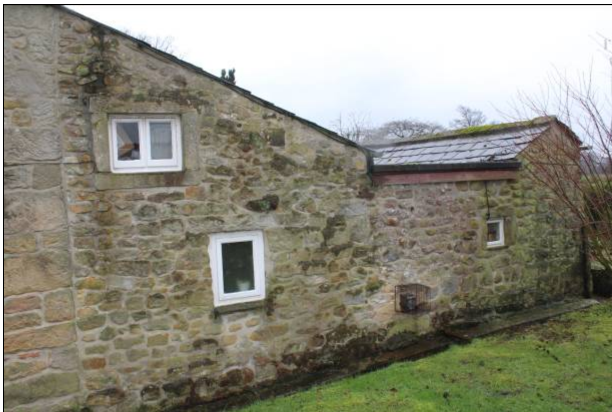
22. Rear showing junction between main range and the cartshed/garage
