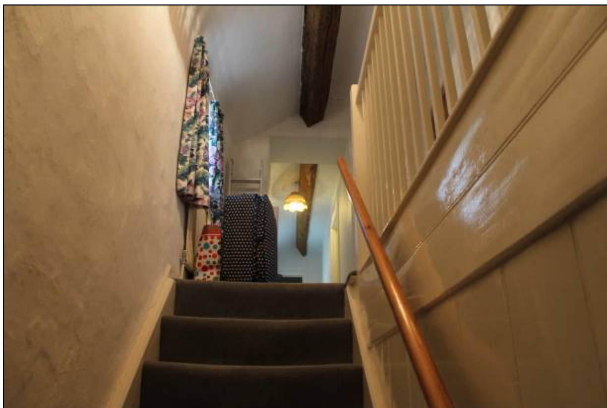
17. Staircase: its position in housebody is unlikely to be original
