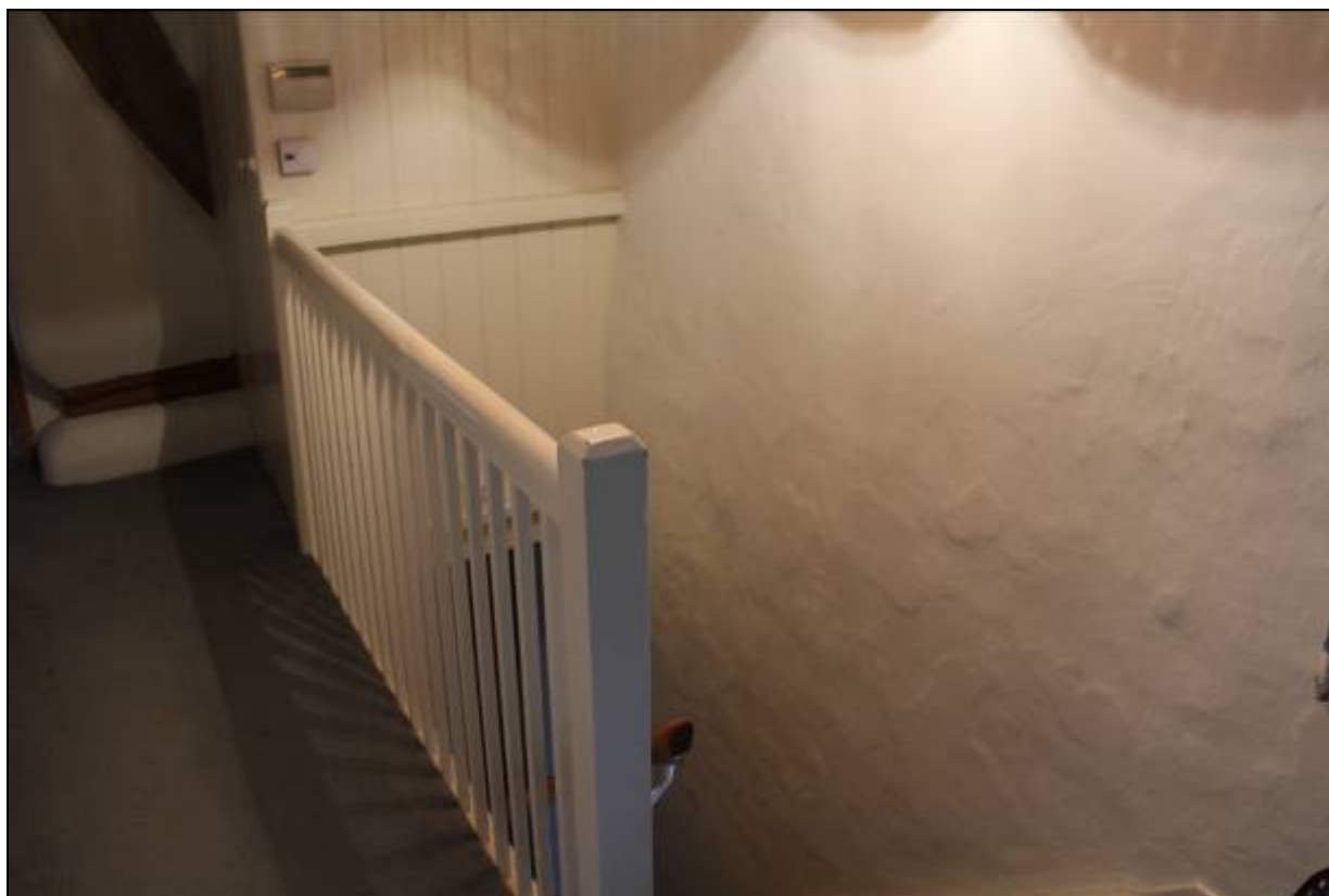
20. First floor staircase balustrade, mid-late 20 th century
