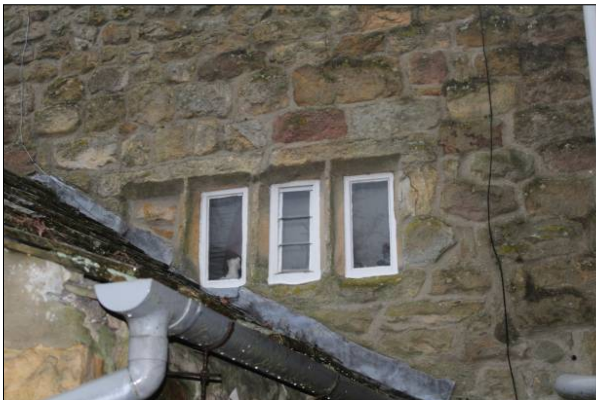
9. The 17 th century four-light window of the east gable is a crucial piece of evidence in the dating of the building
