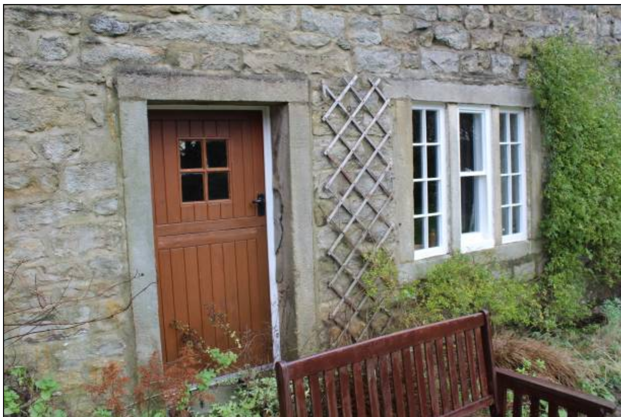
10. The plain surround of the door and windows suggests a late 18 th -early 19 th century date
