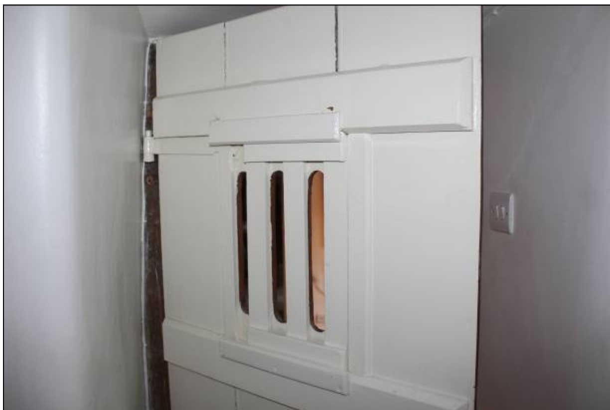
19. Door from kitchen to outbuildings with sliding panel
