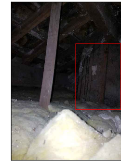
LH-2 View-3 Lime render/ plastered chimney at loft level
