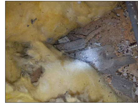
LH-1 Ceiling Lath and plaster ceiling (loft level) over Bed-2 & Bed-3
