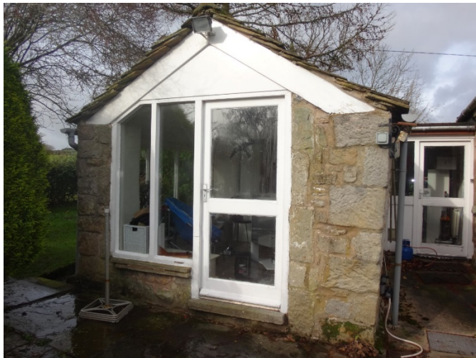
Figure 4 Large window and door inserted into outbuilding in the 70s - South Elevation
