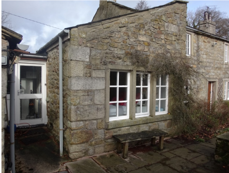
Figure 5 Existing coach house/stable door infilled with mullioned window and stone at lower level, along with flat roof link to outbuildings carried out in the 70s. The roof of the coach house appears to have been raised probably in the seventies (compare with figure 7 in the Heritage Assessment) to accommodate the flat roof link
