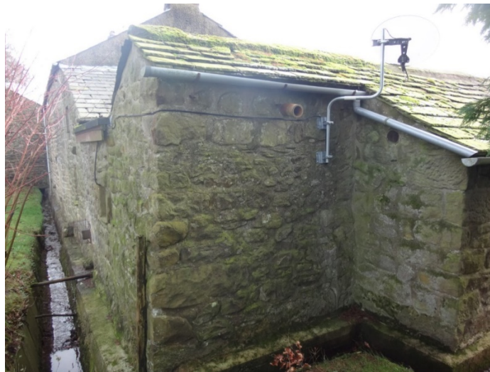
Figure 8 Original corner and recess indicating possible 'privy' linked to 'pig sty' forming the original untouched part of the outbuildings to the West. Also noteworthy is the Moat which runs around the North and West of the buildings
