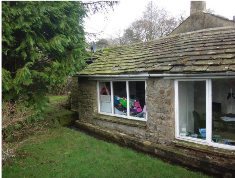
Figure 3 Large windows inserted in outbuildings to west of property in the 70s
